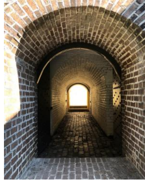
One of Fort Moultrie's many ground level entrances
