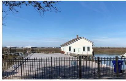
The Quartermaster's Dock, a support facility, was fully restored in 2015 by private owners.
