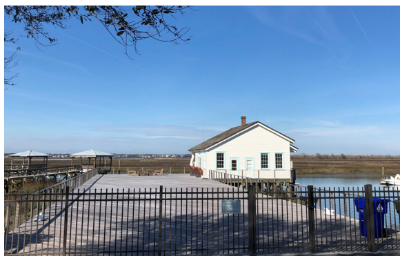
The Quartermaster's Dock, a support facility, was fully restored in 2015 by private owners.
