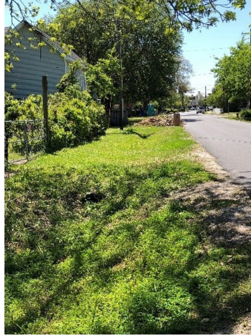
Open ditches: Unmaintained ditches can obstruct water flow and overall functionality of the storm drainage system.
