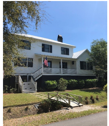
New construction is required to be elevated over the flood elevation.
