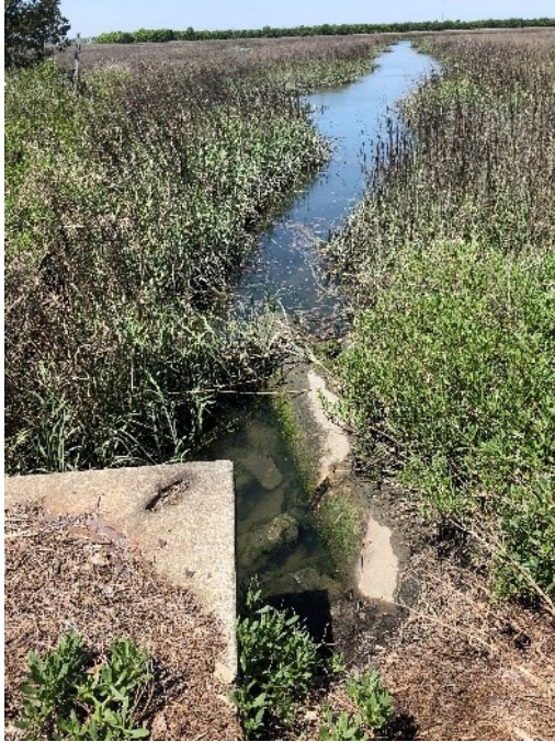
Stormwater outfalls: A damaged and cracked pipe on the right is located well below the water level creating problems with drainage.
