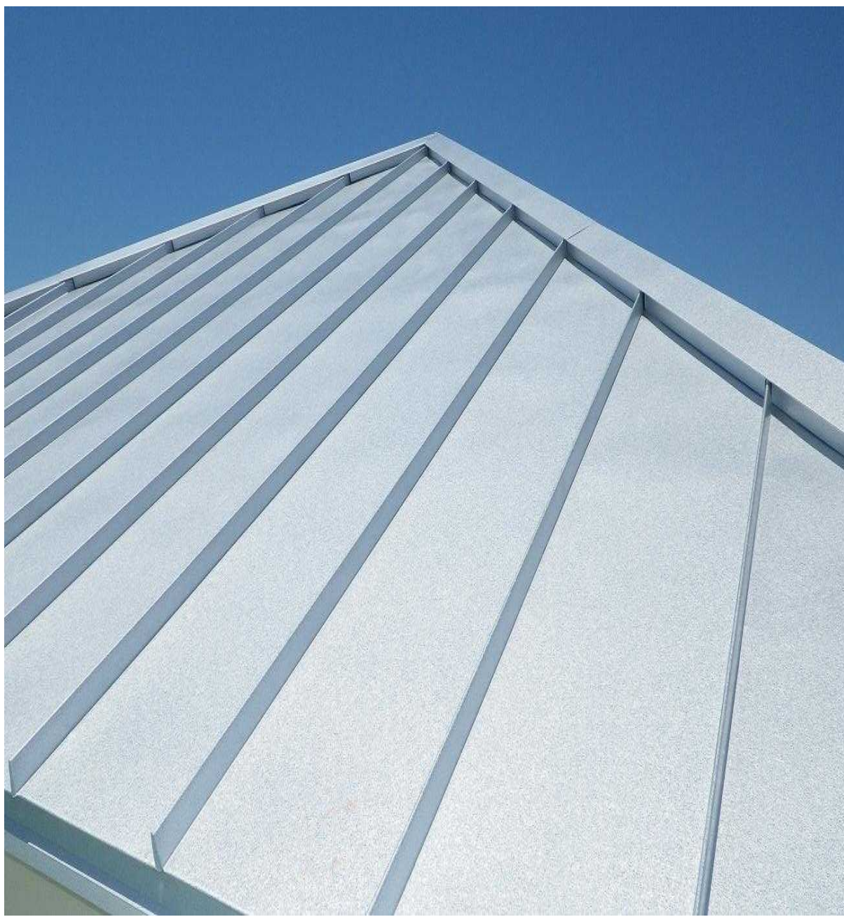
24 GAUGE MECHANICALLY SEAMED METAL ROOF
