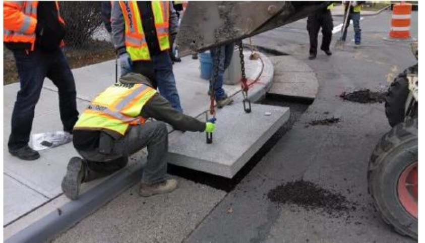
Pre-cast Stormcrete can be placed to make a porous gutter.
