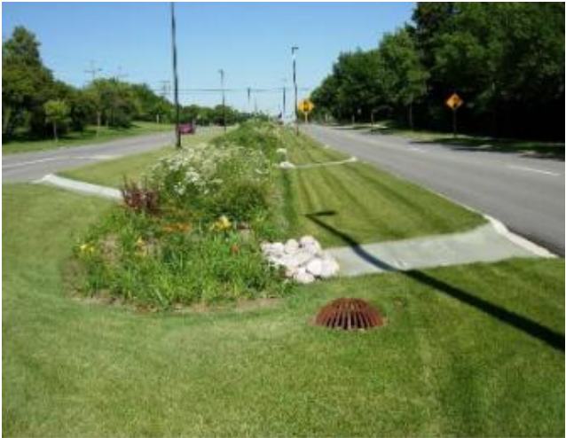
Bioswale installation in Mt. Pleasant
