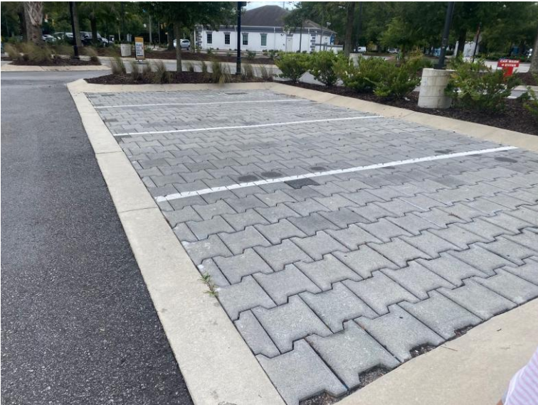
Materials vary such as this Powerblock System
