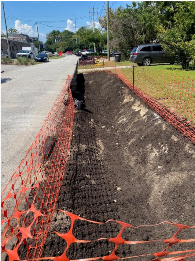
Bioswale installation in Mt. Pleasant
