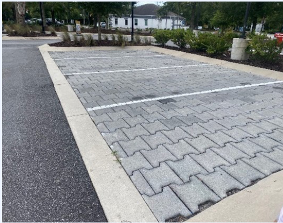
Figure 56: Interlocking permeable paver system that does not require aggregate between pavers, James Island, SC.
