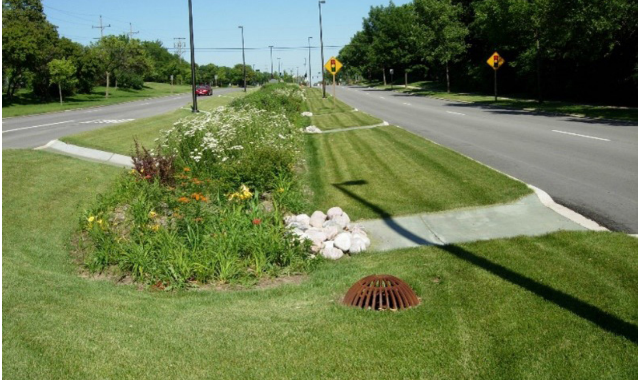
Figure 90: Example of median bioswale. Image Source: McCormick Taylor.
