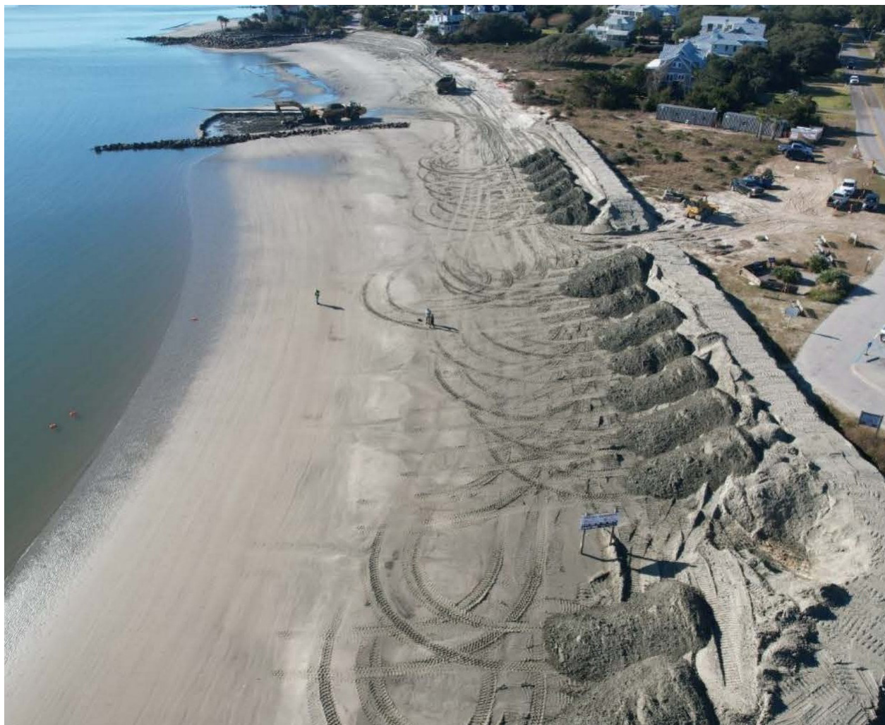
Figure 73: Town contractor moving sand from USACE Beneficial Use of Dredged Material (BUDM) project along the Sullivan's Island Breach Inlet shoreline in late 2024. (Image Source Coastal Science & Engineering).
