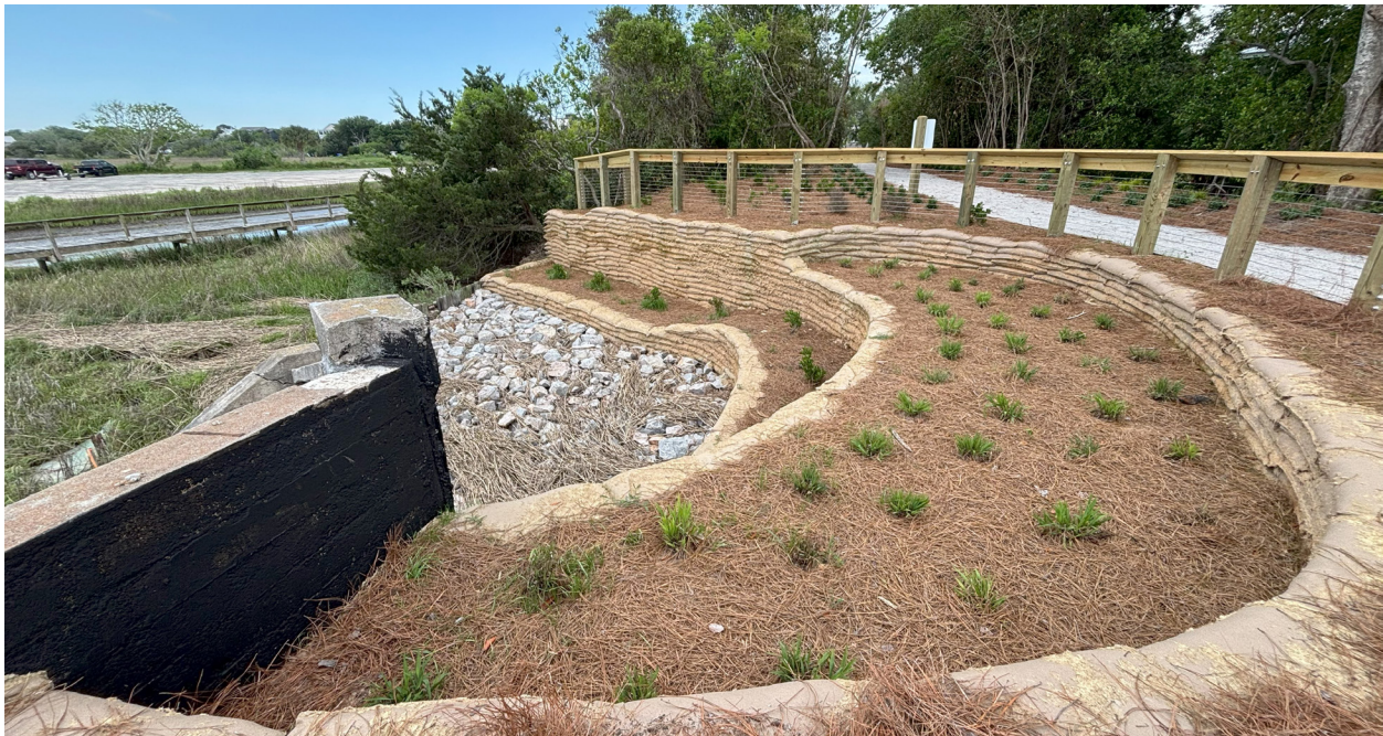
Figure 67: Envirolok on Sullivan's Island. Source: Elko Coastal Consulting.
