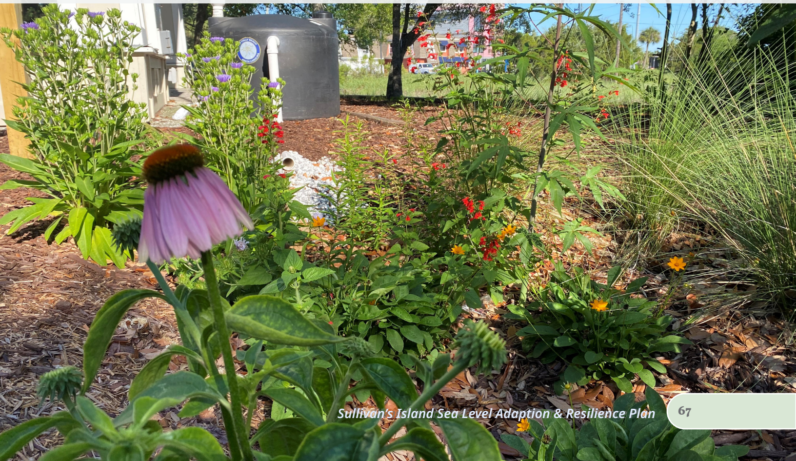
Figure 37: A rain garden and rainwater harvesting system located at the Folly River Park work together to manage stormwater
