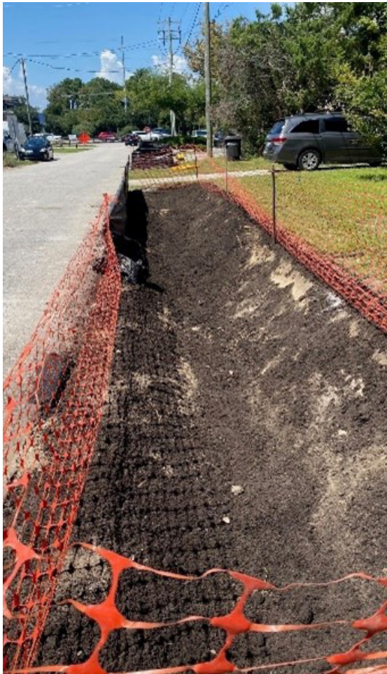
Figure 58: Bioswale installation using a product called “Bold & Gold” filtration media to assist with pollutant removal, Mount Pleasant, SC.
