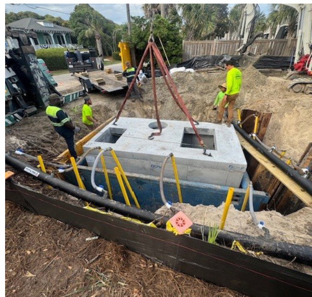
Figure 80: Installation of the innovative Dune Infiltration System on Folly Beach, June 2025. Image Source: Elko Coastal Consulting.
