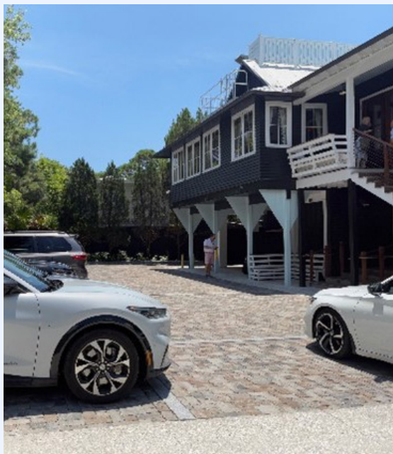
Figure 54: Existing permeable parking at Obstinate Daughter
