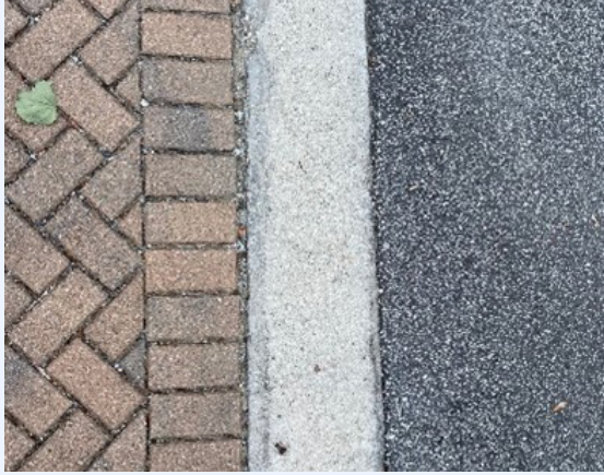
Figure 55: Concrete ribbon separates a permeable parking area from travel lanes, Mount Pleasant, SC.
