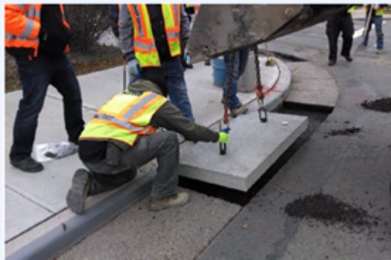
Figure 57: Stormcrete, a pre-cast pervious concrete system, is placed along road gutters in New York City, NY.
