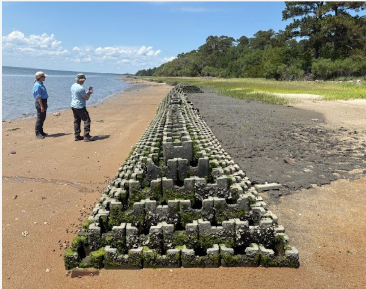
Figure 42: A recently installed living shoreline uses oyster castles to attract oyster growth, capture sediment, and support aquatic life. Beaufort, SC.
