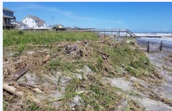
Figure 45: Photo of sand fencing and walkover materials that were destroyed during the passage of Hurricane Irma, increasing the post-storm clean-up effort (2017 Folly Beach).
