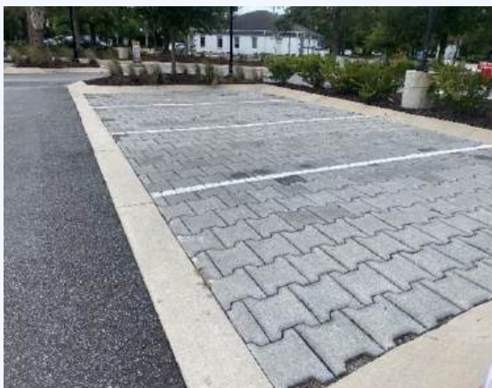
Figure 25: Interlocking permeable paver system that does not require aggregate between pavers, James Island, SC.
