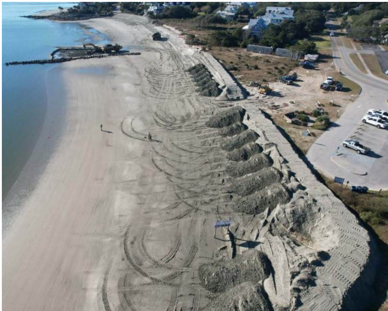
Figure 43: Town contractor moving sand from USACE Beneficial Use of Dredged Material (BUDM) project along the Sullivan's Island Breach Inlet shoreline in late 2024. Photo by CSE.
