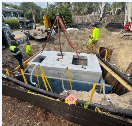
Figure 51: Installation of the innovative Dune Infiltration System on Folly Beach, June 2025.
