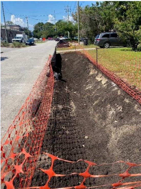
Figure 27: Bioswale installation using a product called "Bold & Gold" filtration media to assist with pollutant removal, Mount Pleasant, SC.
