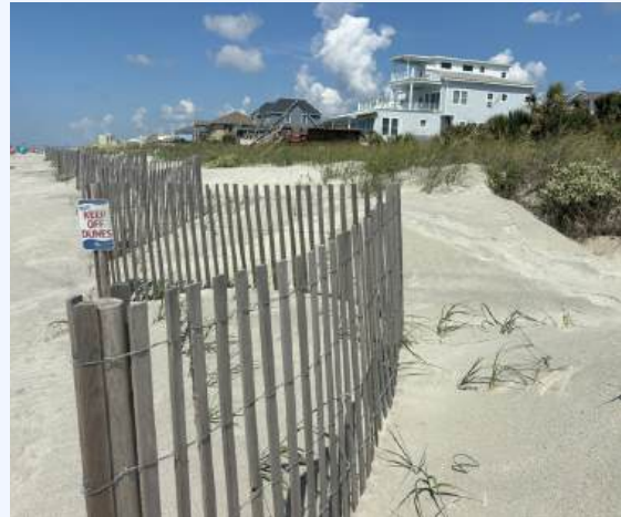
Figure 49: Example of using sand fencing and vegetation to restore dune system on Folly Beach.
