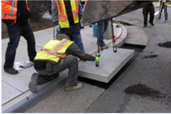
Figure 26: Stormcrete, a pre-cast pervious concrete system, is placed along road gutters in New York City, NY.
