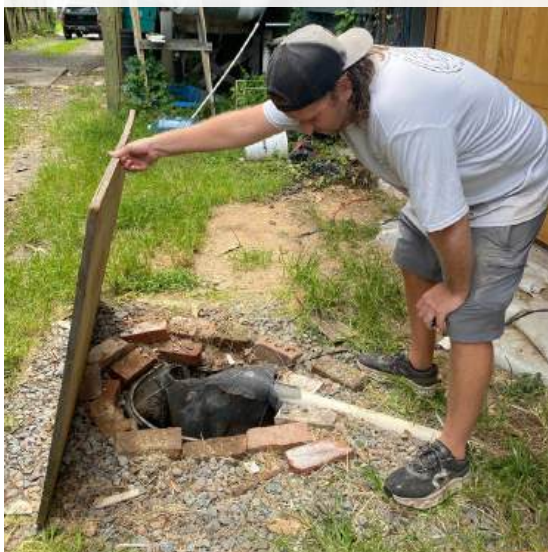
Figure 5: A local business owner showcases a sump pump used during high water events to reduce flooding in his place of business along Middle Street
