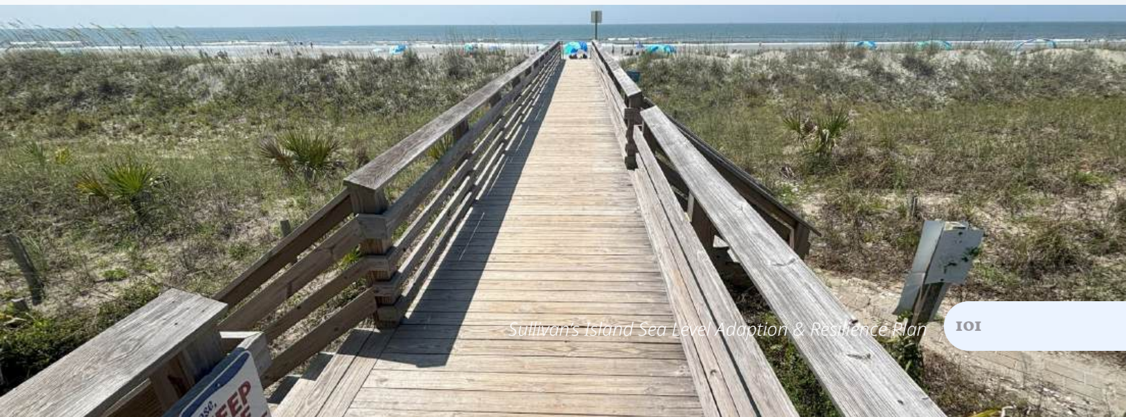
Figure 47: Example of offshoots of public dune walkover into secondary dune path to discourage use of numerous private footpaths through the dunes (Folly Beach 6th St. W.).
