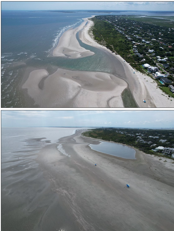
FIGURE 3.12. Aerial imagery between August 2023 (upper) and September 2024 (lower) reflects the attachment of a shoal released via ‘bypass’ from Breach Inlet. As the shoal attached to Sullivan’s Island near CSE station 142+50 (Sta 28 ½), its crest elevation increased, and the onshore migration rate slowed. As a result, a ‘cat-eye’ pond was formed near the attachment zone.
