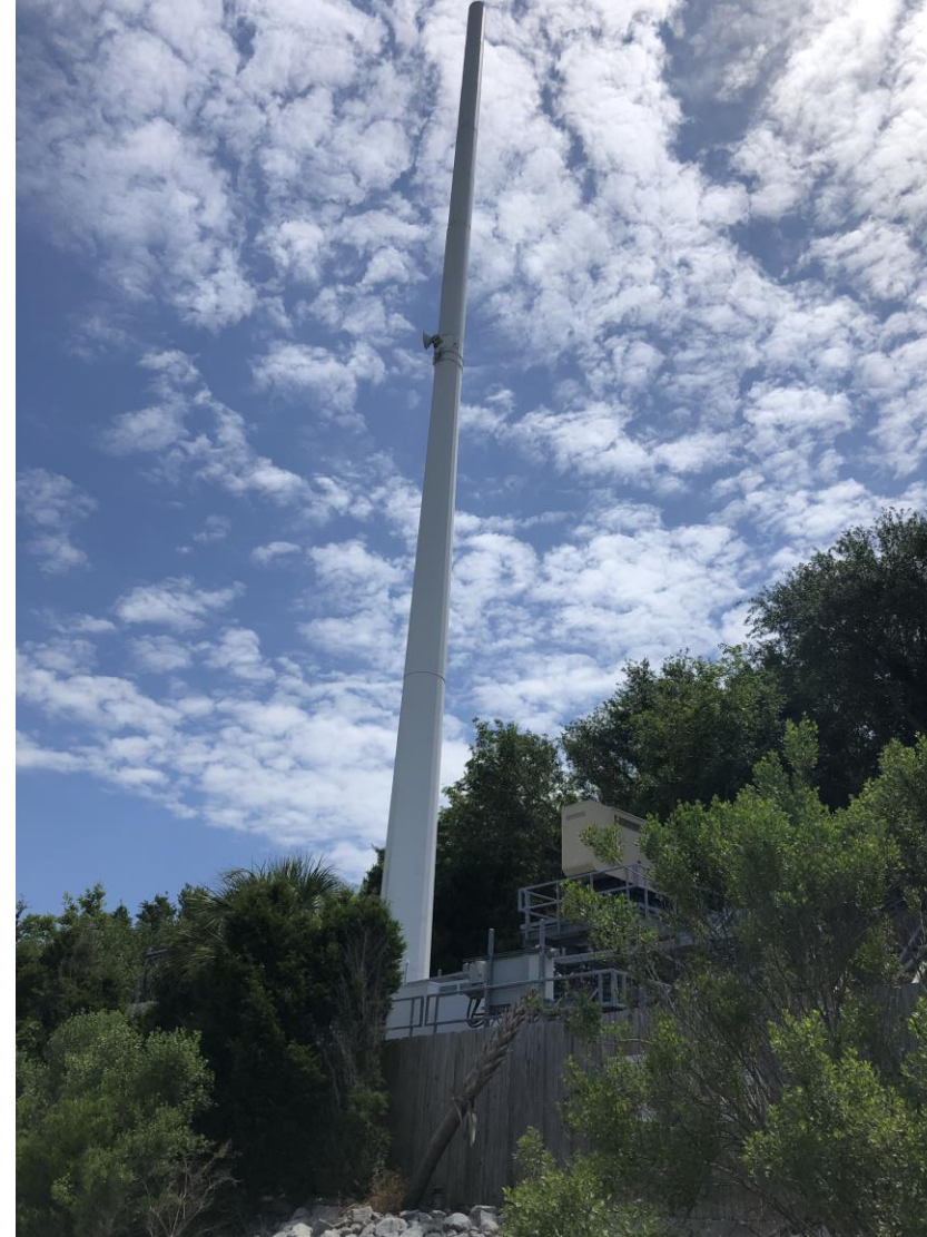
Stealth Monopole Tower
