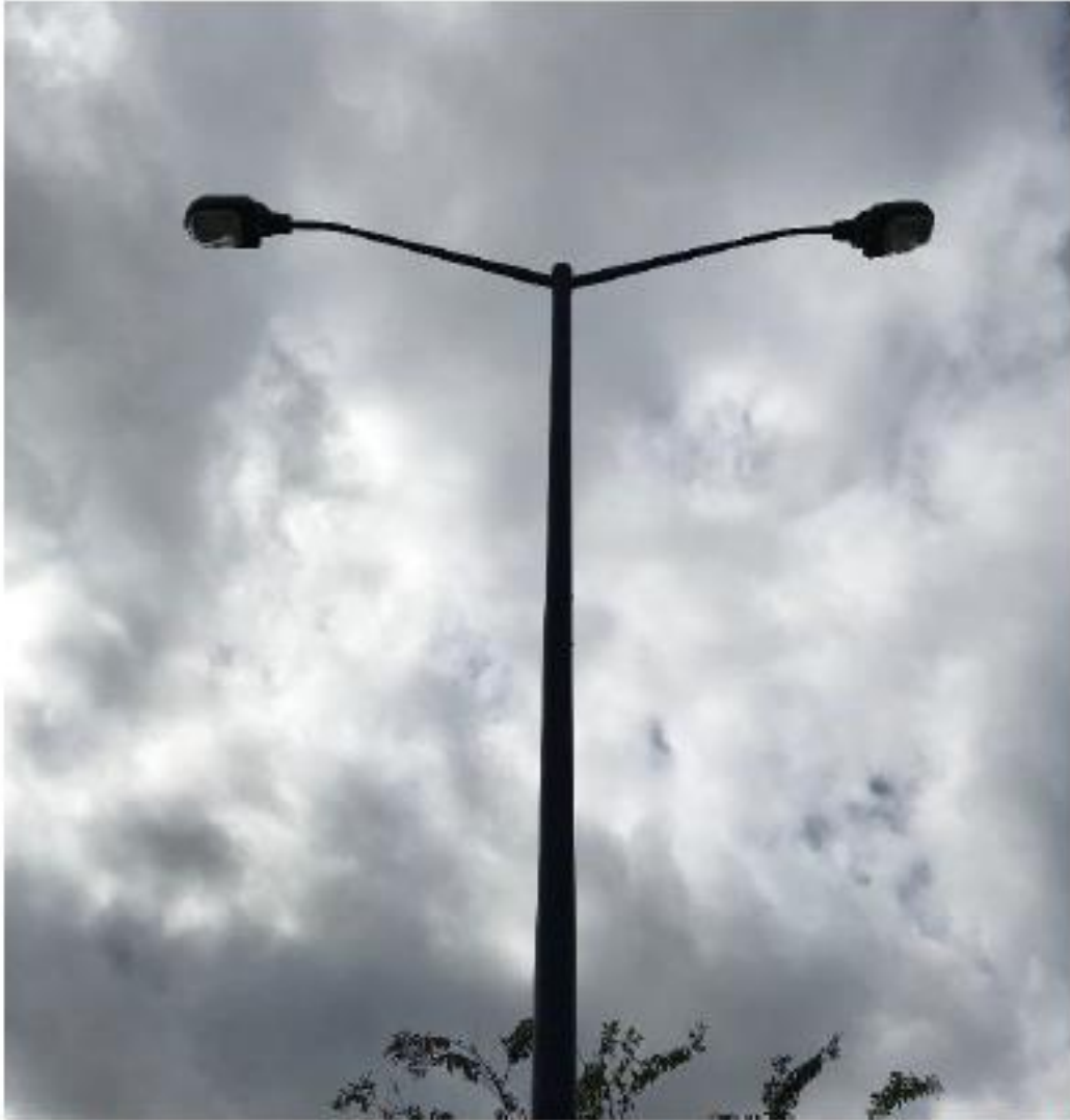
Existing “cobra” pole on Johnnie Dodds Blvd
