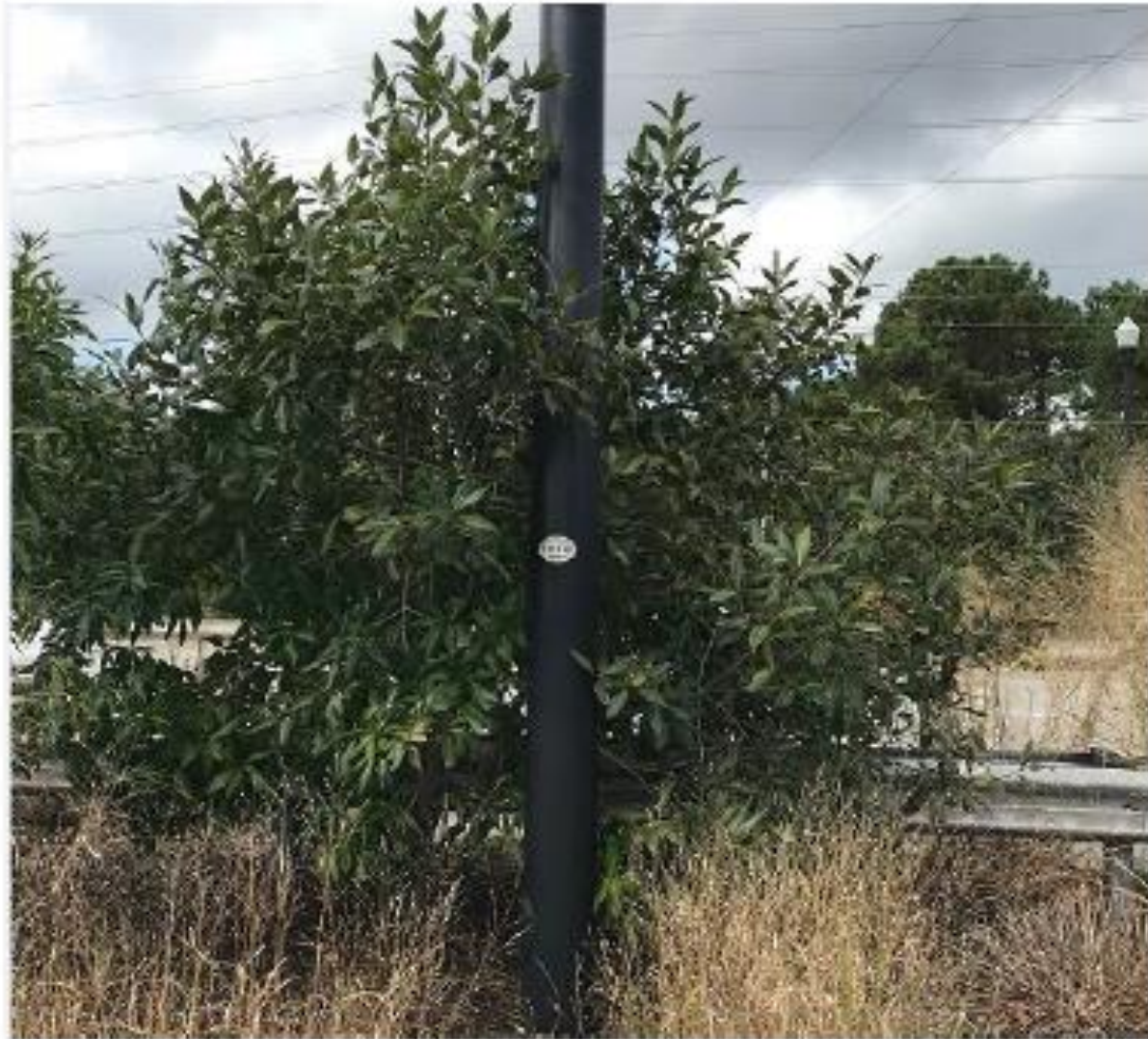
Existing bottom of pole on Johnnie Dodds
