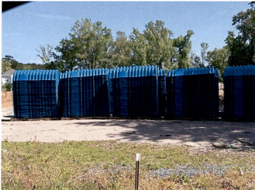
Examples of underground detention chambers about to be installed on Johns Island, SC.
