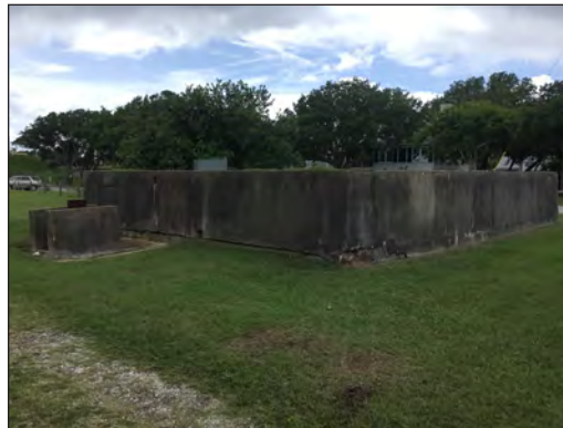
D. Circa 1898 Battery Jasper Reservoir No. 1, SHPO Site Number 1036.01
