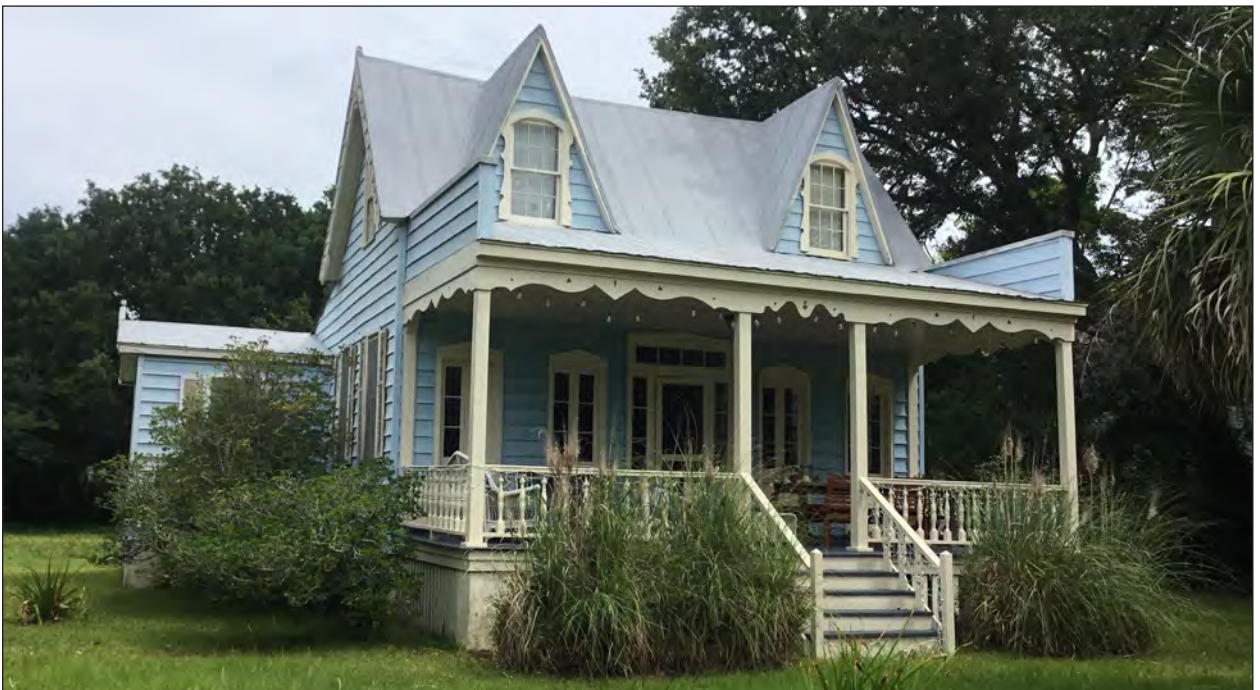
B. McGoldrick House at 2002 Middle Street, SHPO Site Number 0922
