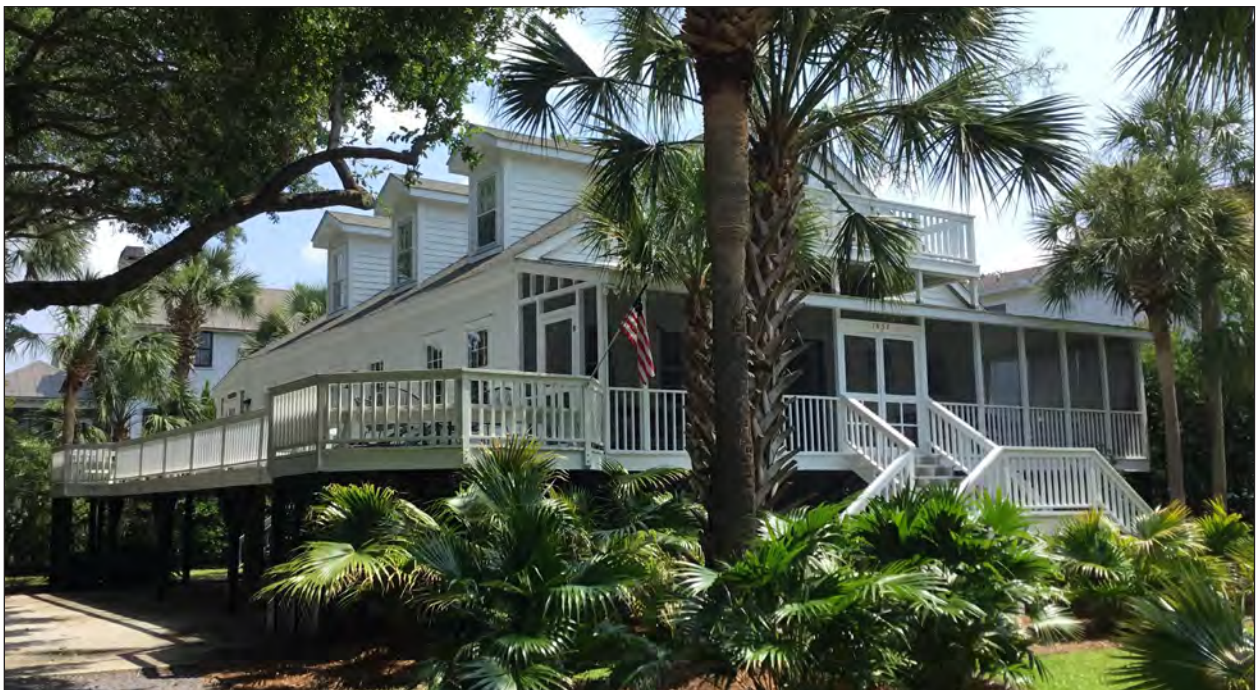
B. Circa 1888 Residence at 1656 Atlantic Avenue, SHPO Site Number 8765
