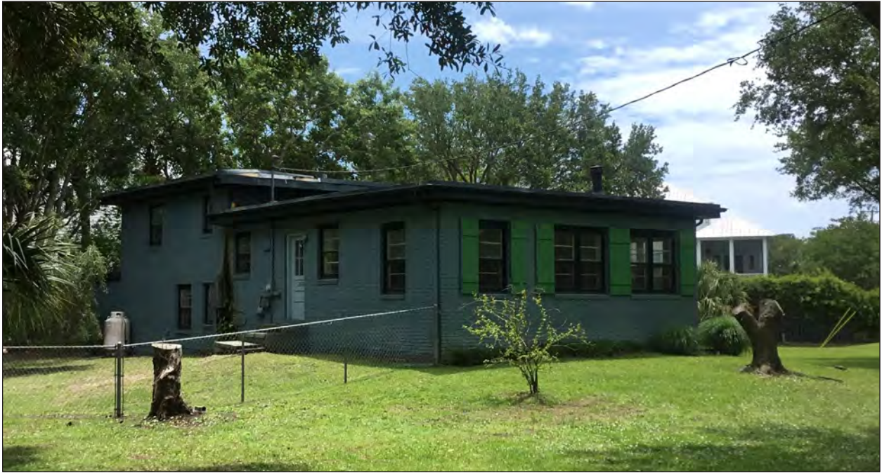
A. Flat-Roofed Type at 2851 I'On Avenue, SHPO Site Number 8607
