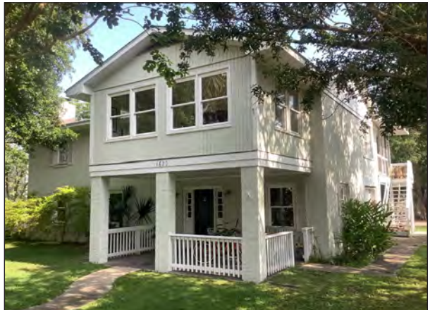
D. 1620 Middle Street, SHPO Site Number 8771
