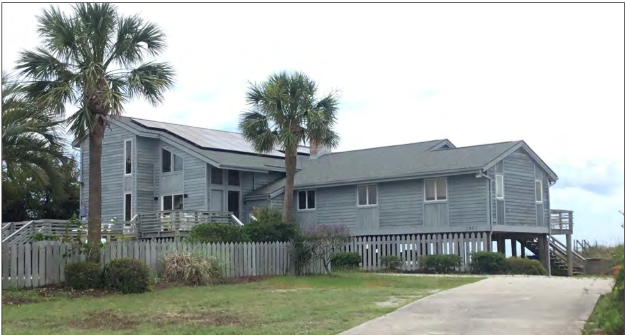
B. Gabled Type at 2905 Marshall Boulevard, SHPO Site Number 8589
