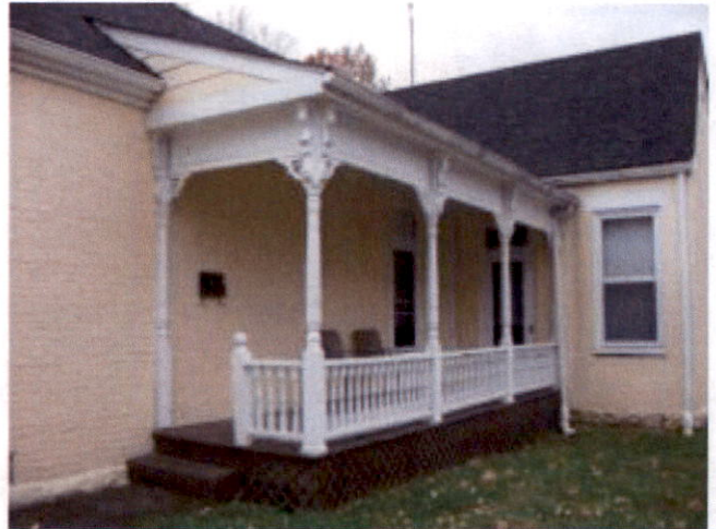
Many dwellings retain late nineteenth-century milled porch columns and detailing (311 W. Second Street).
