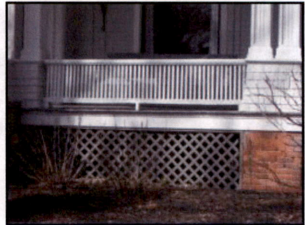
Appropriately designed and placed lattice panels between the porch foundation piers at 650 Jackson Street, SE.
