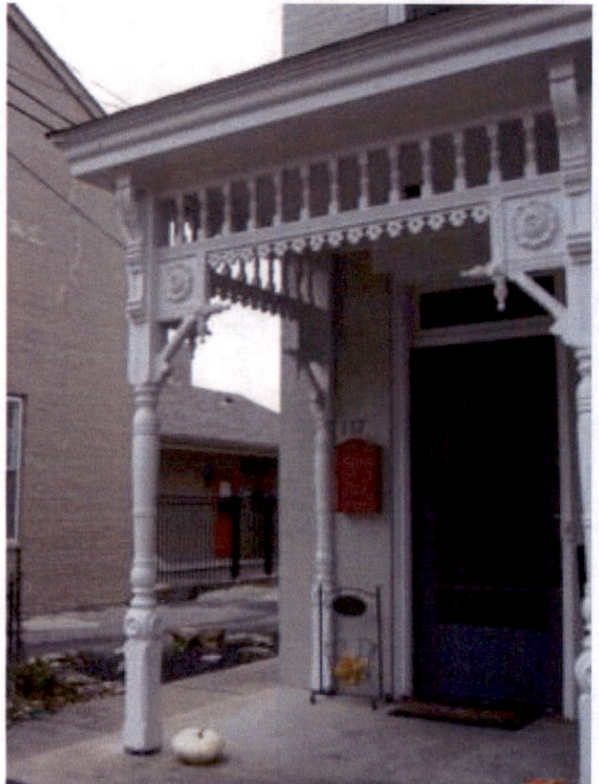
Some mid-nineteenth century dwellings were remodeled with added decorative wood porches at a later time as at 117 W. Third Street.
