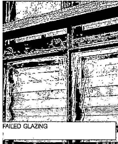
NON ORIGINAL- DETERIORATED WOOD RAIL & SASH
