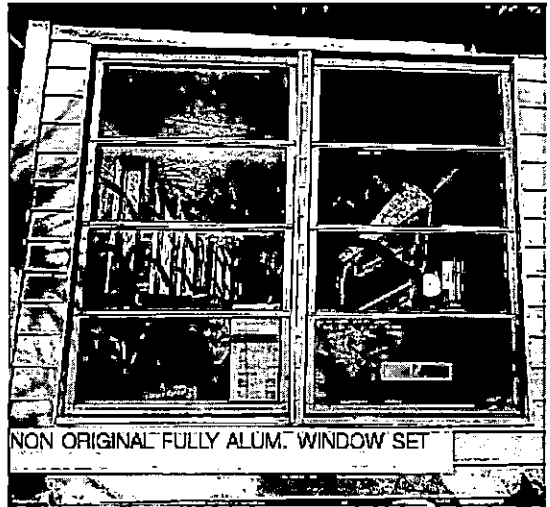
NON ORIGINAL ALUM. WINDOW DETAIL
