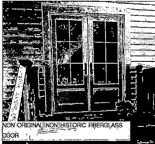
NON-ORIGINAL NON-HISTORIC FIBERGLASS DOOR
