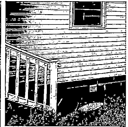
NON-ORIGINAL NON-HISTORIC CONCRETE STAIRS & VINYL SIDING
