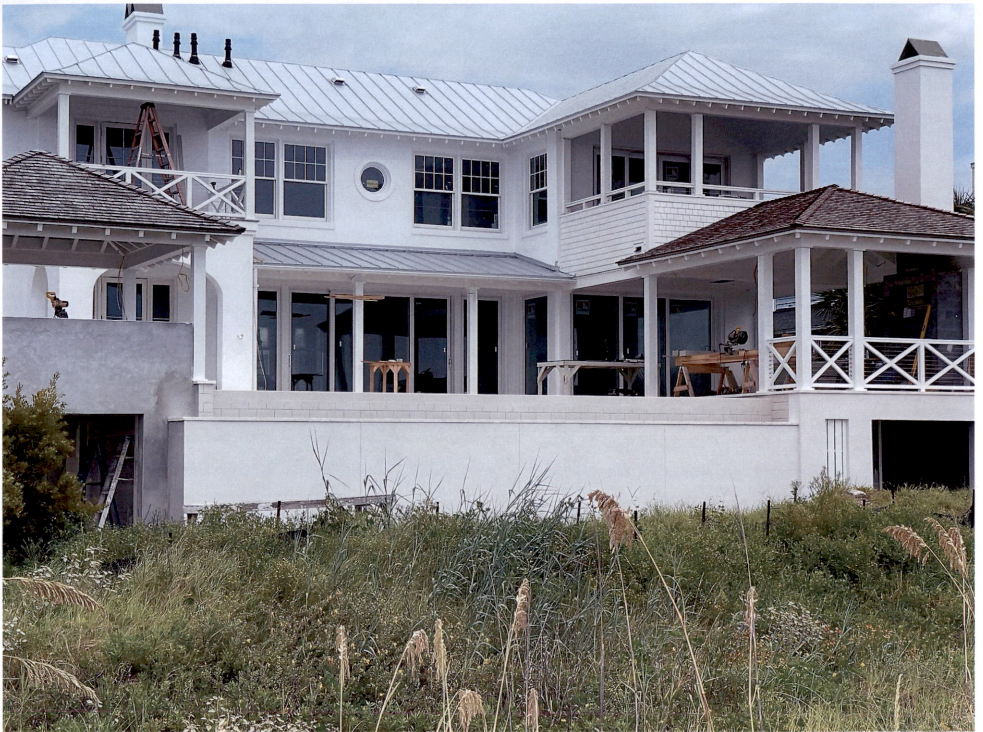
2863 MARSHALL BLVD. – CURRENTLY UNDER CONSTRUCTION
