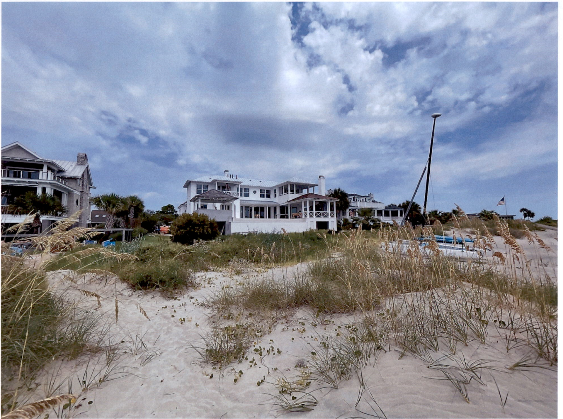
2863 MARSHALL BLVD. - CURRENTLY UNDER CONSTRUCTION
