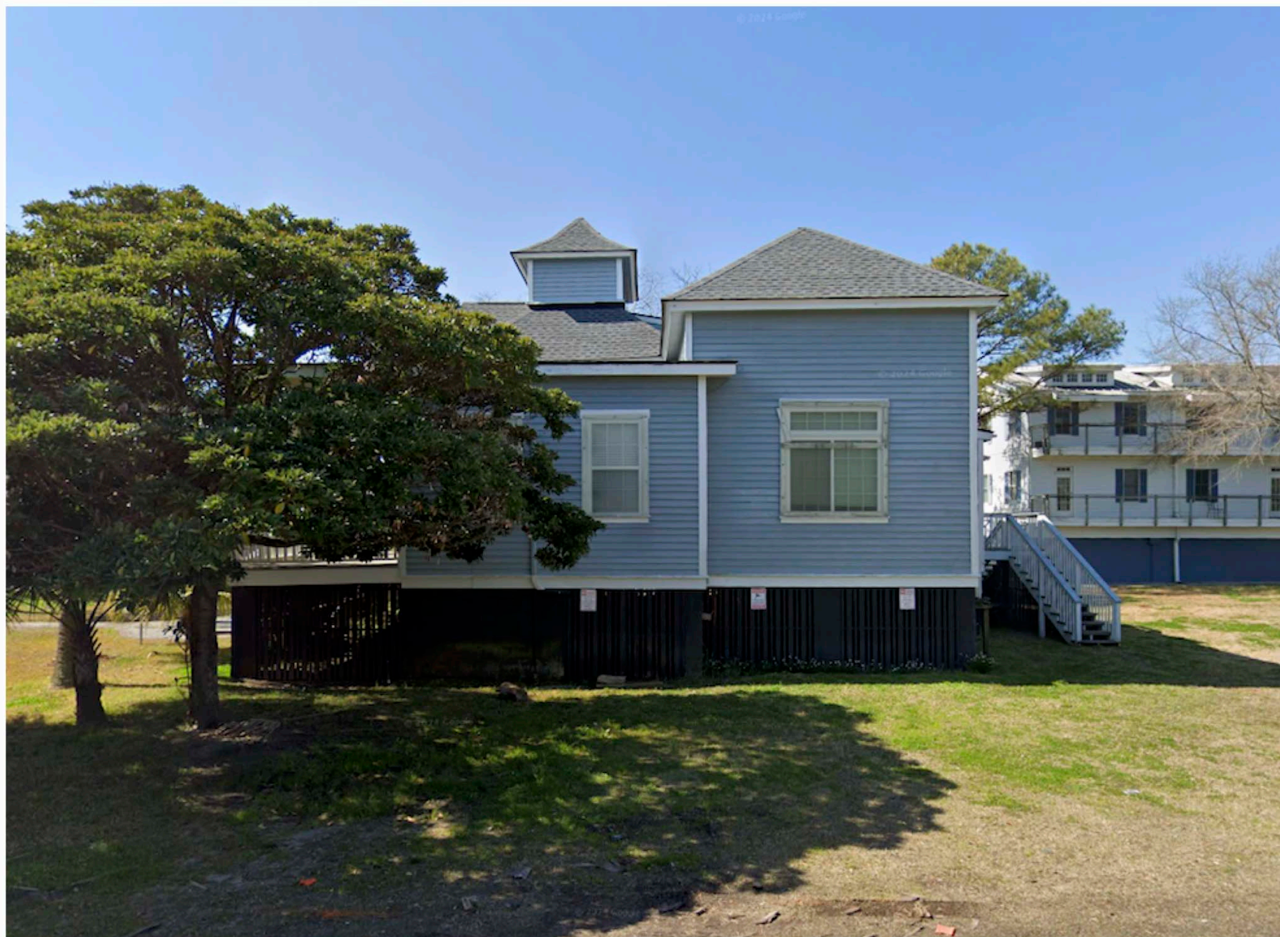
EAST (STATION 22 STREET) VIEW
