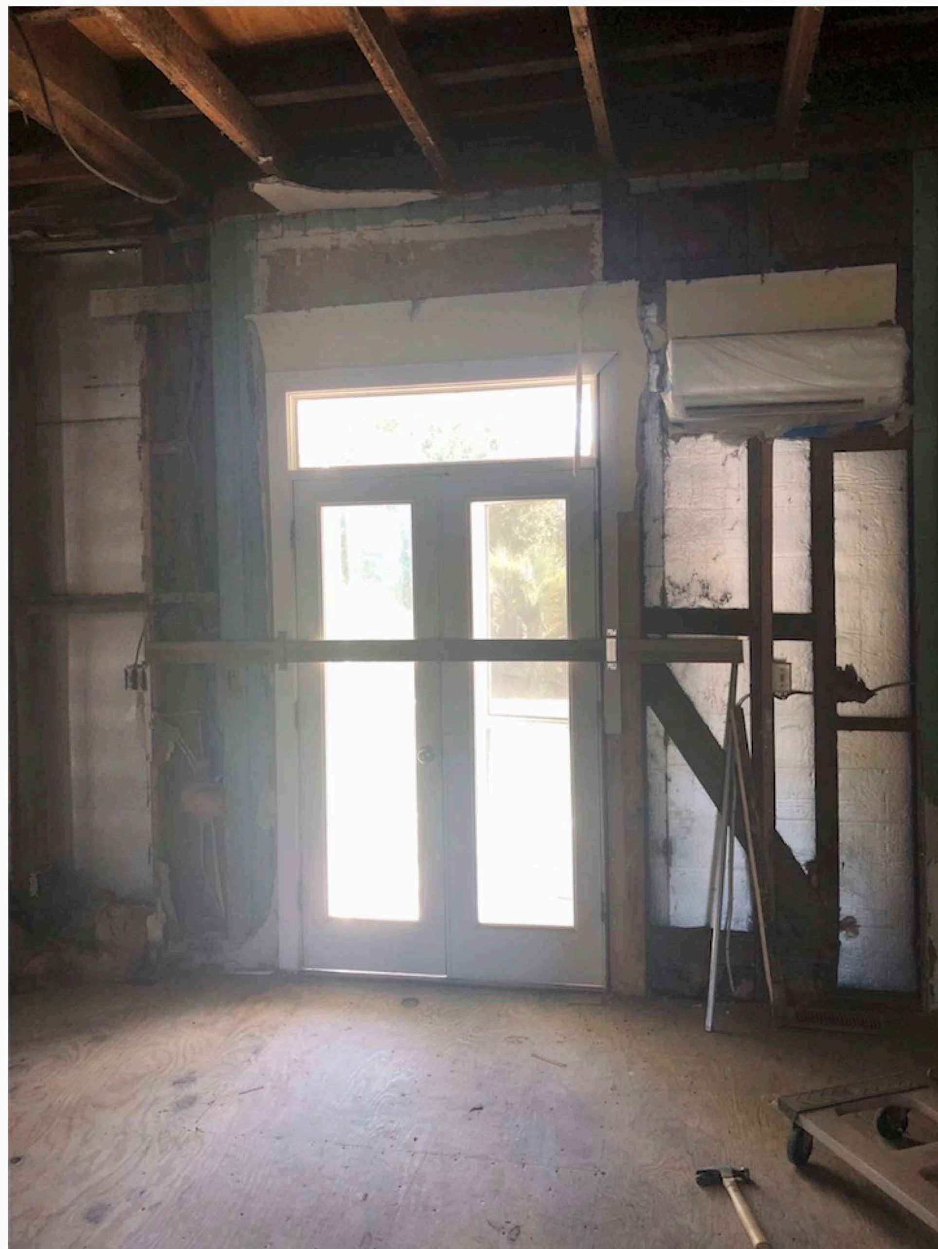
NONHISTORIC FIBERGLASS DOORS @ FRONT (ION AVENUE)
