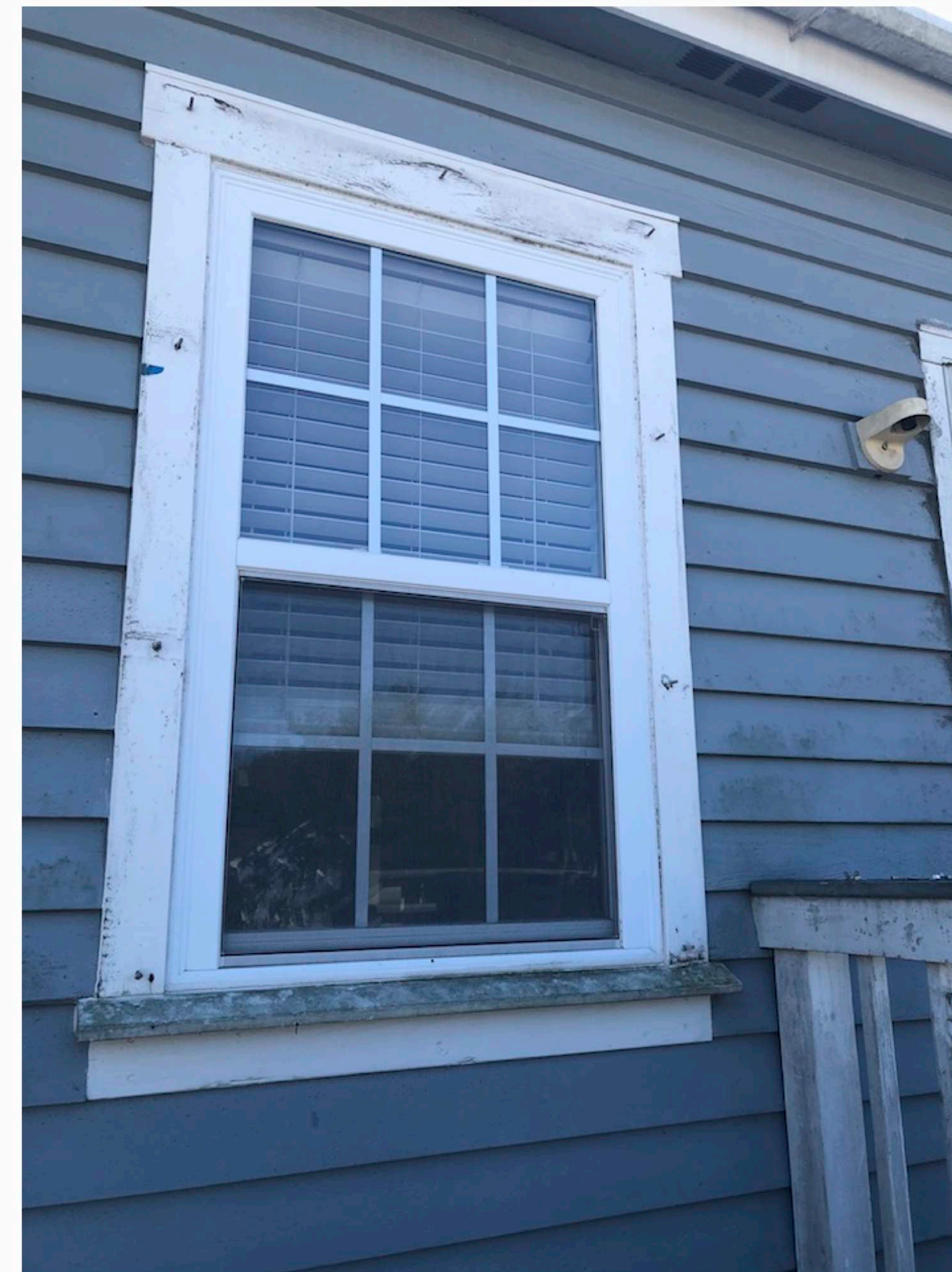
NONHISTORIC VINYL WINDOW, TYP. *note the simulated muntins/grilles: located between insulated glass
