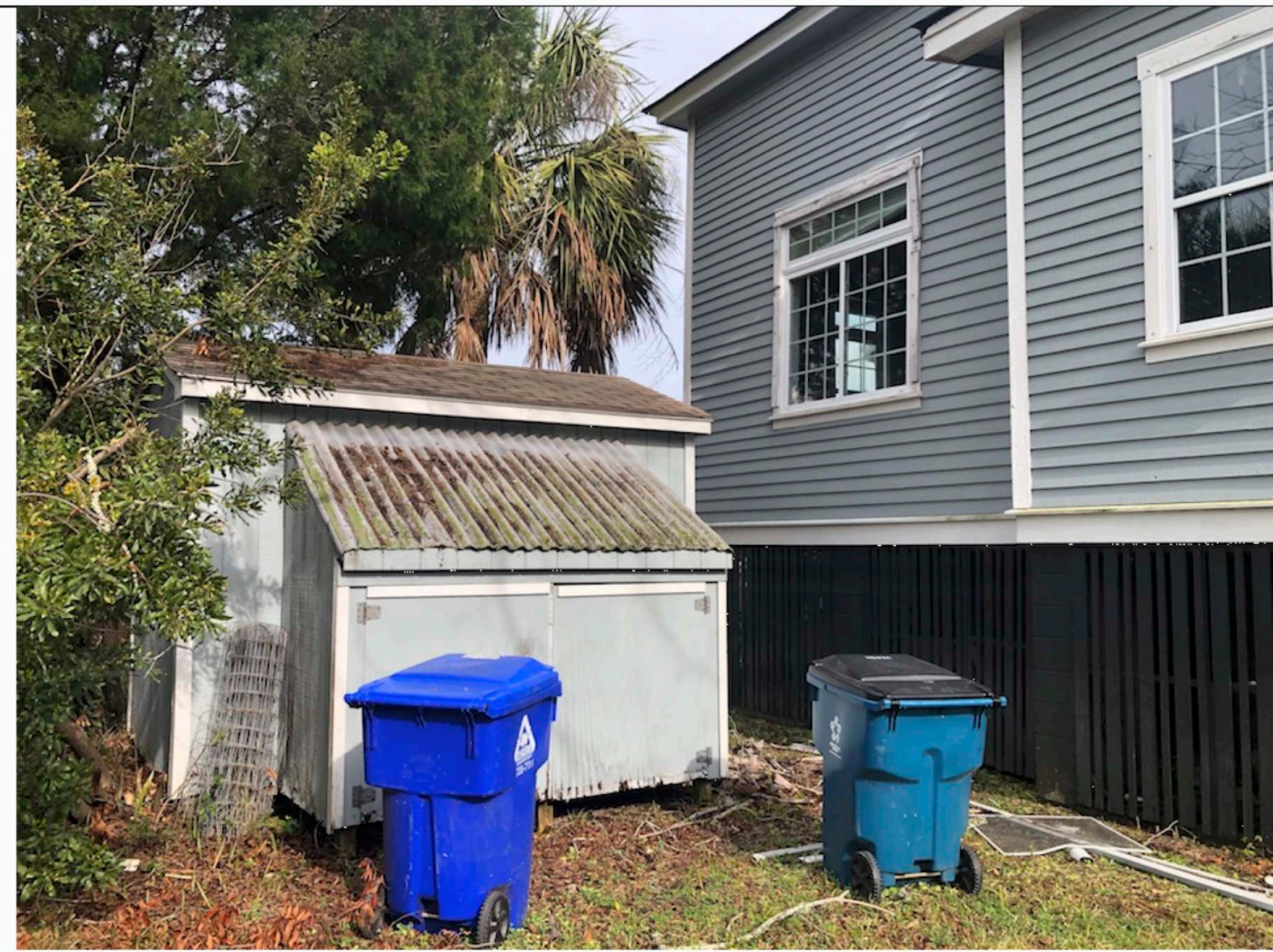
VIEW FROM ION AVENUE
