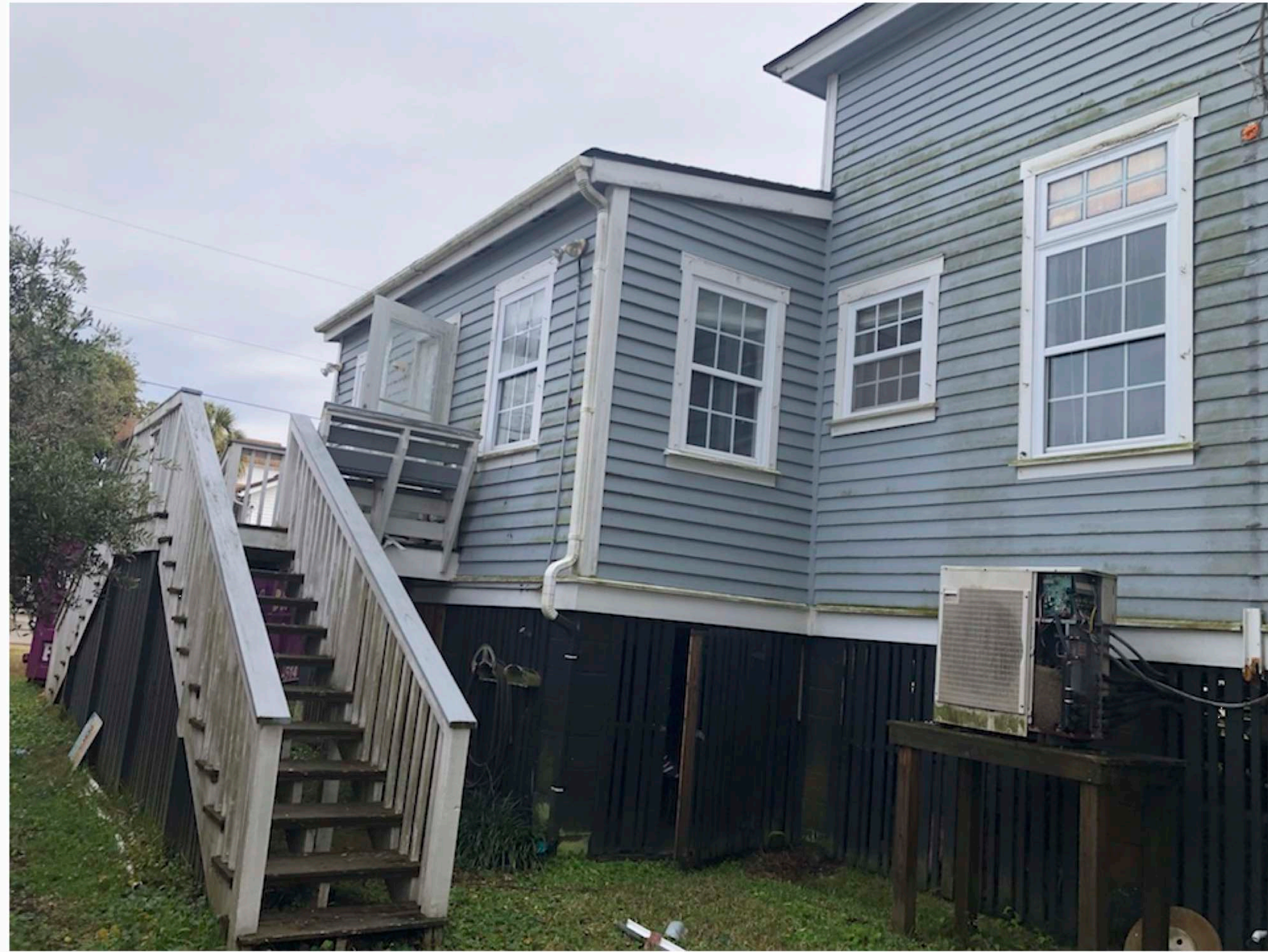
NORTH (REAR) VIEW
