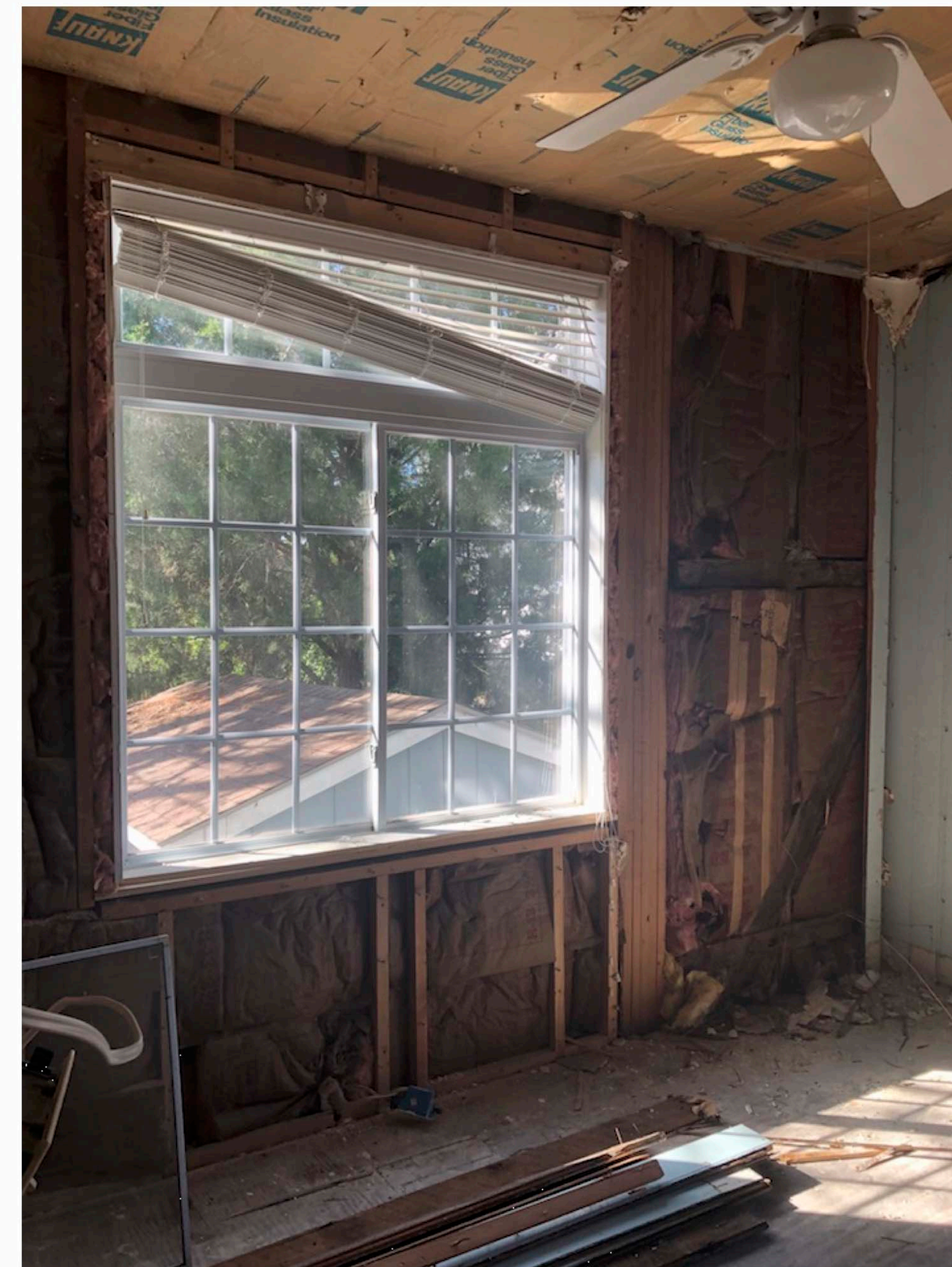
NONHISTORIC VINYL WINDOWS @ SIDE (STATION 22 STREET)
