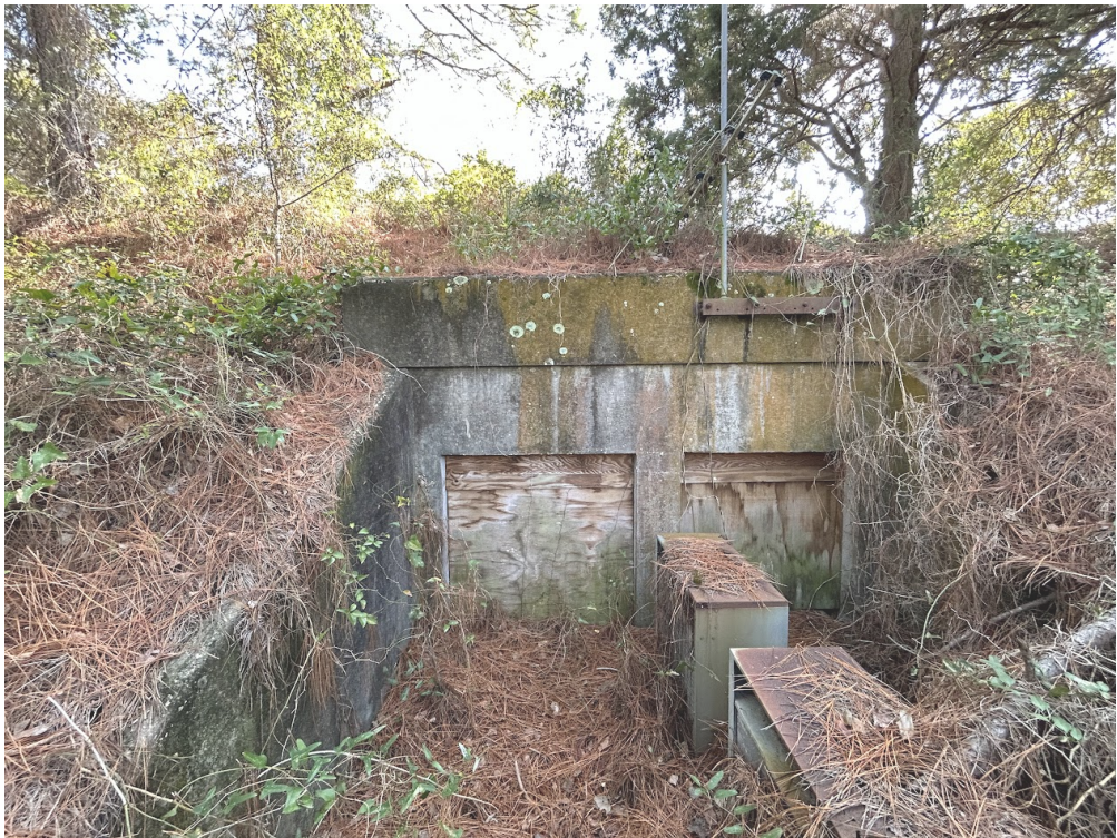
HISTORIC BUNKER HVAC OPENING ON ION AVENUE
