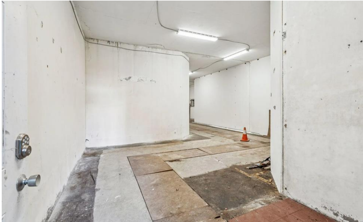
Interior views from the property listing show concrete interior walls that are nearly two foot thick, with concrete ceilings lined with electrical conduit above. The steel doors show evidence of corrosion from exposure to moisture and salt air. Previous owners cut into the concrete slab floor to run systems, denoted by the osb plywood coverings.
