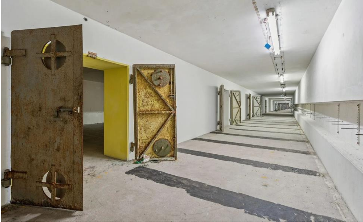
Another view of the hallway, showing the width of the interior concrete walls.
