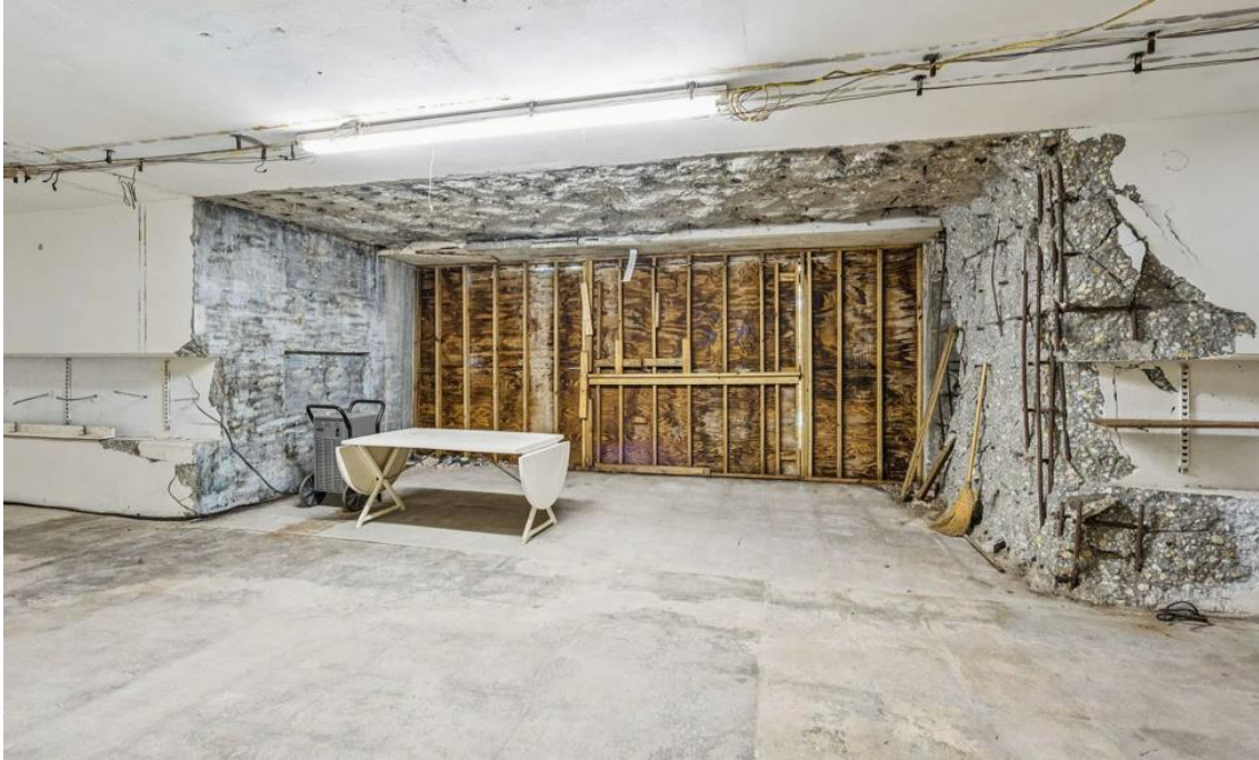
An entrance that Mr. Curd blew through the ten-foot-thick Brownell Avenue facing side of the bunker to create a window opening. It has been enclosed with plywood and dimensional framing and is partially backfilled with earth on the exterior. Note the rebar sticking through the concrete.
