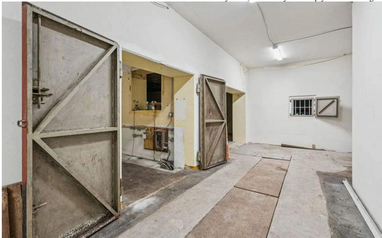
Interior views from the property listing show concrete interior walls that are nearly two foot thick, with concrete ceilings lined with electrical conduit above. The steel doors show evidence of corrosion from exposure to moisture and salt air. Previous owners cut into the concrete slab floor to run systems, denoted by the osb plywood coverings.
