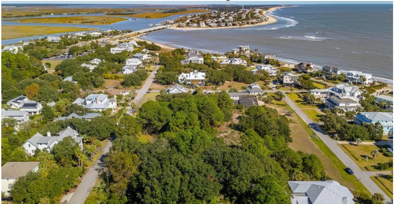
Aerial view of the property show it covered with earth and vegetation, which hides it from view as was the intention when it was used as munitions storage for the gun mounts on either side.
