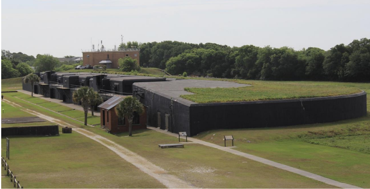
Battery Jasper in a recent photograph. National Park Service.
