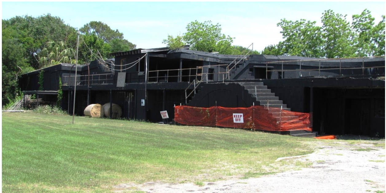
Recent photo of Battery Thomson, which is no longer accessible but which is often explored by island youths, by Brian Stansberry.
