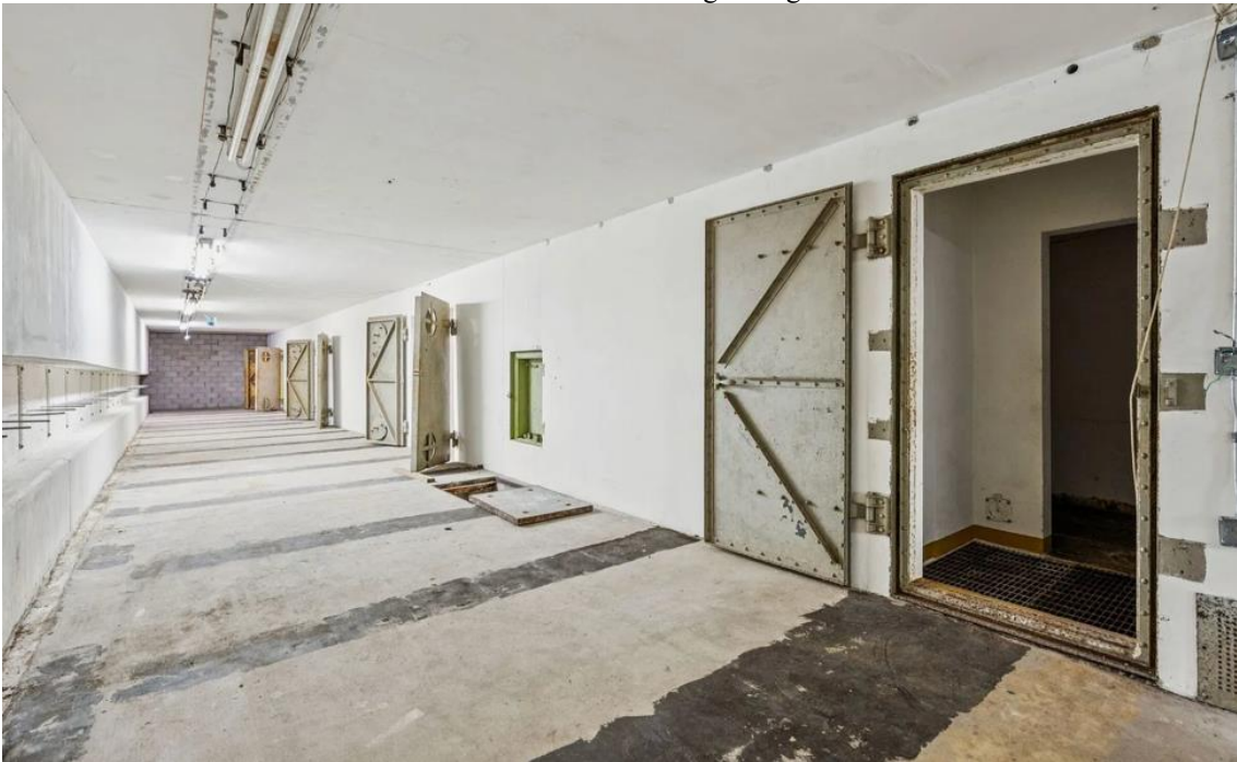
One of the bunker hallways, constructed of concrete for the walls, floor, and ceiling, and with riveted bombproof metal doors leading into storage rooms.
