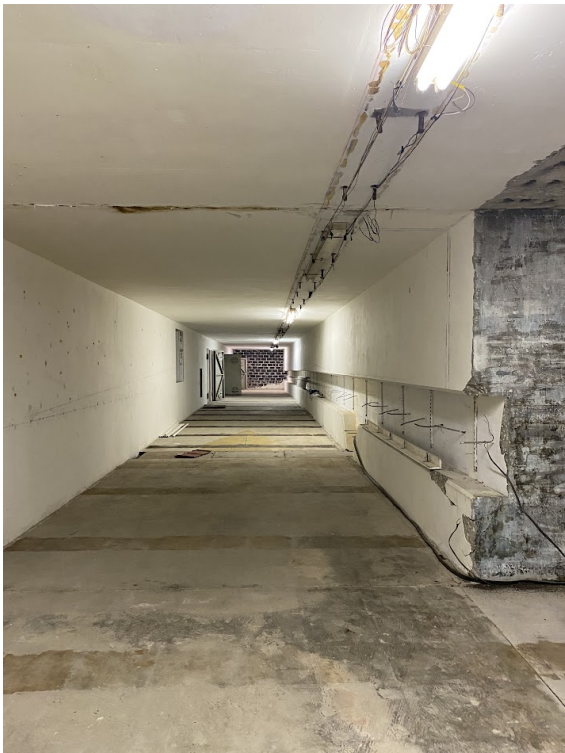
HISTORIC BUNKER INTERIOR
