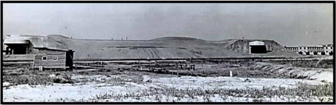
Figure 3.110: 1945 U.S. Army Photograph of Battery 520’s two casemated gun opening with connecting magazines protected by the large concrete and earth mound between the two openings. Image also shows the Overseas Discharge and Replacement Depot barracks buildings in the background that had been converted for use by the soldiers manning the Marshall Reservation’s 155mm guns. Courtesy of the National Archives, Record Group 338, Box 139, General Correspondence Relating to Places, compiled 1936 – 1945, Ft Moultrie, College Park, MA.
