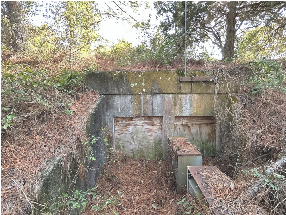
HISTORIC BUNKER HVAC OPENING ON ION AVENUE
