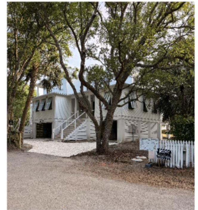
NEW HOUSE @ END OF 18
