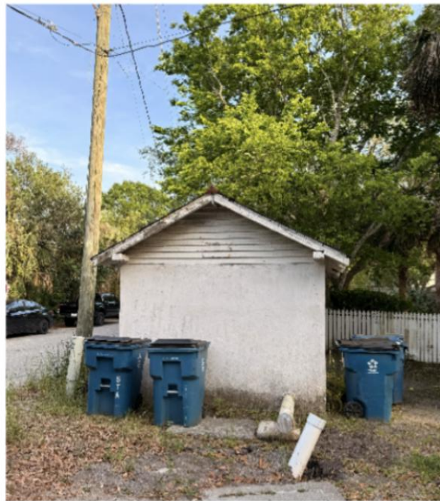
PUMP HOUSE @ CORNER
