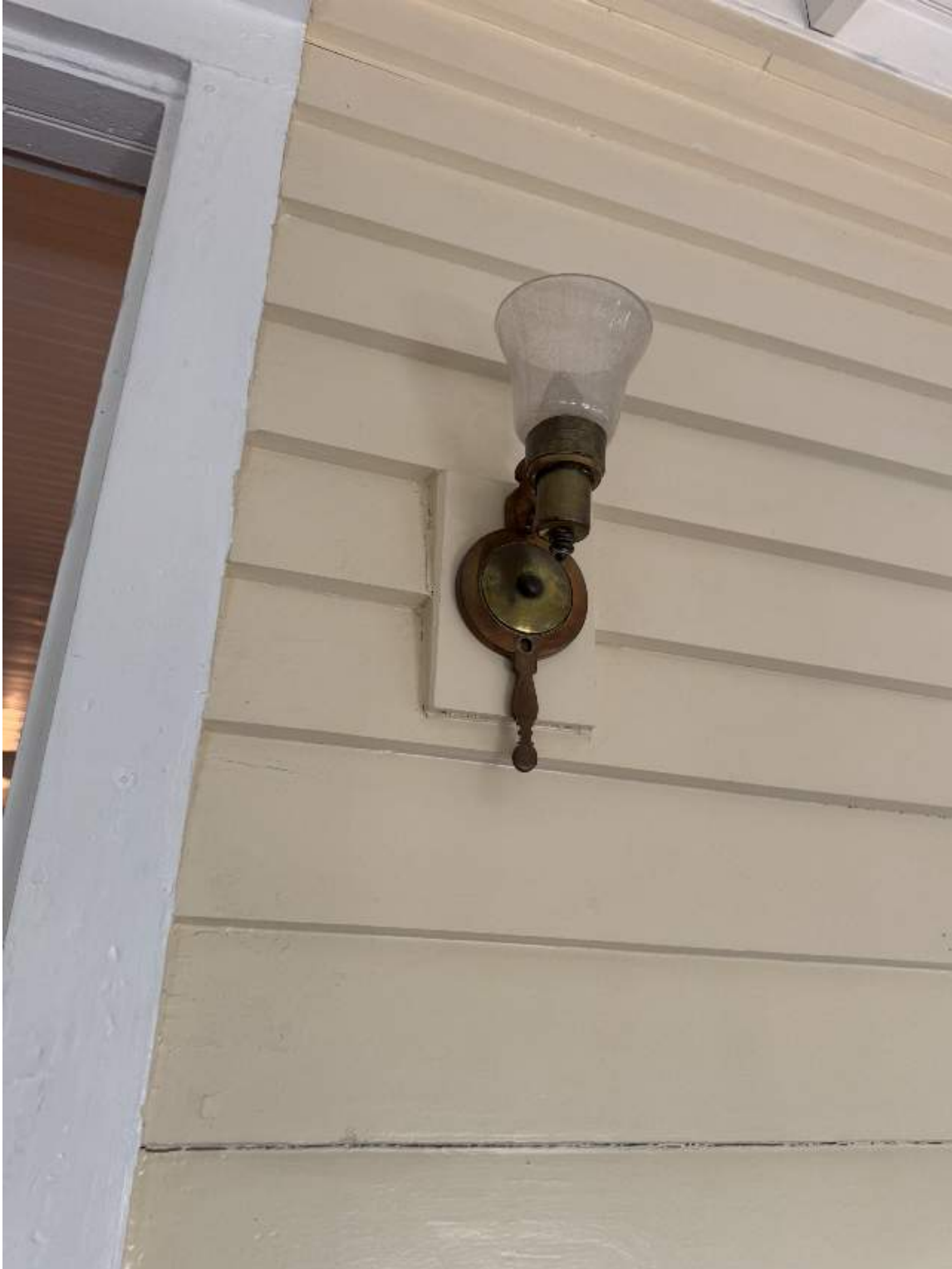
Siding and light fixture left inside the enclosed porch.
