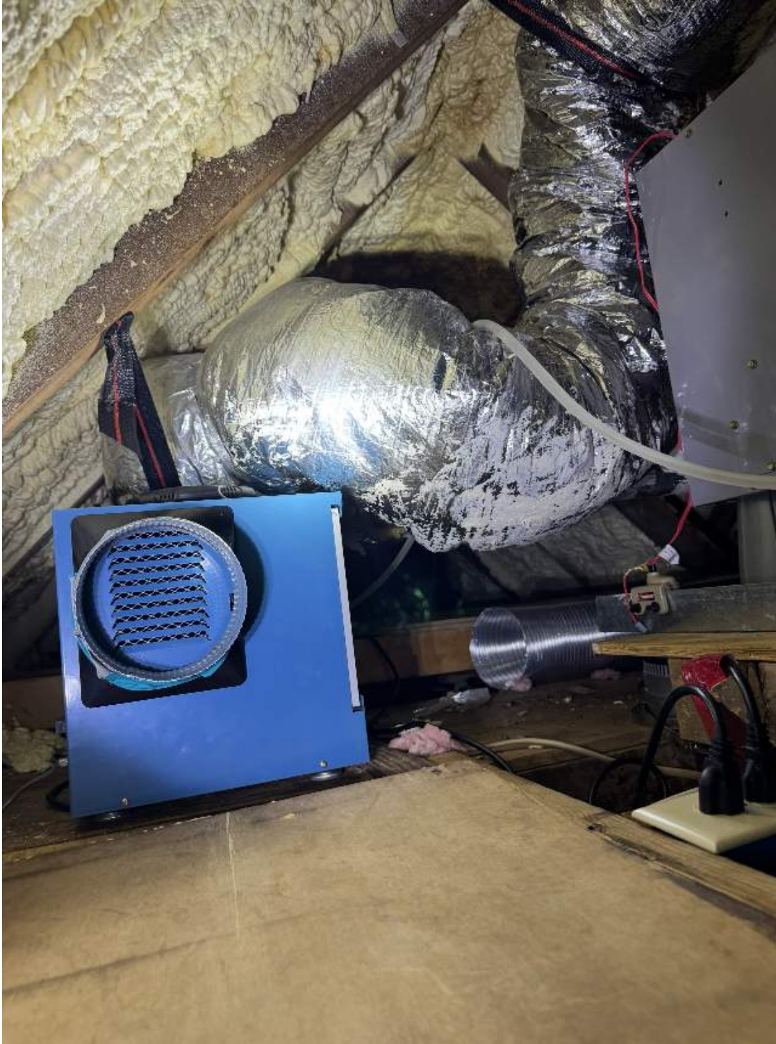
Inside the attic, looking down the side gable.
