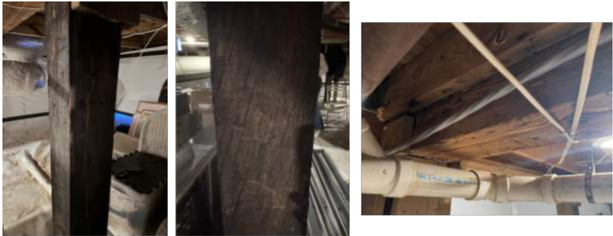
Large timbers used in construction. Viewed from the crawlspace.
