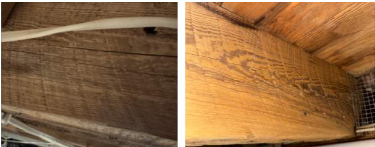
Circular saw marks on first floor joists.
