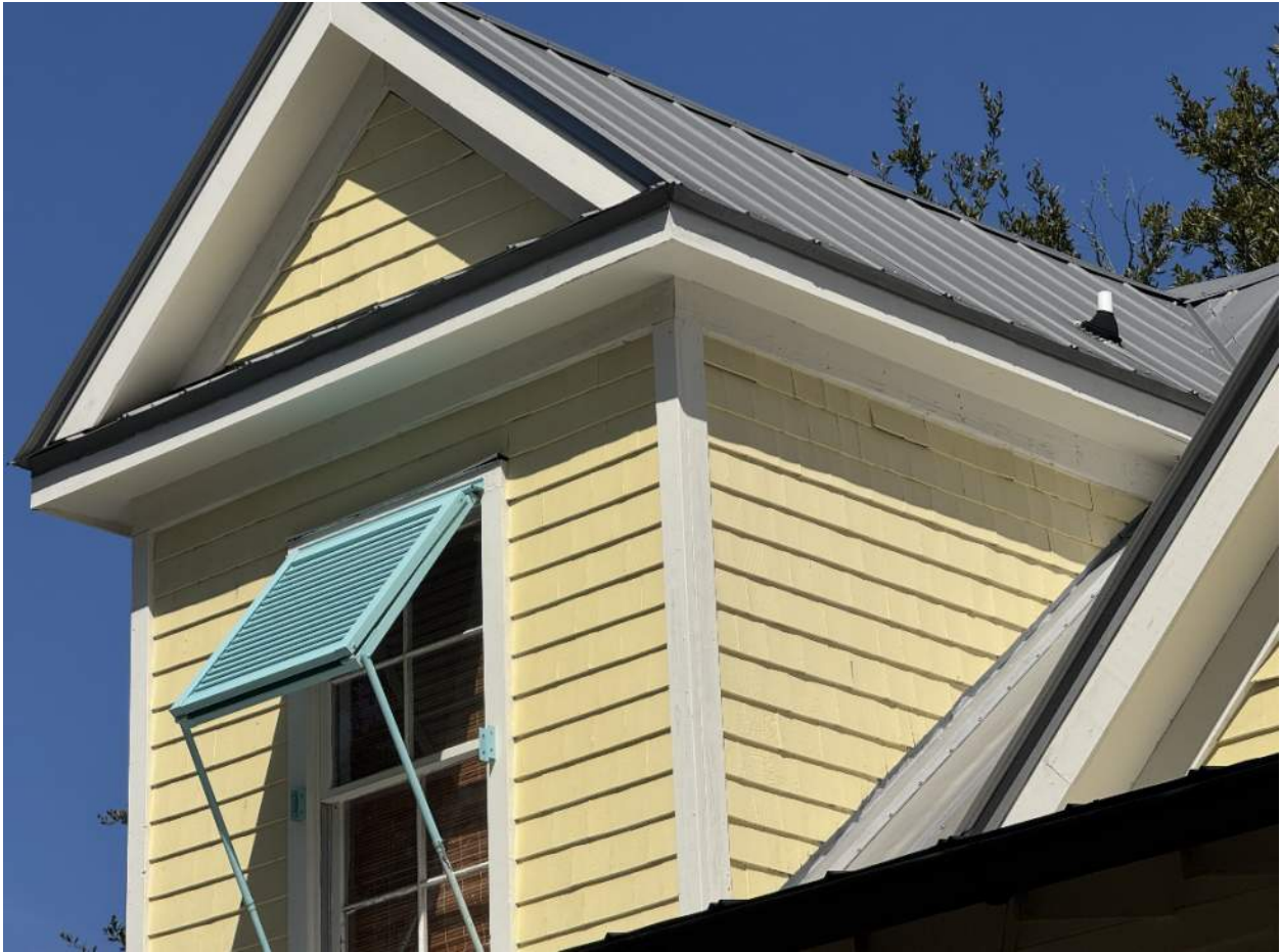
Shingle detail on dormer, south facade.
