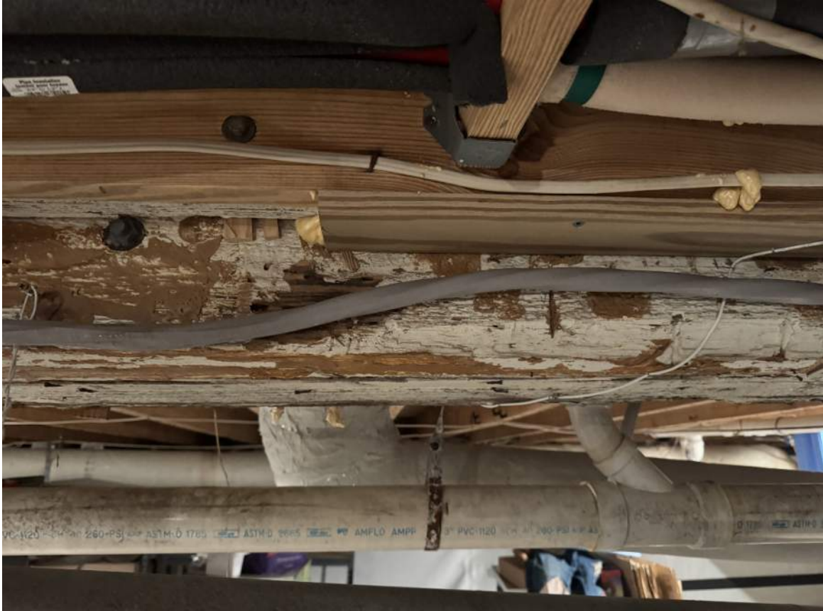
Axe marks visible in reclaimed floor joist.
