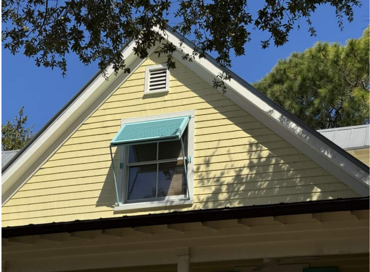
Gable detail, south facade.
