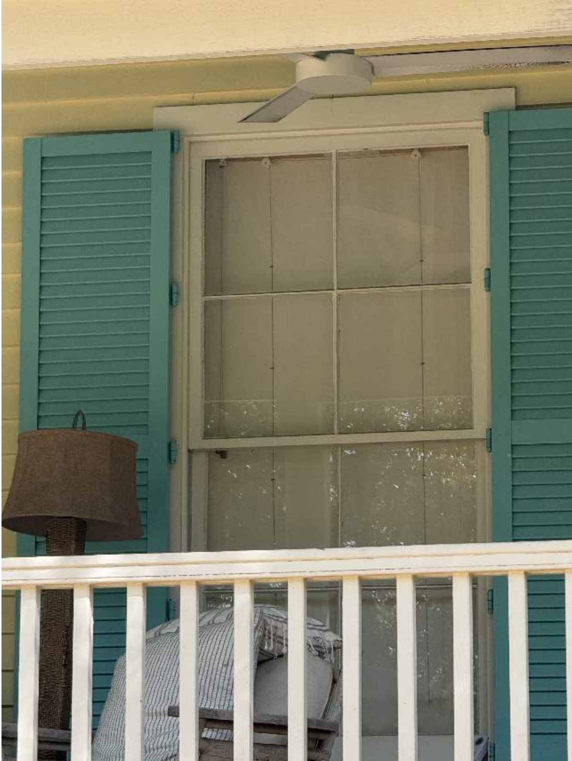
Window detail, south facade.
