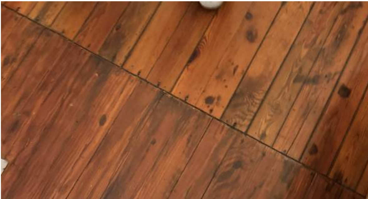
Difference in flooring between addition (bottom) and original main house (top).
