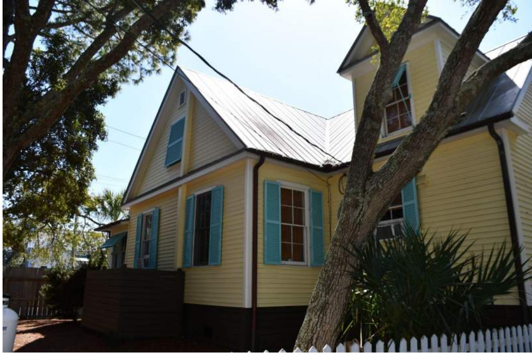
The north facade.
