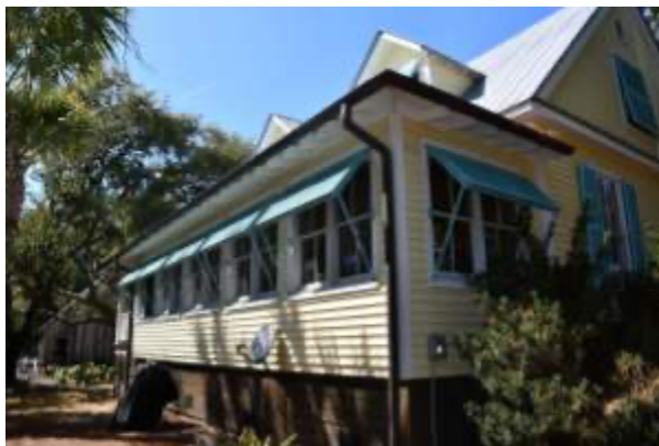
The enclosed porch facing Jasper Blvd. March 4, 2026.
