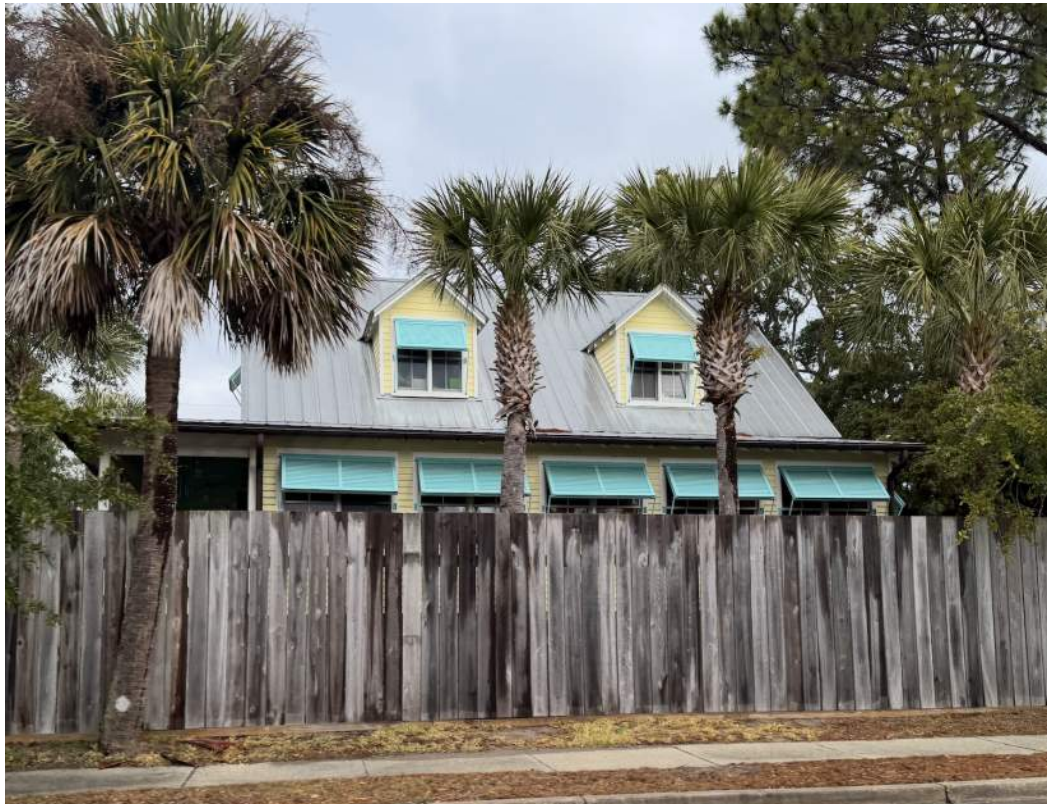
The east facade, viewed from Jasper Boulevard.
