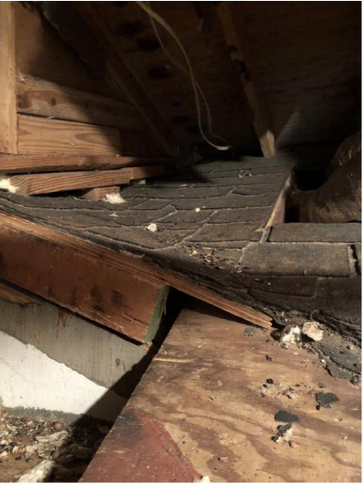
Images the end wall of the house, which has evidence of later repairs. The original back exterior wall of the house can be seen (painted grey and white) and the gable roof over the earlier iteration of the side ell.
