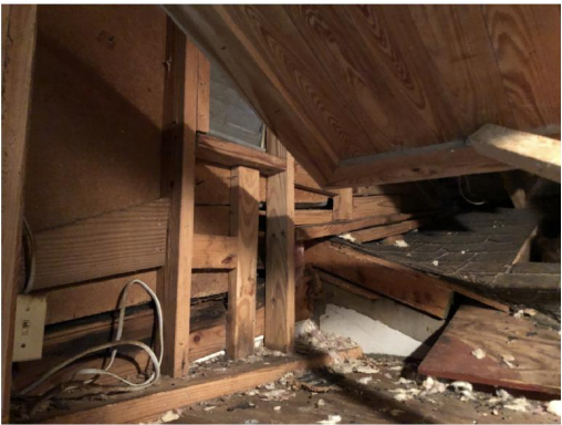
Images the end wall of the house, which has evidence of later repairs. The original back exterior wall of the house can be seen (painted grey and white) and the gable roof over the earlier iteration of the side ell.
