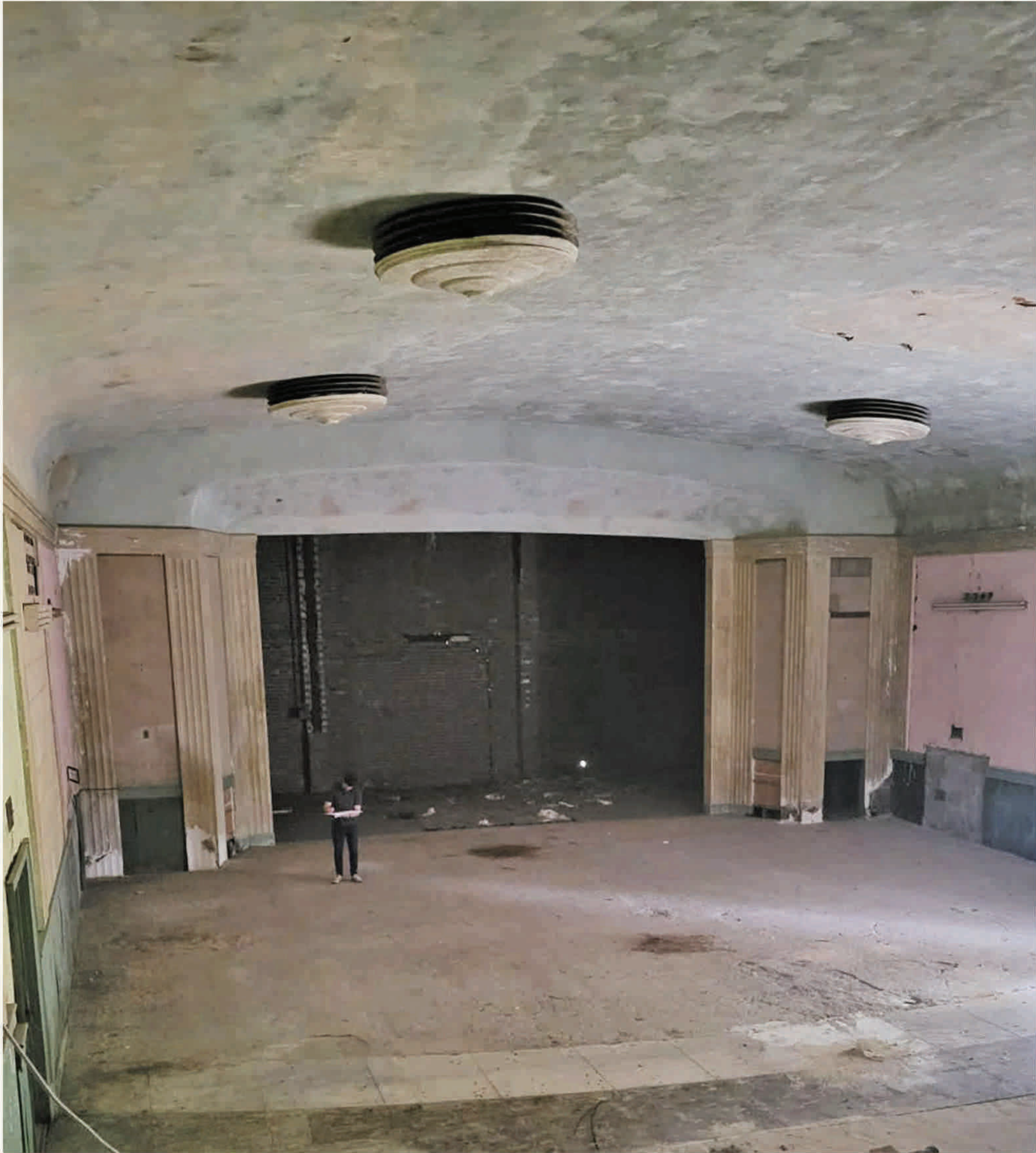
The theater interior as it exists today, with the screen removed and the seating area filled in. The lower exit doors have been bricked in and there is a general level of degradation of the plaster and wood finishes.
