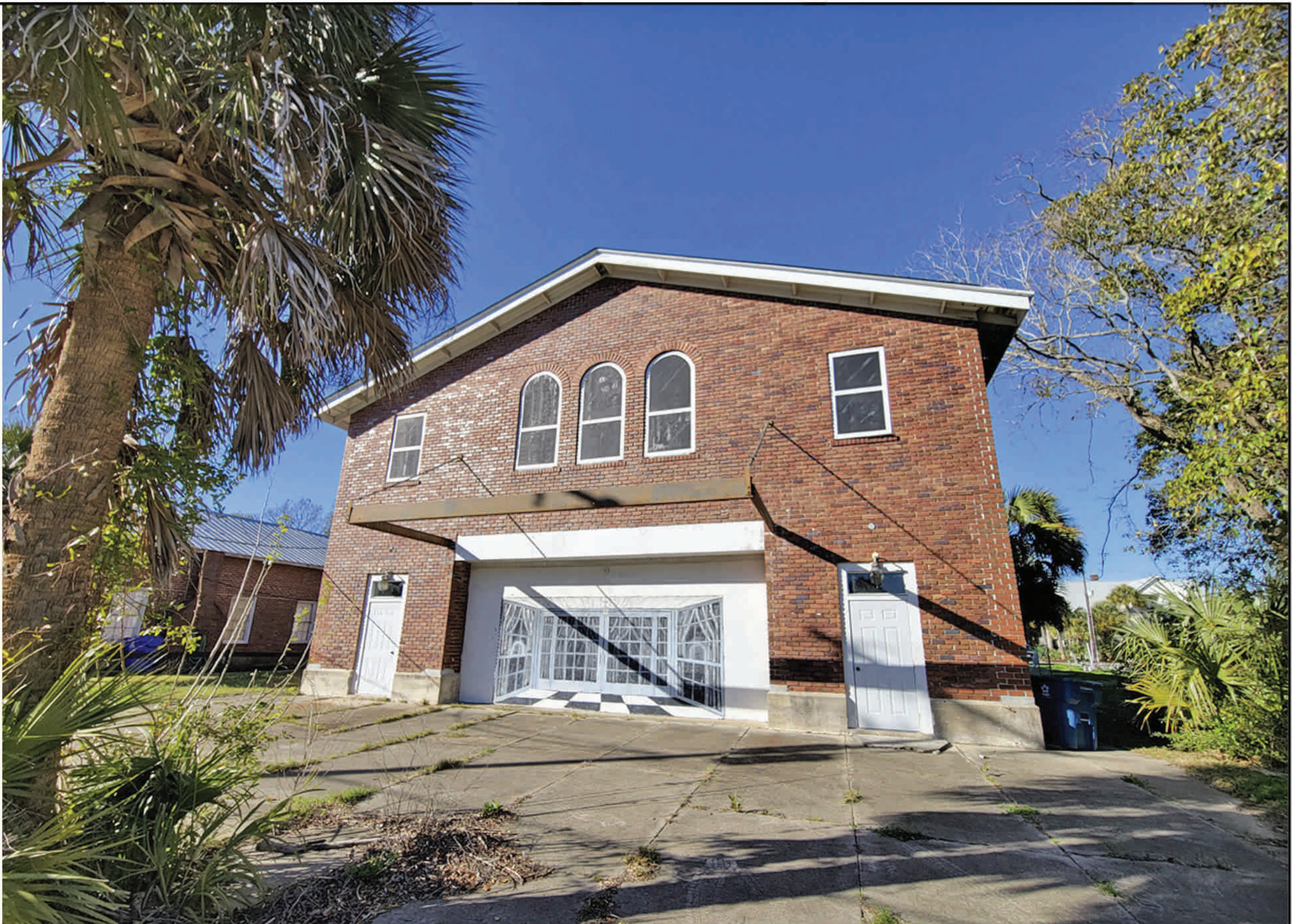
The Middle Street facade is the only formal facade, with an ordered series of doors and windows centered by three Roman-arched upper windows. The former recessed ticket and entry plaza has been covered with an infill wall.
