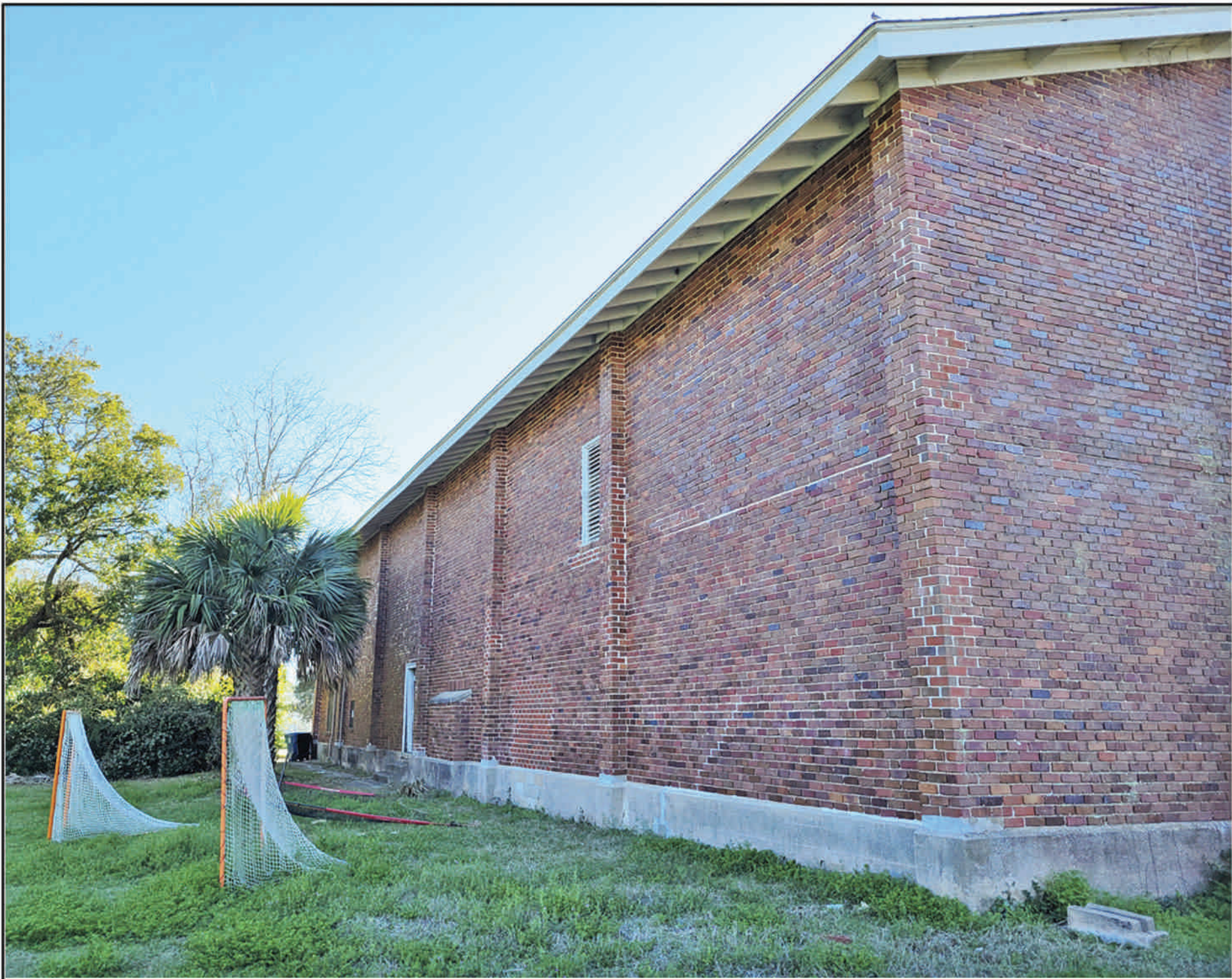
The side elevations are defined by a series of brick pilasters, with minimal windows and louvered ventilation openings.
