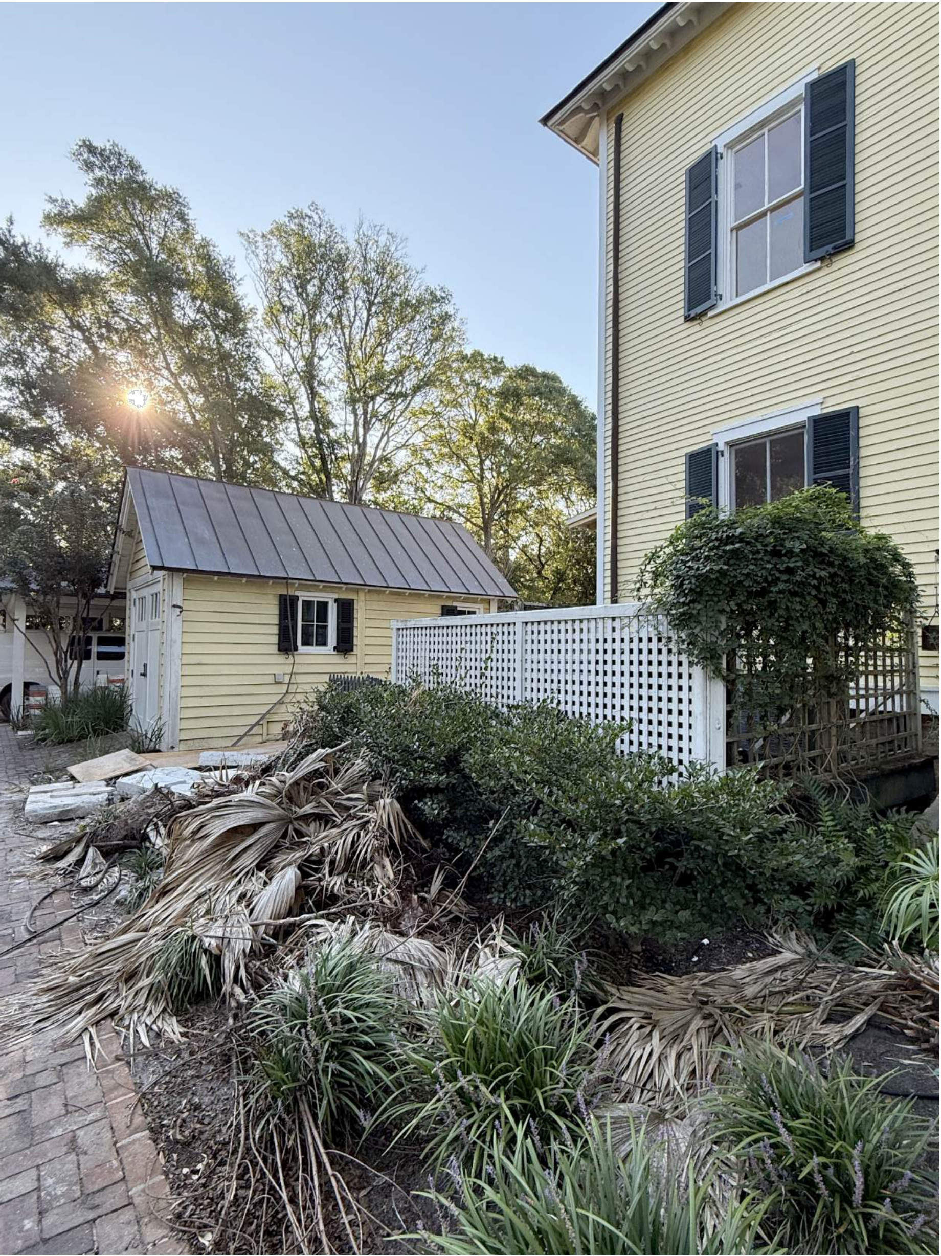
HVAC STAND LOOKING EAST
