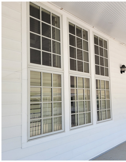
Asbestos siding and flush windows.
