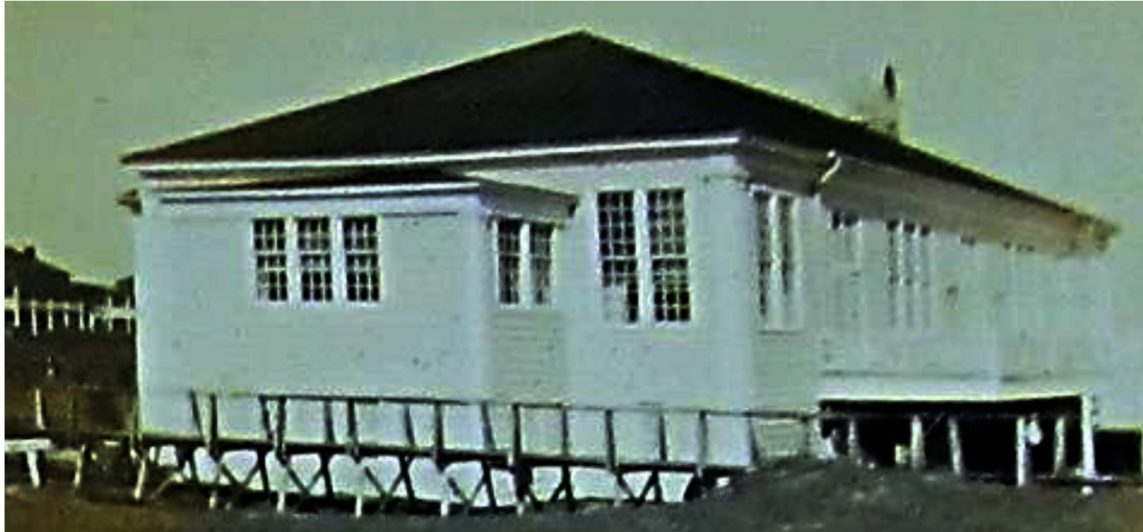
An early 1930s photo of Jasper Hall shows many of the original windows that have been closed in or covered.
