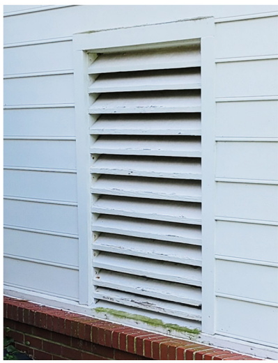
Diamond pattern vent grilles were replaced with louvers.
