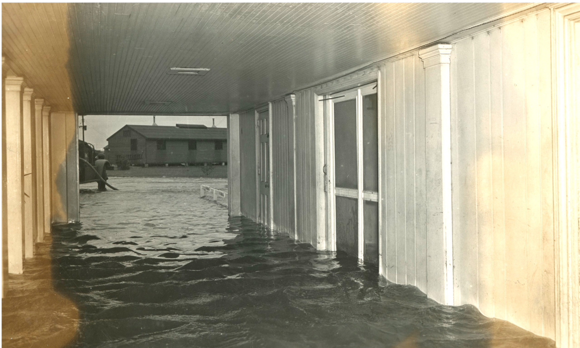
A view from inside Jasper Hall's historic drop-off. Screen doors to the right lead into the club lobby.
