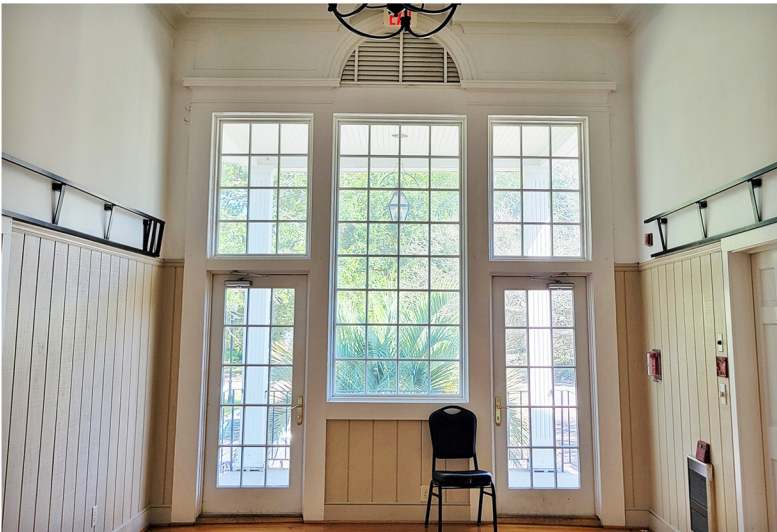
The round palladian window turned into an attic vent for the new portico.
