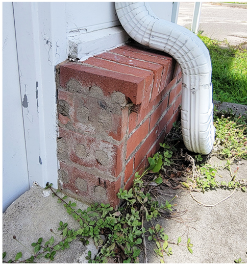
A poorly detailed brick water table was added to the base of the building.
