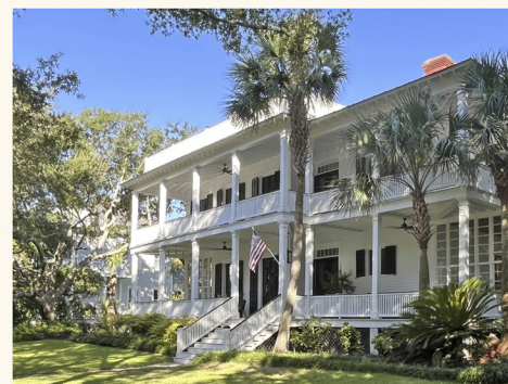
One of the historic Senior Officer's Residences with it's added widow's walk open porch above the two-story main porch.
