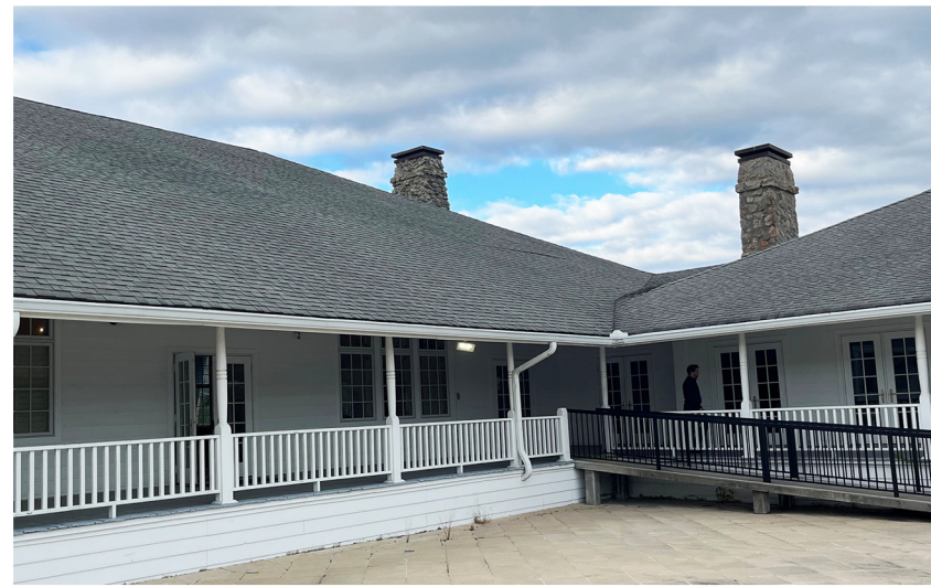
New porch roofs covered most of the architectural detail of the beach facade.
