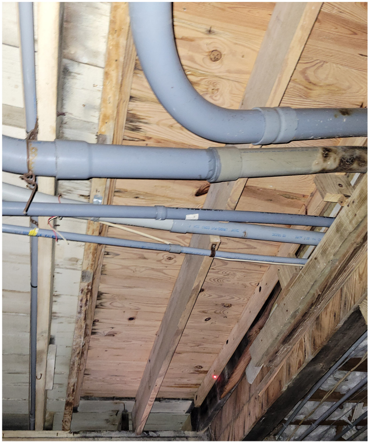
Ceiling/floor patched to close the former stairway opening.
