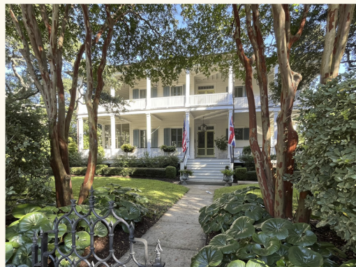
Jasper Hall was originally intended to be complimentary structure to the Senior Officers’ Residences, on which tow-level porches overlooking formal landscape is a common feature.
