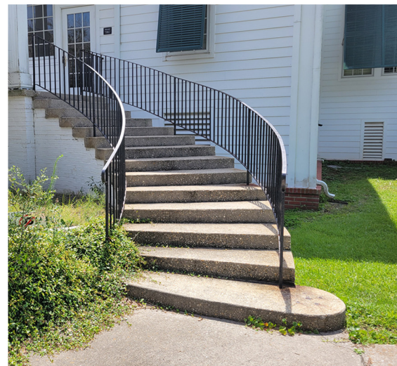
Mid-century exposed aggregate pebble concrete on stairs treads instead of natural stone.
