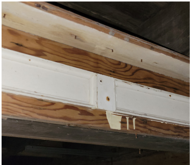
Vestiges of historic trim attached to ceiling structure.
