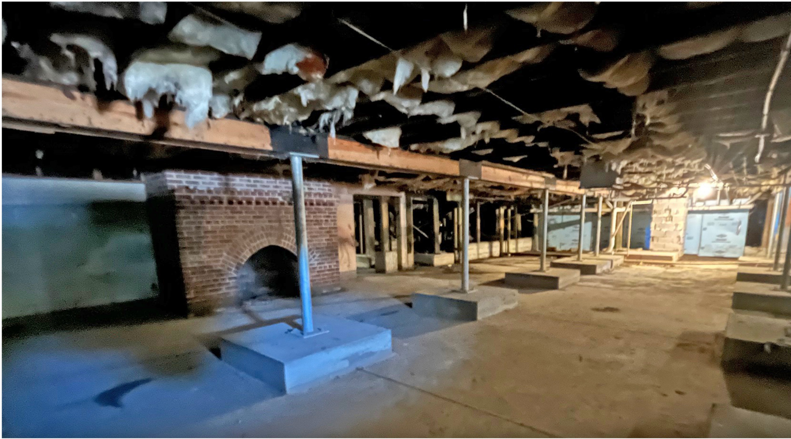
View of basement area that once housed the caretaker's apartment with its brick fireplace and shower stall still visible.
