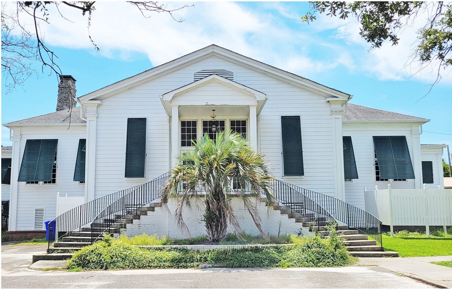
The new stair and portico solved a functional issue, but used details that were not compatible with the Island Beach Cottage character of the early 20th century Fort Moultrie architecture.
