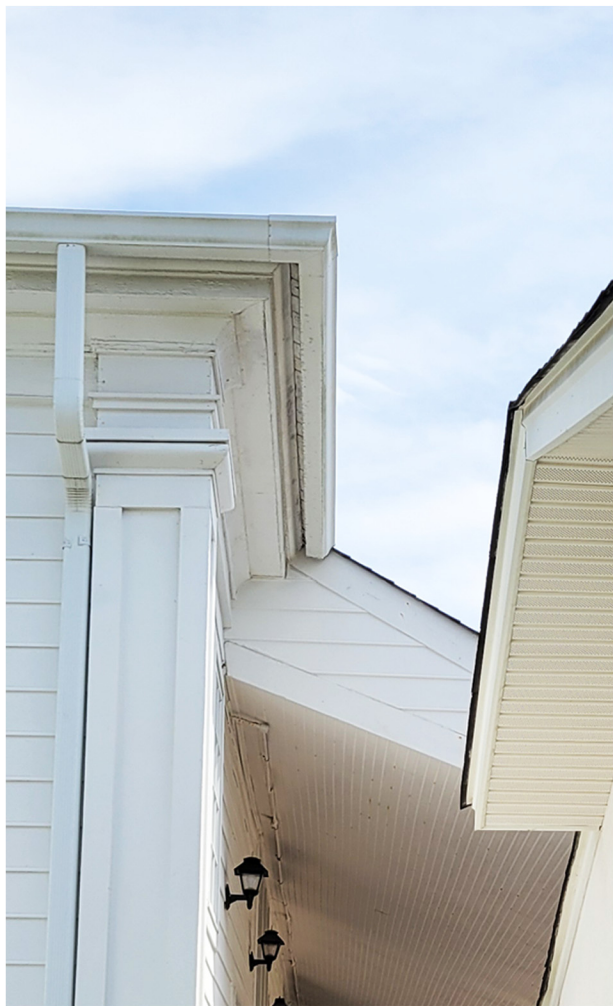
New porch roofs covered most of the decorative eave detailing on the beach facade.
