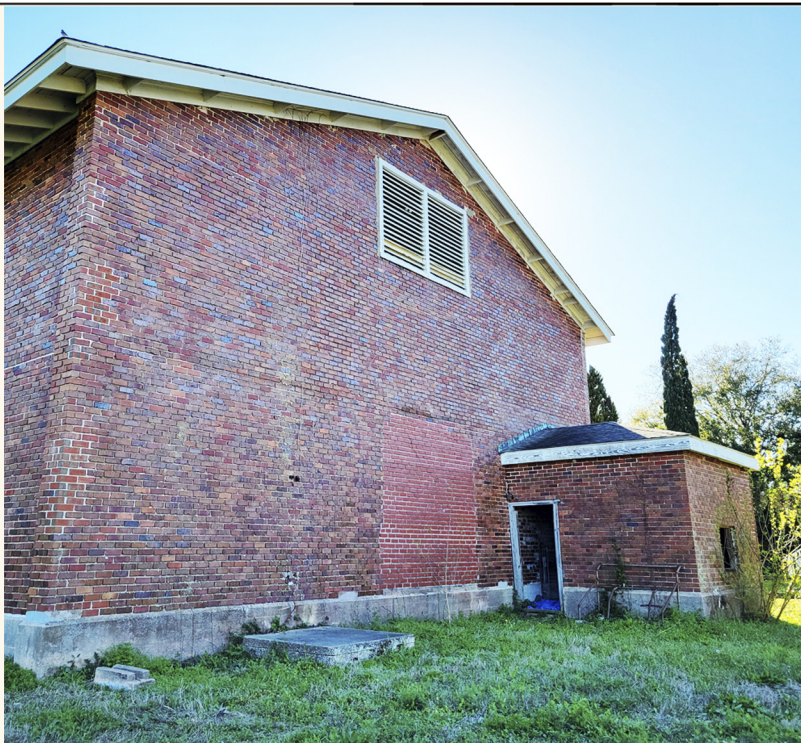
The Thompson Avenue facade with its louvered vent, the boiler room, and evidence of a rear opening that has been filled in.
