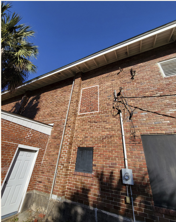
Evidence of filled historic openings on the side facade.
