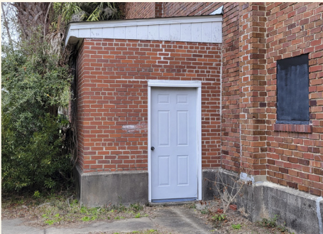
View of the smaller side boiler room.
