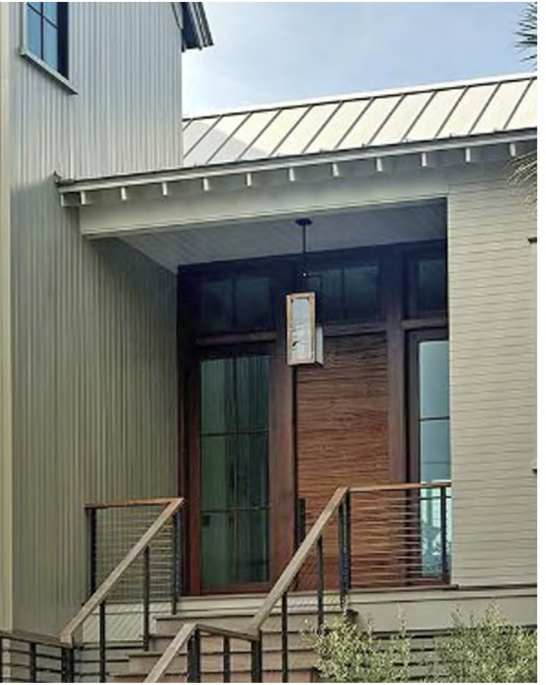
Precedent Image Solid wood door with full height sidelights, set back under cover.
