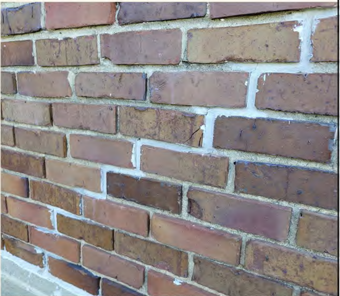
Incompatible brick repairs will need to be remediated to prevent further degradation of the brickwork..
