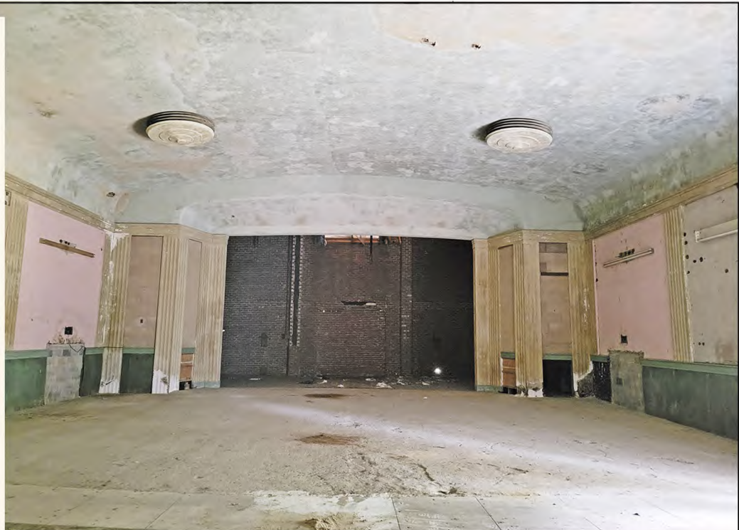
View of the formal proscenium and elliptical arched ceiling. The theater seating area has been filled in up to the level of the former stage.
