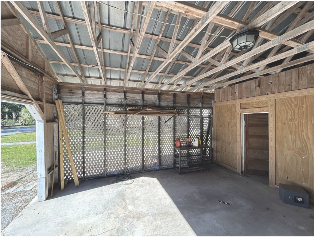
NEW ROOF TRUSSES AND WALL FRAMING
