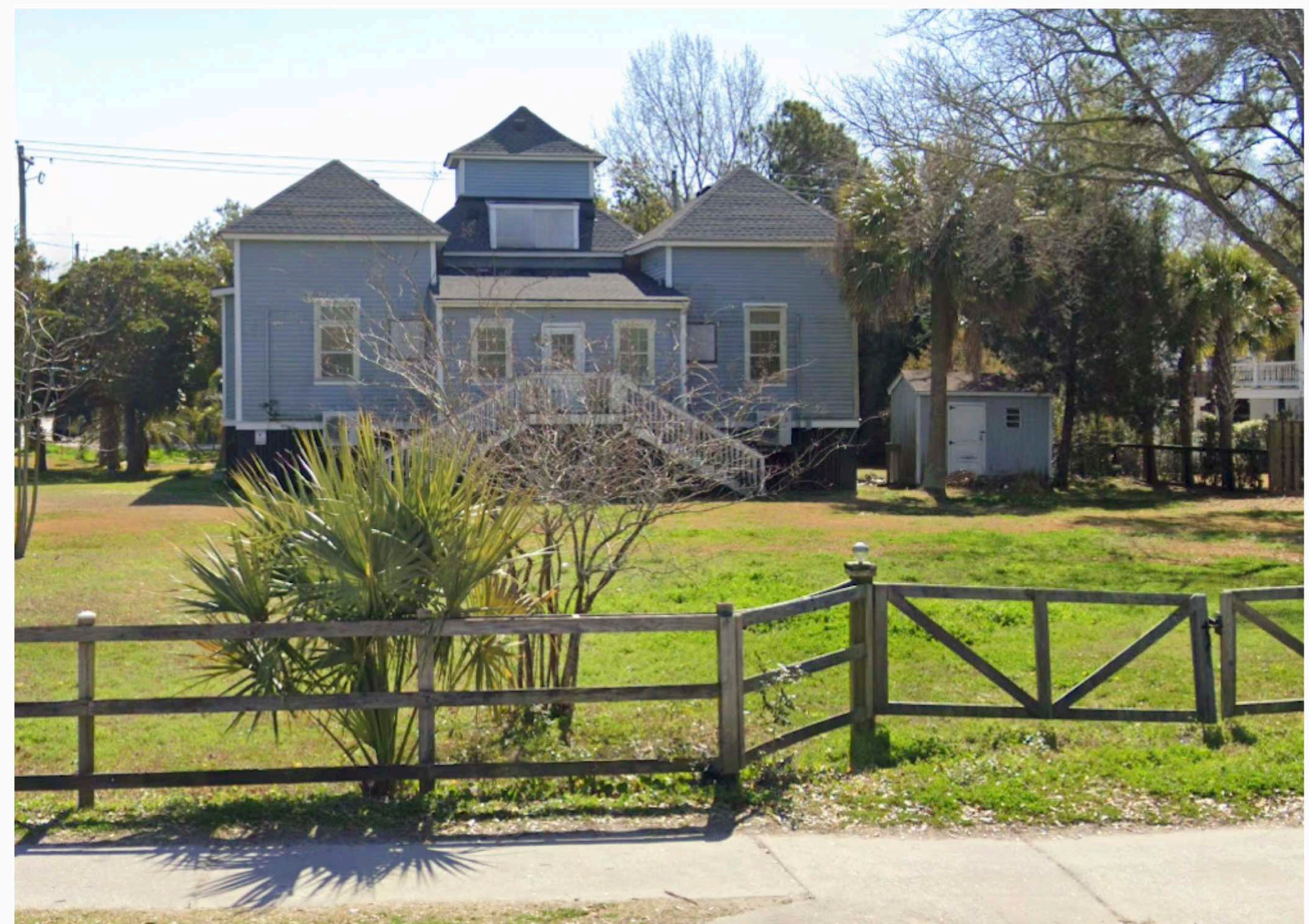
NORTH (MIDDLE STREET) VIEW
