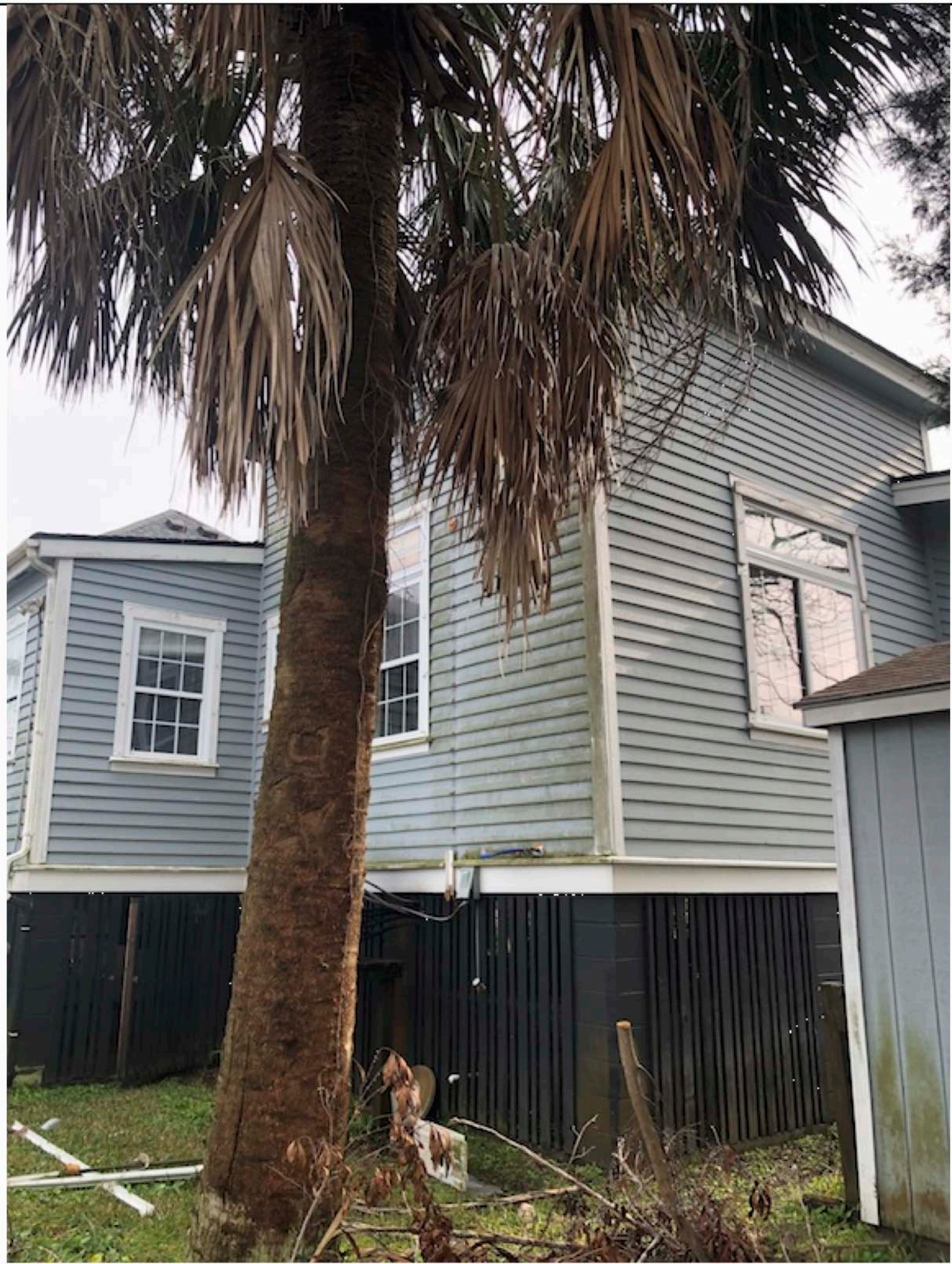
NORTH-WEST (REAR) VIEW
