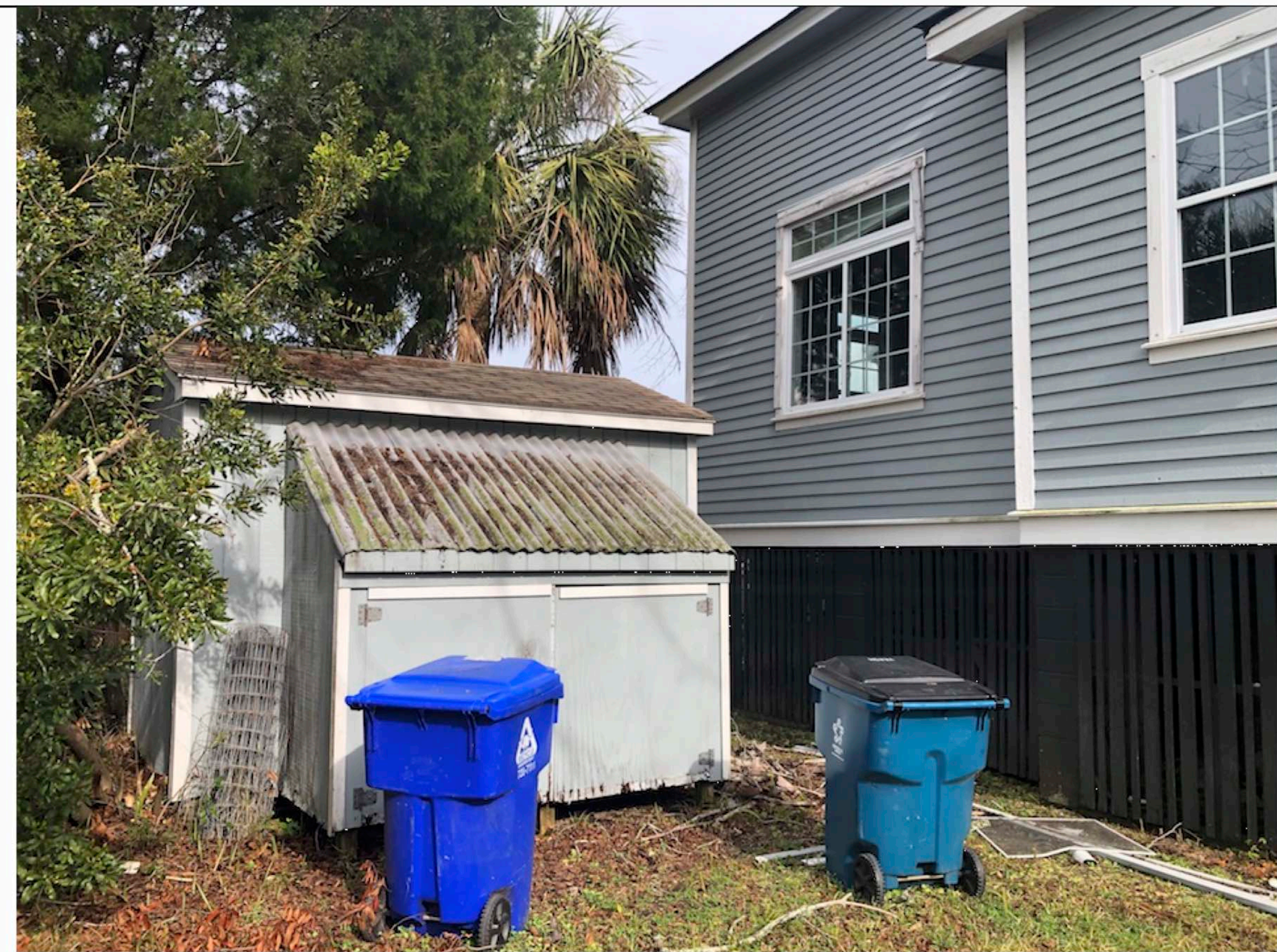
VIEW FROM ION AVENUE
