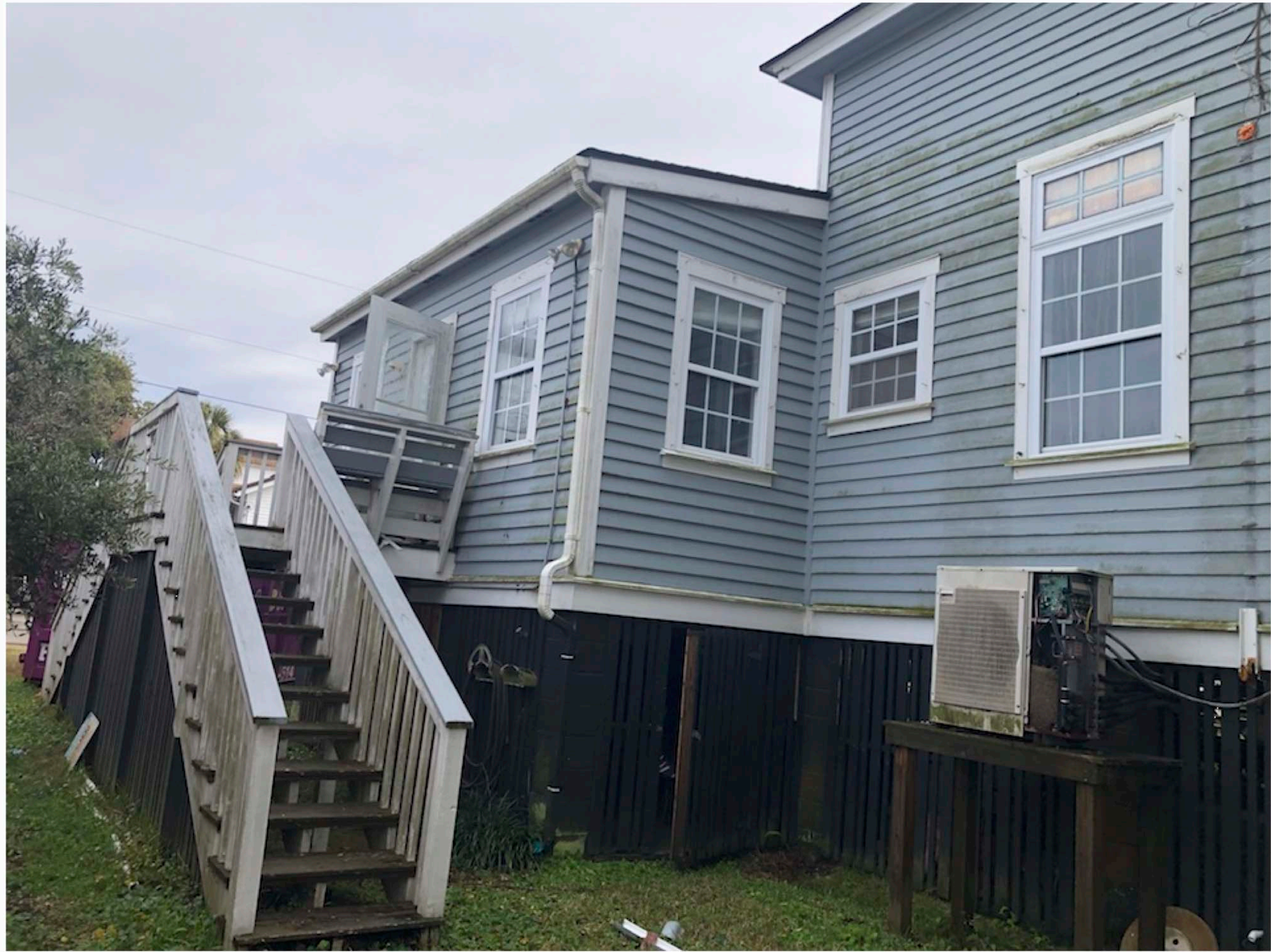
NORTH (REAR) VIEW
