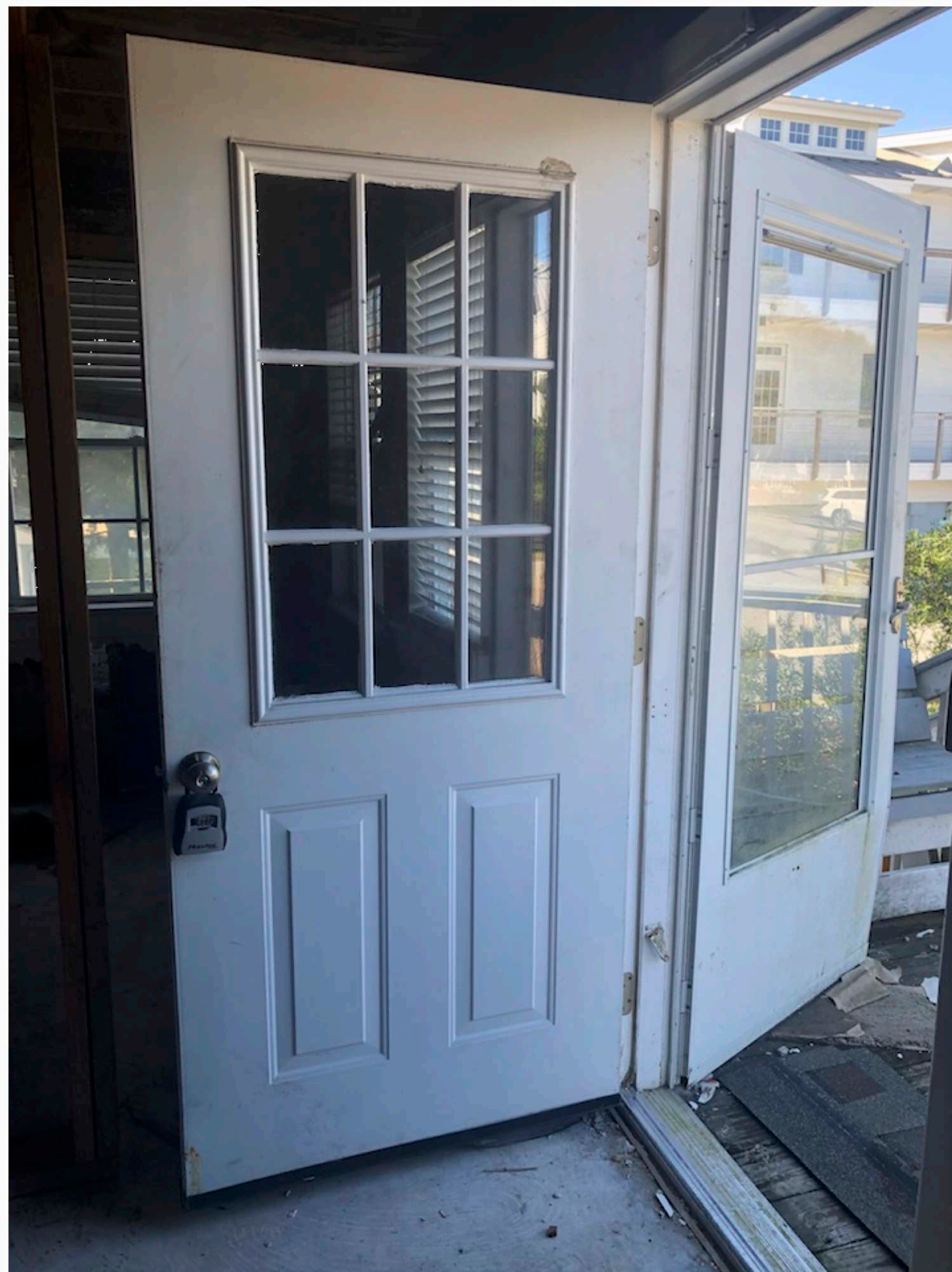
NONHISTORIC FIBERGLASS DOOR @ REAR (MIDDLE STREET)
