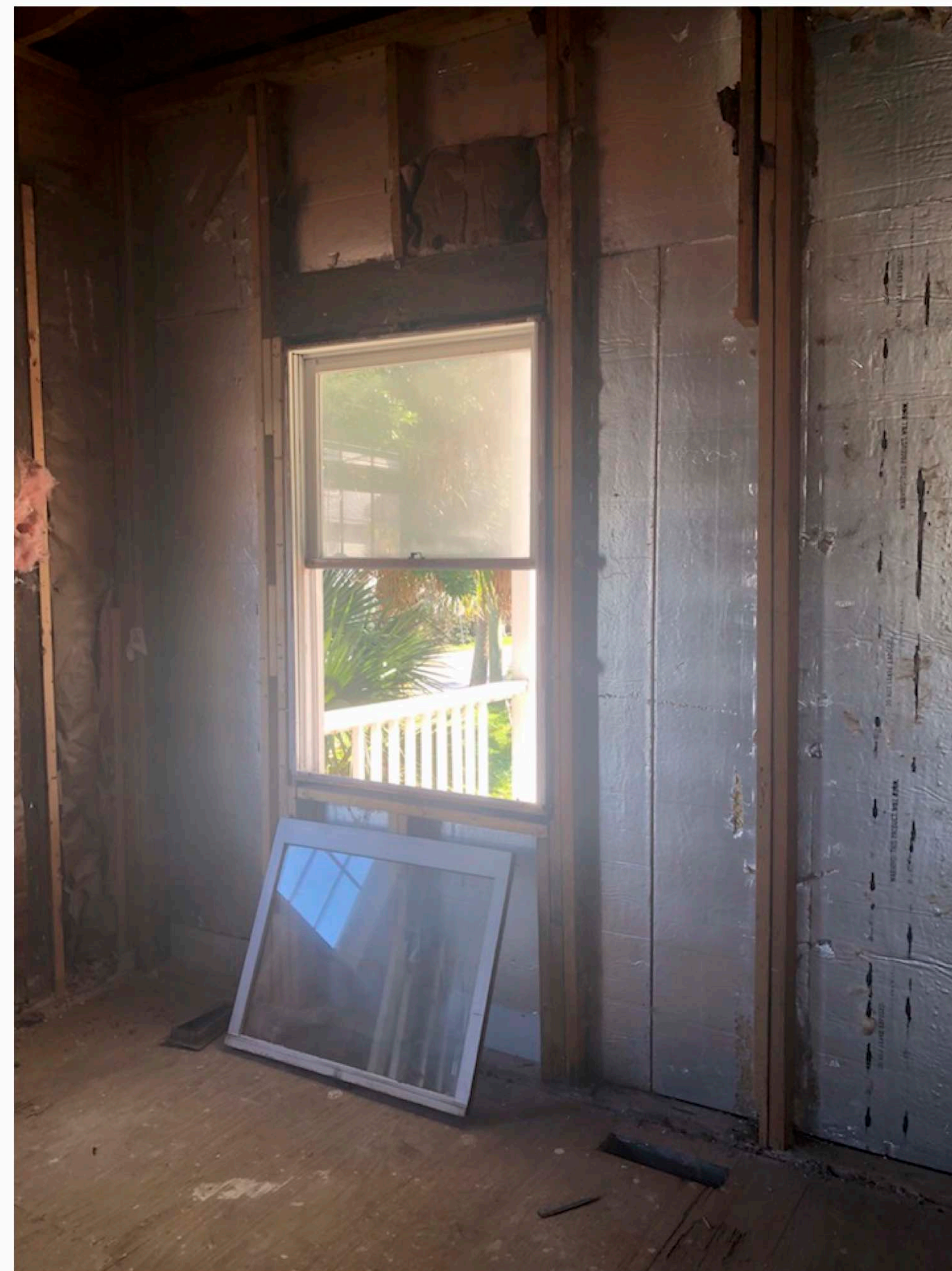
NONHISTORIC VINYL WINDOWS @ FRONT (ION AVENUE)
