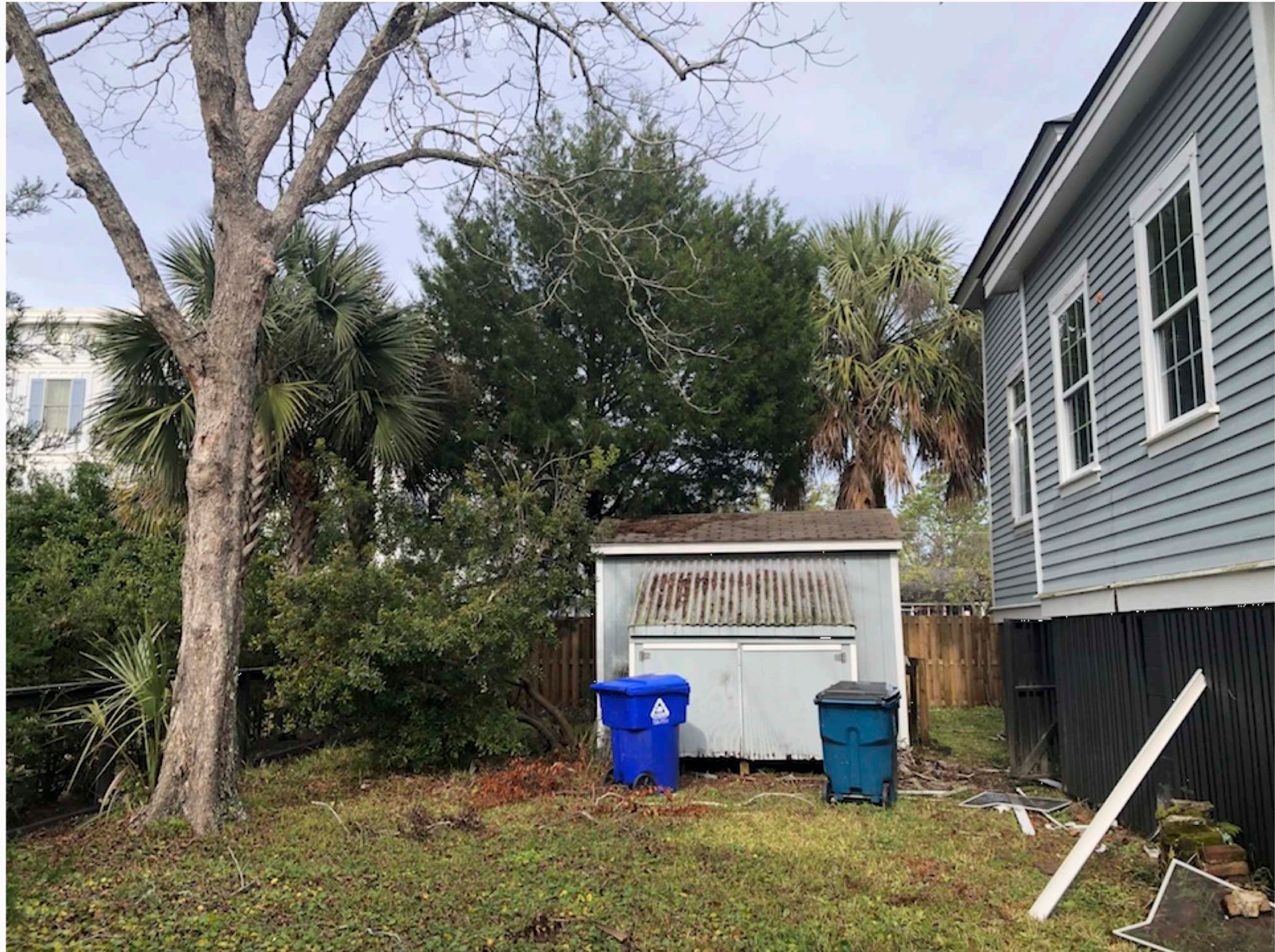
WEST (SIDE) VIEW
