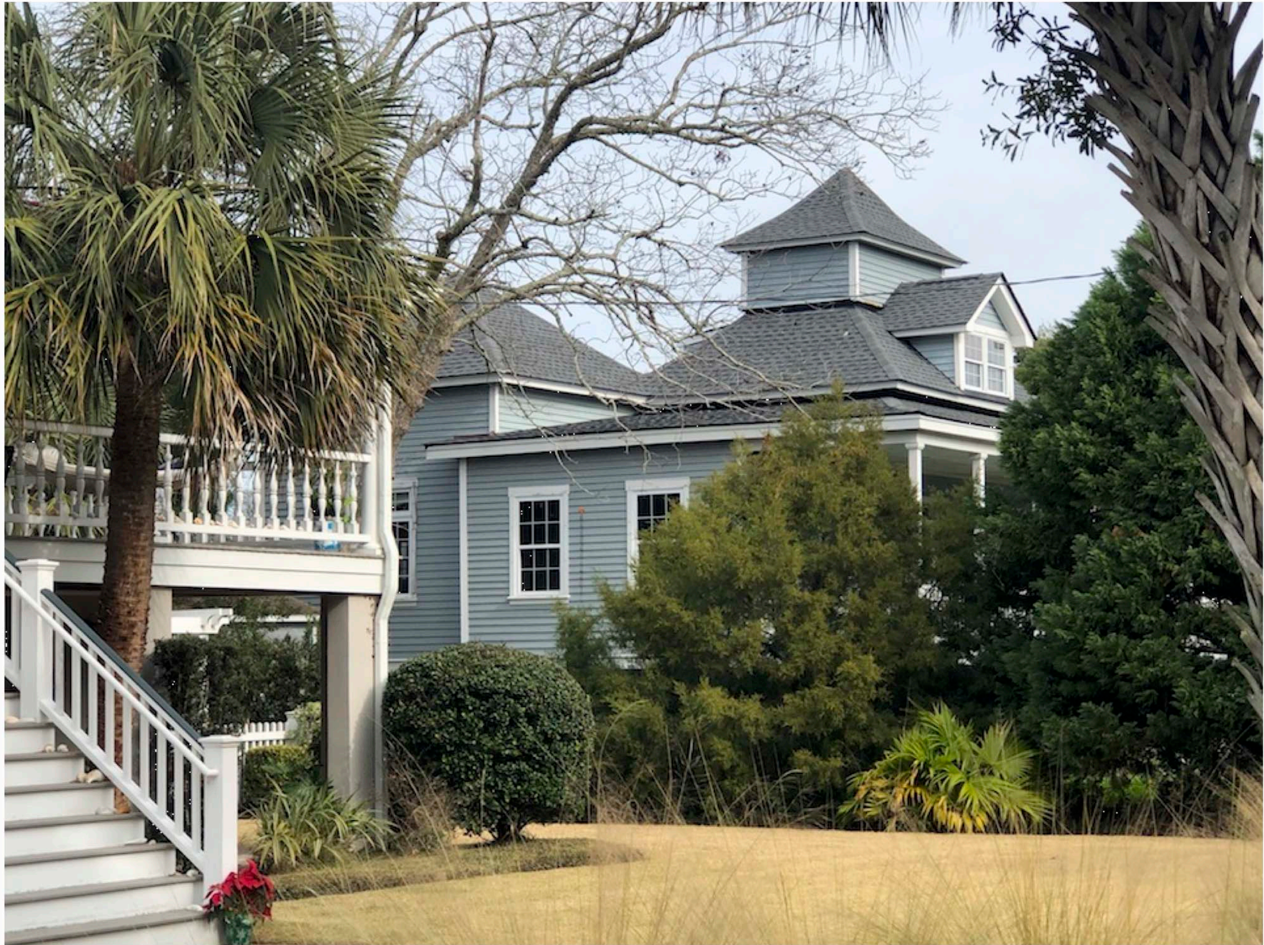
WEST (SIDE) VIEW
