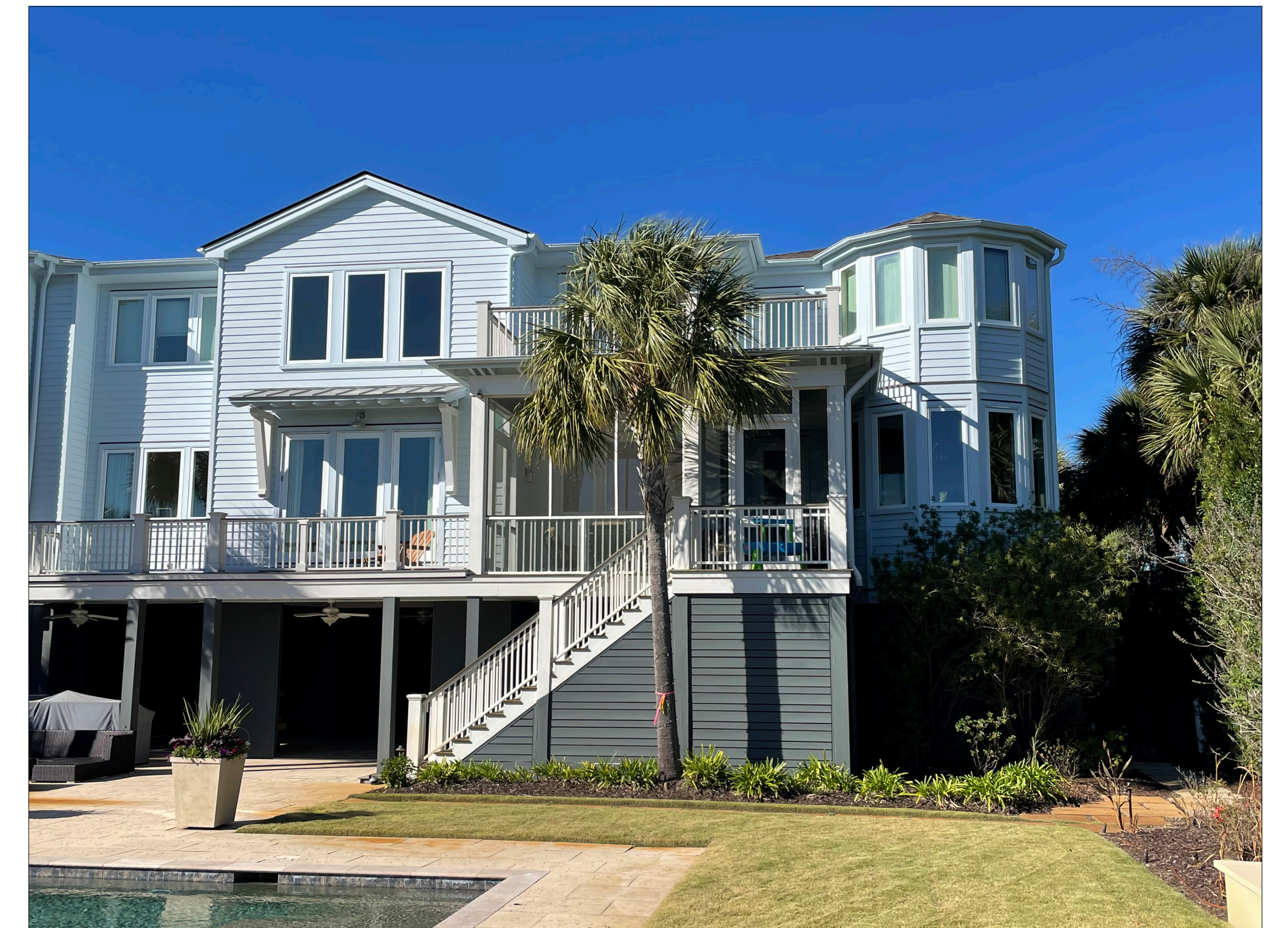
2623 BAYONNE AVE. DETAIL BACK PORCH AND BAY
