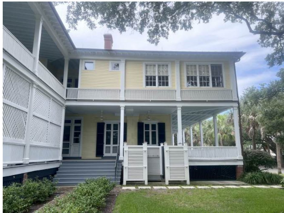
Existing Outdoor Shower, to be Removed
