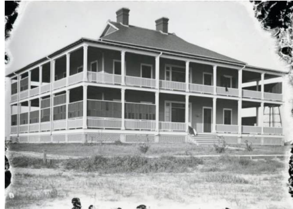
Photo showing Comdant's House (1989) https://www.charlestonmuseum.org/research/collection/sullivan-s-island-fort-moultrie-officers-quarters/86D089AC-4CB4-441C-9DDD-192522015165
