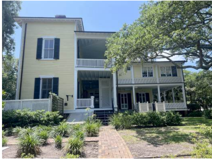
1702 I'On Avenue, North elevation
