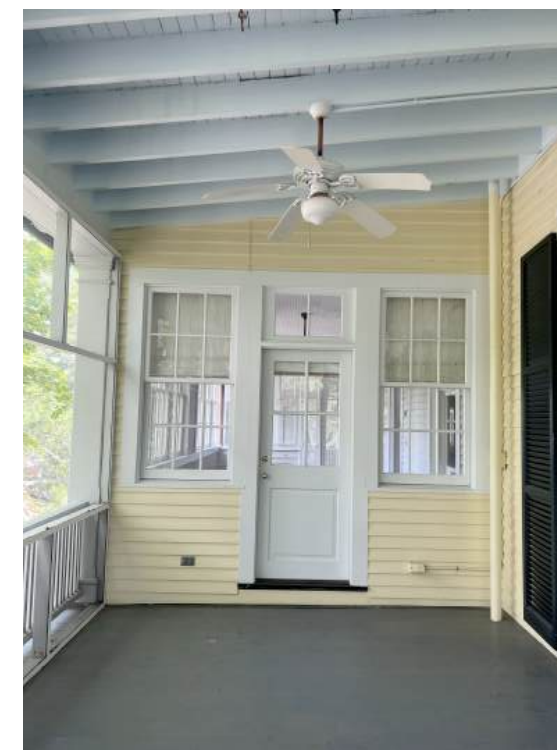
SW Screened Porch looking towards Enclosed Porch- 2nd Floor
