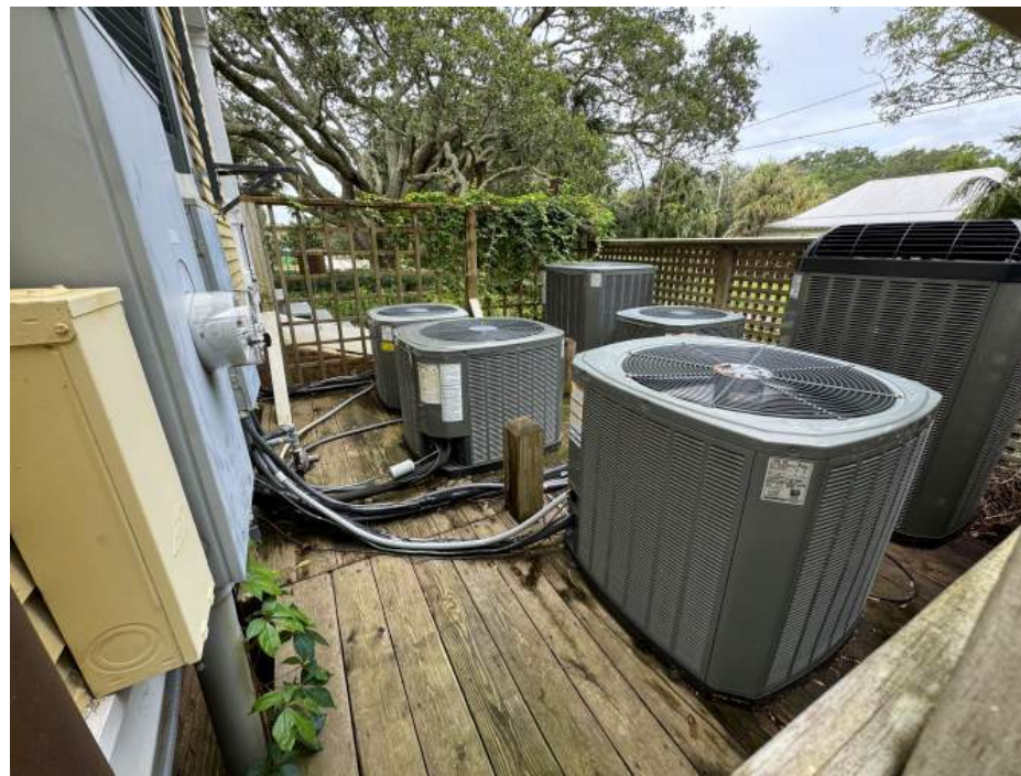
Existing HVAC Units, Deck, and Screen to be Removed and Replaced
