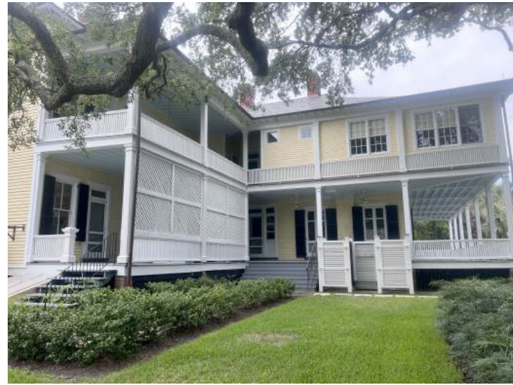
1702 I'On Avenue, North and West elevation
