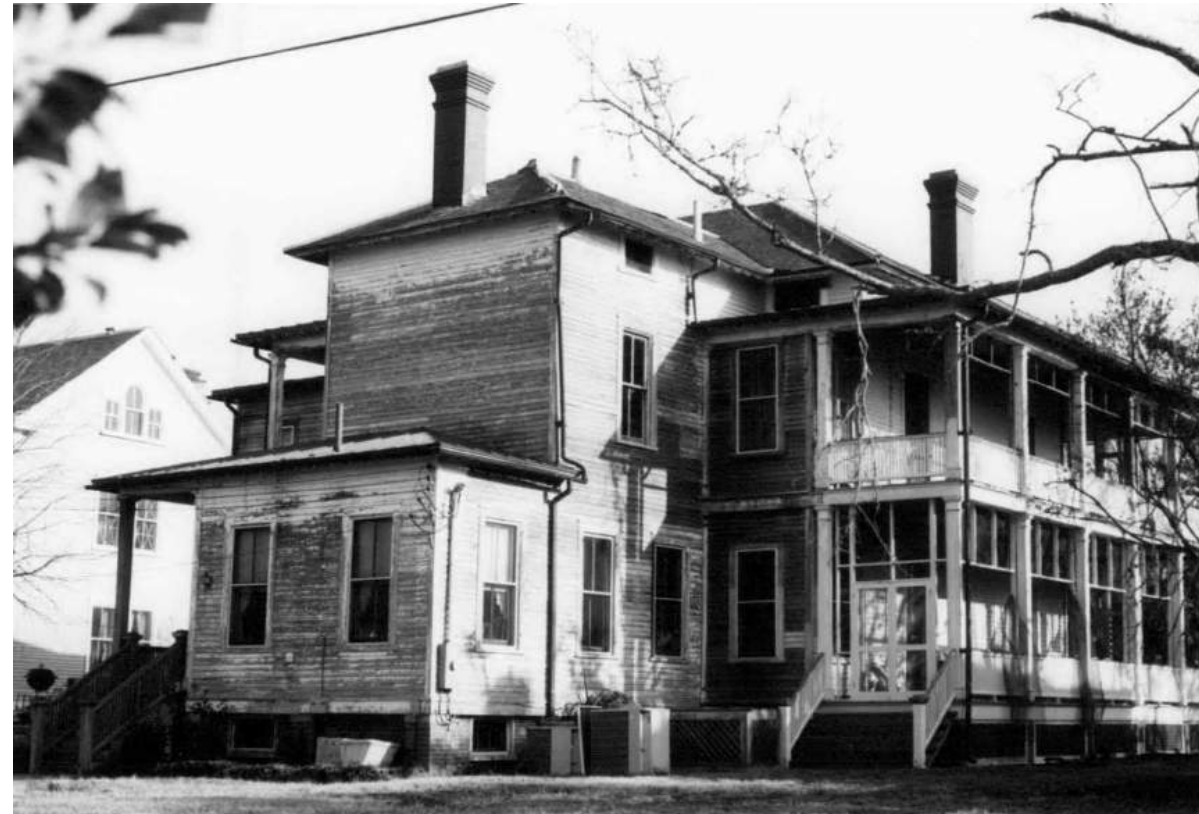
Similar configuration at 1760 I'On Avenue, Seen from the Back Yard - January 18, 1990
