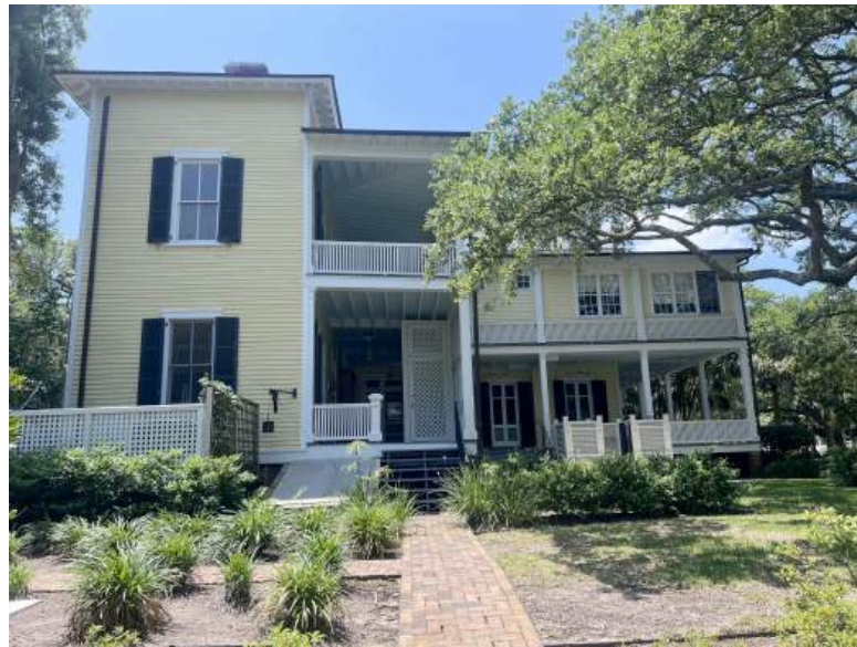
1702 I'On Avenue, North elevation
