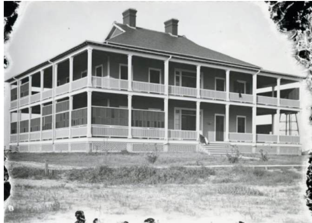
Photo showing Commandant's House (1989) https://www.charlestonmuseum.org/research/collection/sullivan-s-island-fort-moultrie-officers-quarters/86D089AC-4CB4-441C-9DDD-192522015165
