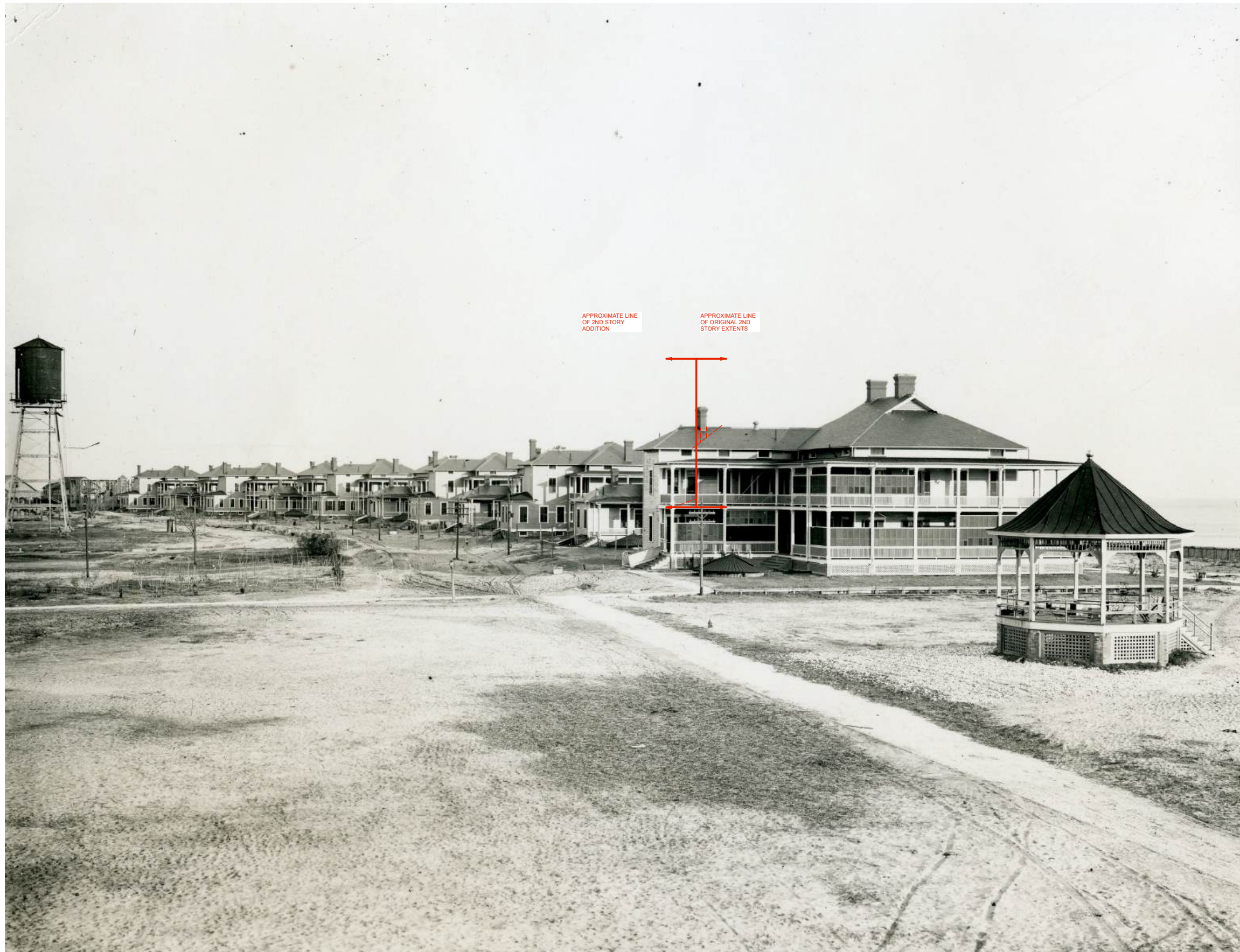
HISTORIC PHOTO DEMONSTRATING SIMILAR 2ND FLOOR CONFIGURATION AT ADJACENT OFFICER'S UNITS
