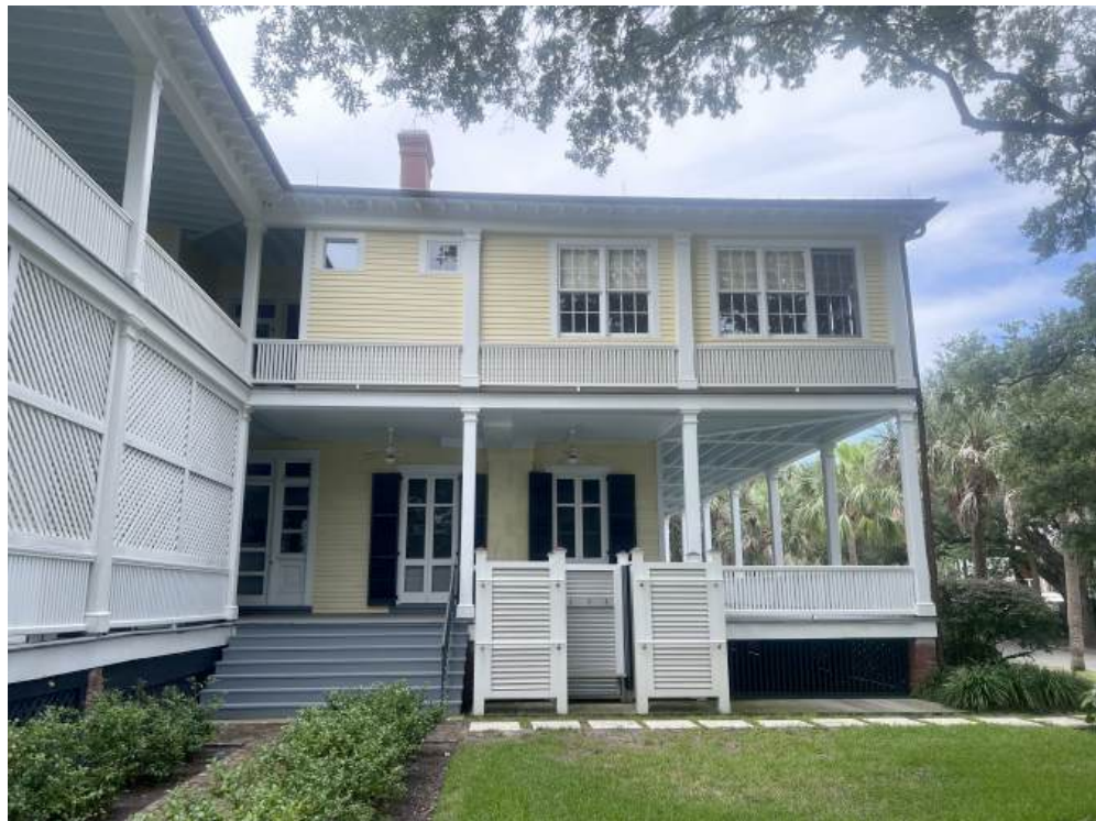
Existing Outdoor Shower, to be Removed
