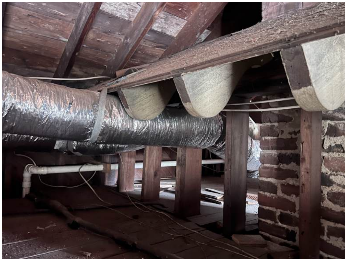
Original 2nd floor roof framing as remaining in existing attic
