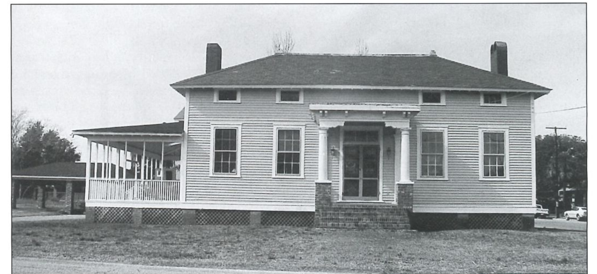
1617 MIDDLE STREET C. 1900. The Fort Moultrie Dispensary/Provost Marshall's Office was constructed as the dispensary for Fort Moultrie and is so indicated on 1901 and 1915 maps. It was later converted for use as the Provost Marshall's Office, and has since been converted to a residence. [Part of a significant grouping of military structures.] (Courtesy Marshall Stith.)
