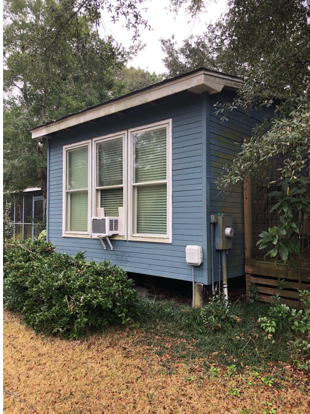
Rear wall of the bedroom addition.
