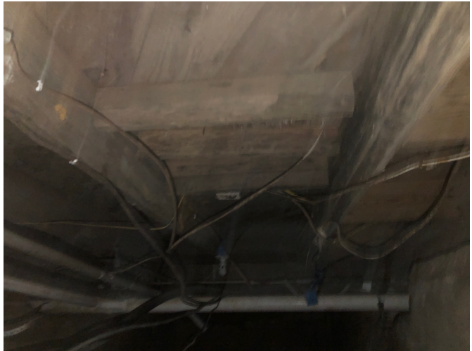
Left: modern plywood and circa 1970s linoleum flooring in the ell bay, which is now an office and pantry. Right: the framing and diagonal sheathing of the ell bay, photographed from a vent on the western elevation.
