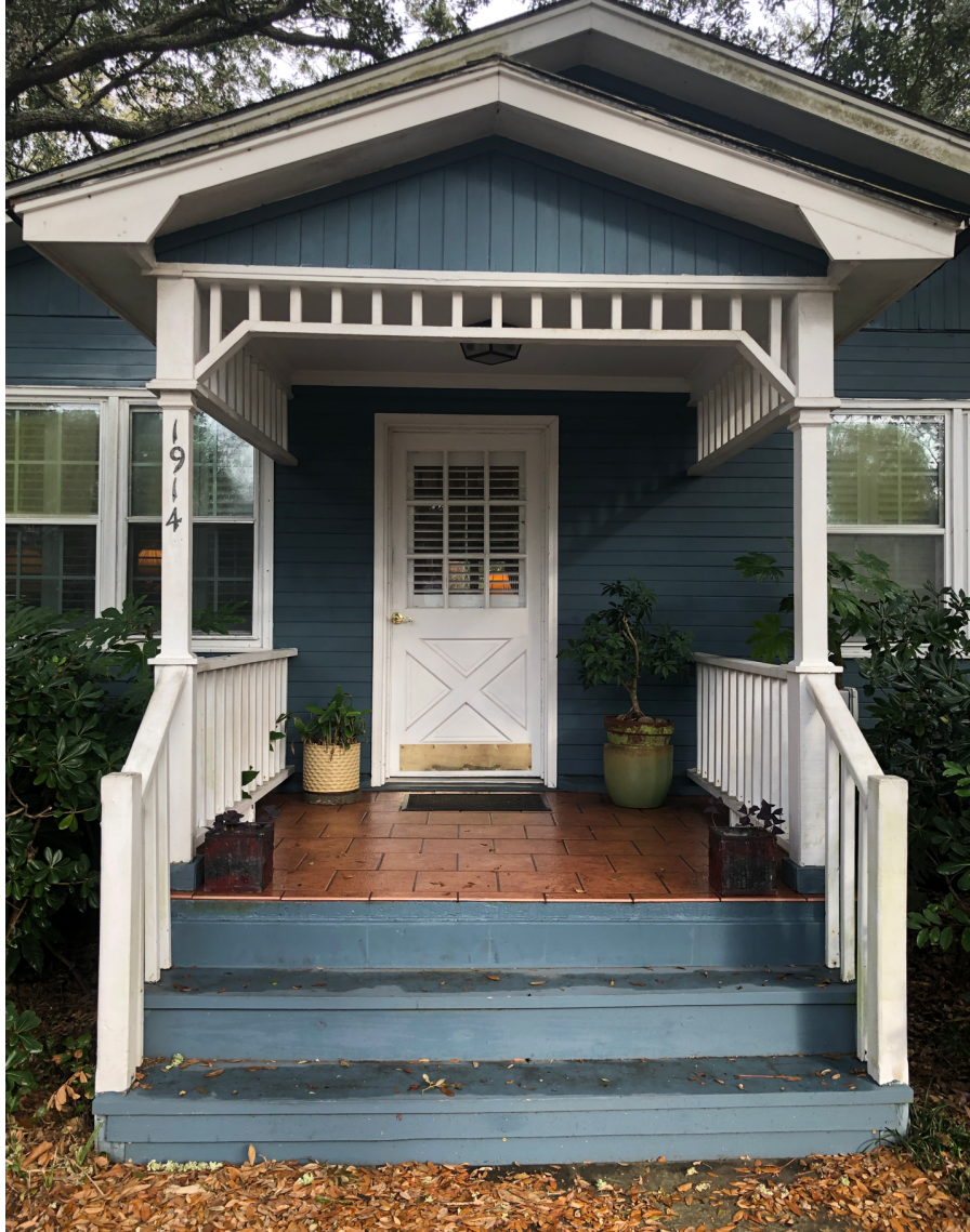
Front porch, which replaced an earlier shed roofed porch that extended along the entire façade.
