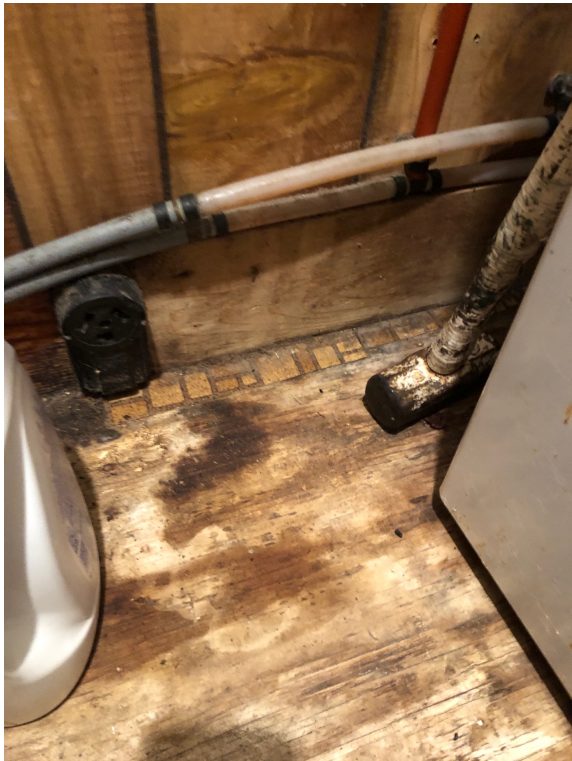
Left: modern plywood and circa 1970s linoleum flooring in the ell bay, which is now an office and pantry. Right: the framing and diagonal sheathing of the ell bay, photographed from a vent on the western elevation.
