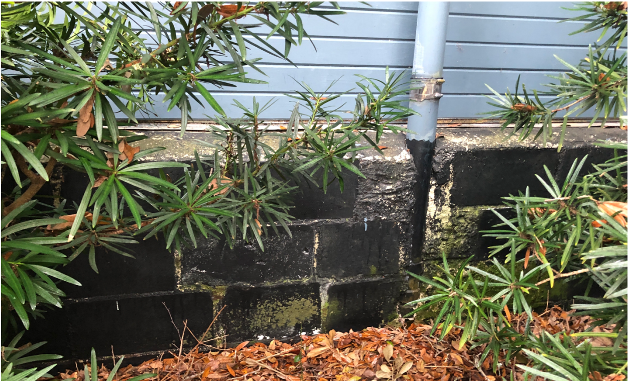
Close up of the painted cinderblock foundation skirting that runs continuously around the portions of the house that predate 1992.
