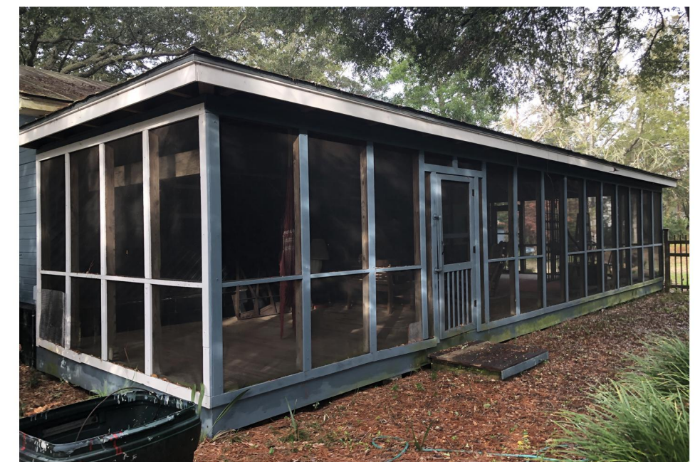
Perspective views of the wrap around side screened porch, which is framed with treated dimensional lumber.
