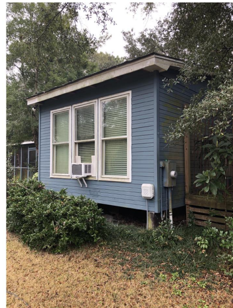
Rear wall of the bedroom addition.
