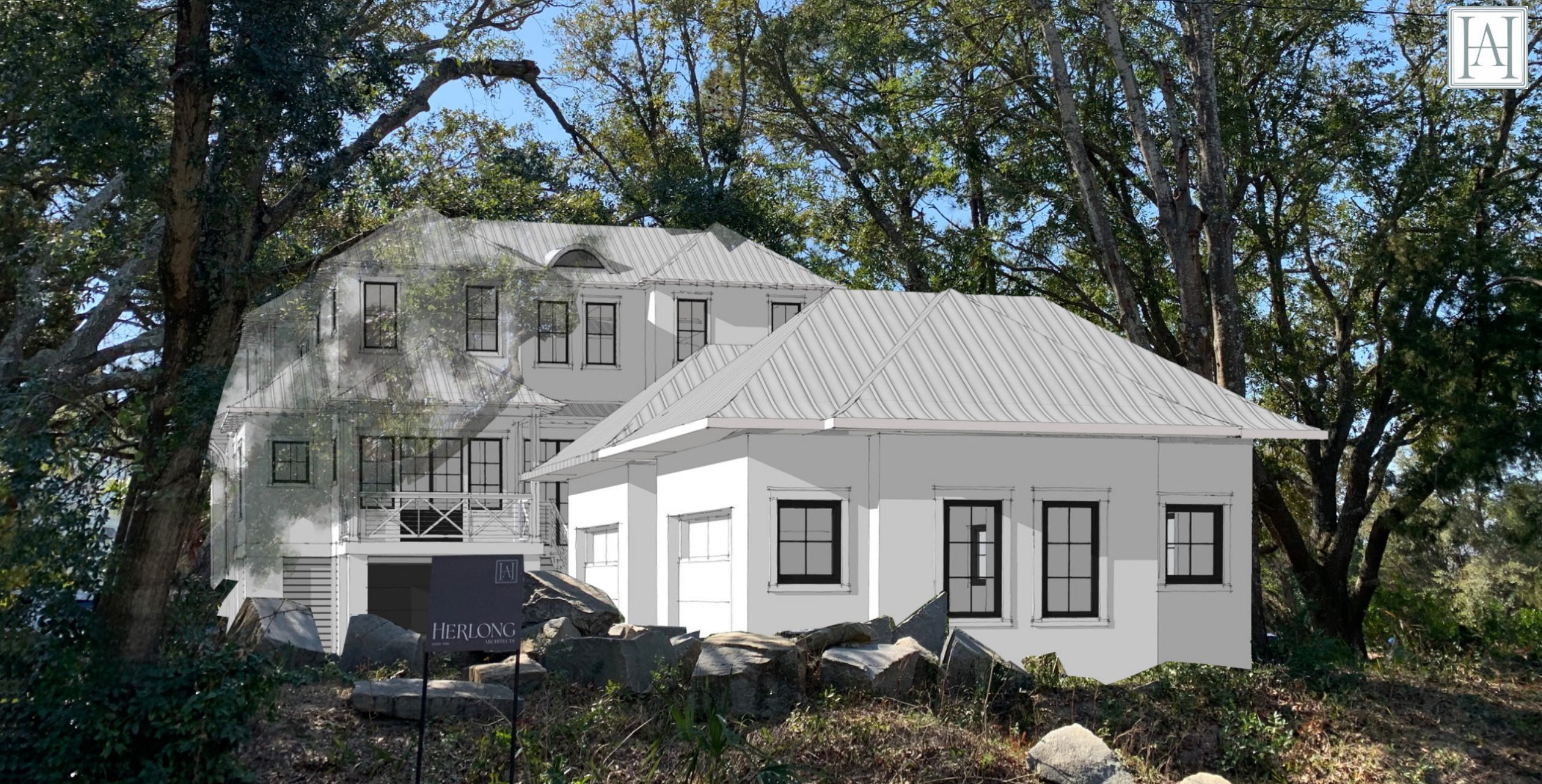
North East View from Atlantic Avenue
