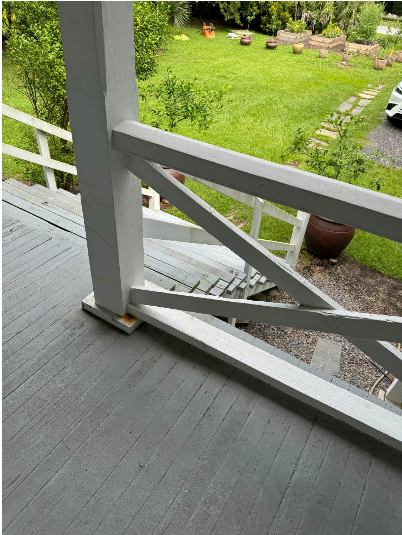
PHOTO - (REAR PORCH, RAILING DETAIL, JULY 19, 2024)
