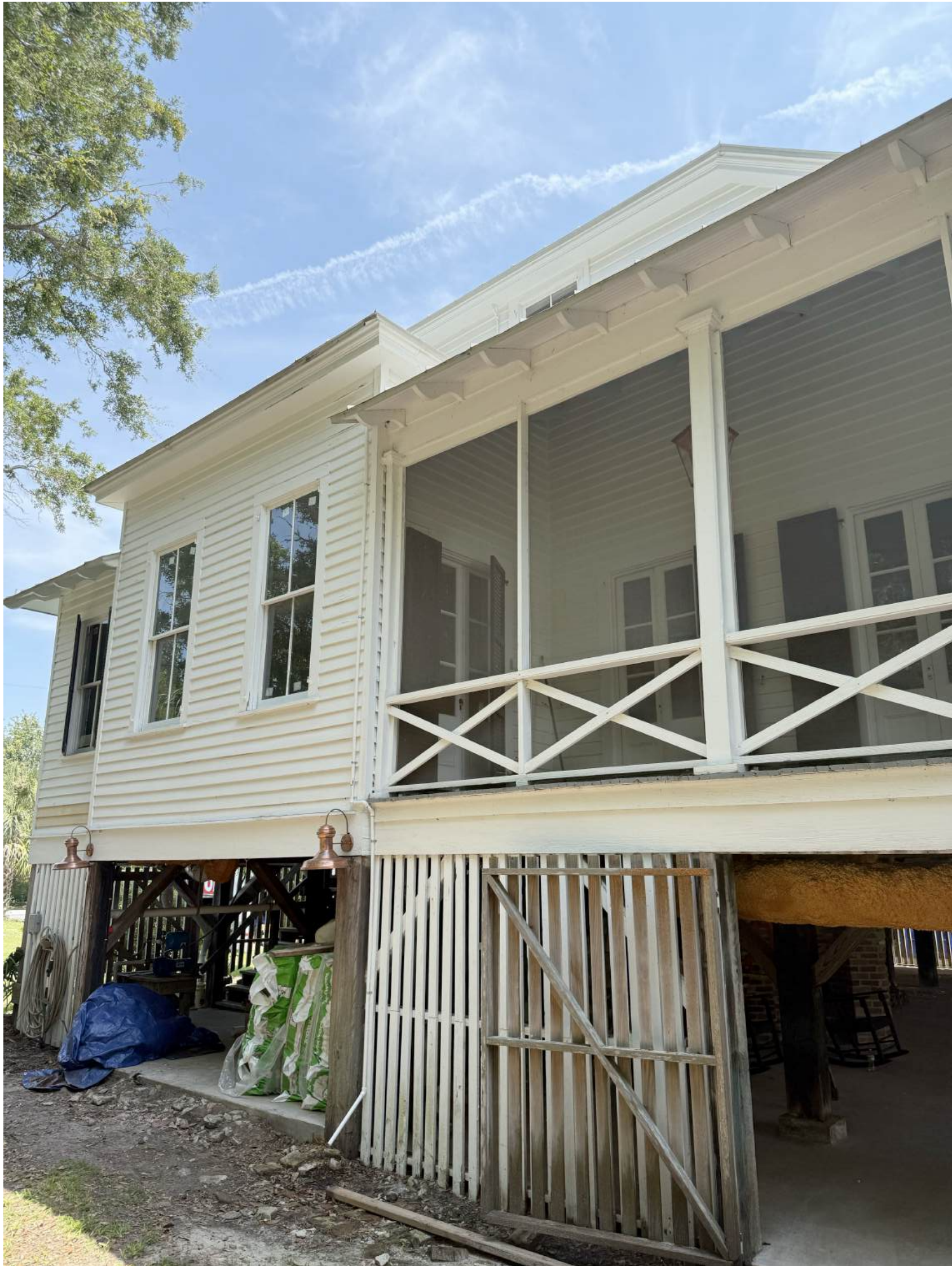
PHOTO - (WEST SIDE, JUNE 25, 2025)
