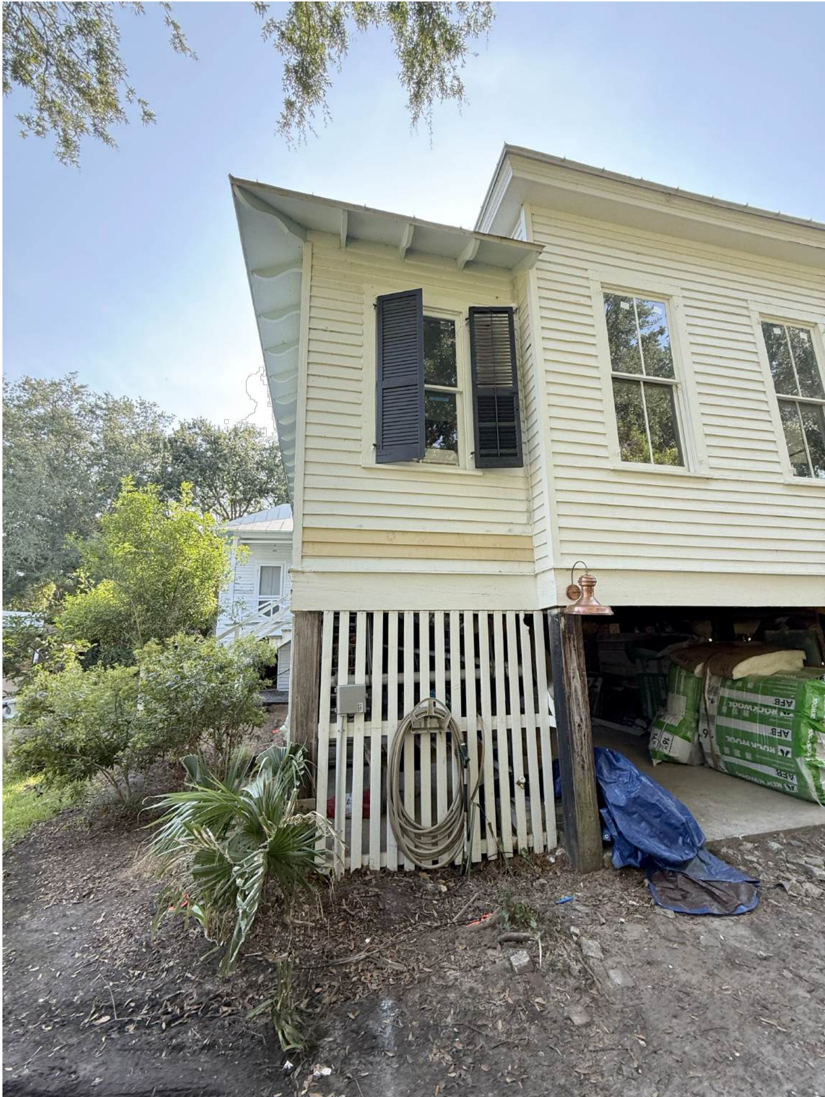
PHOTO - (WEST SIDE, JUNE 25, 2025)
