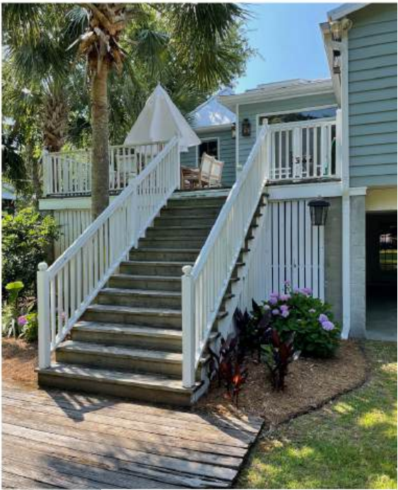
PHOTOS OF EXISTING CONDITIONS
