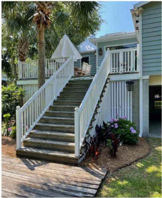
PHOTOS OF EXISTING CONDITIONS
