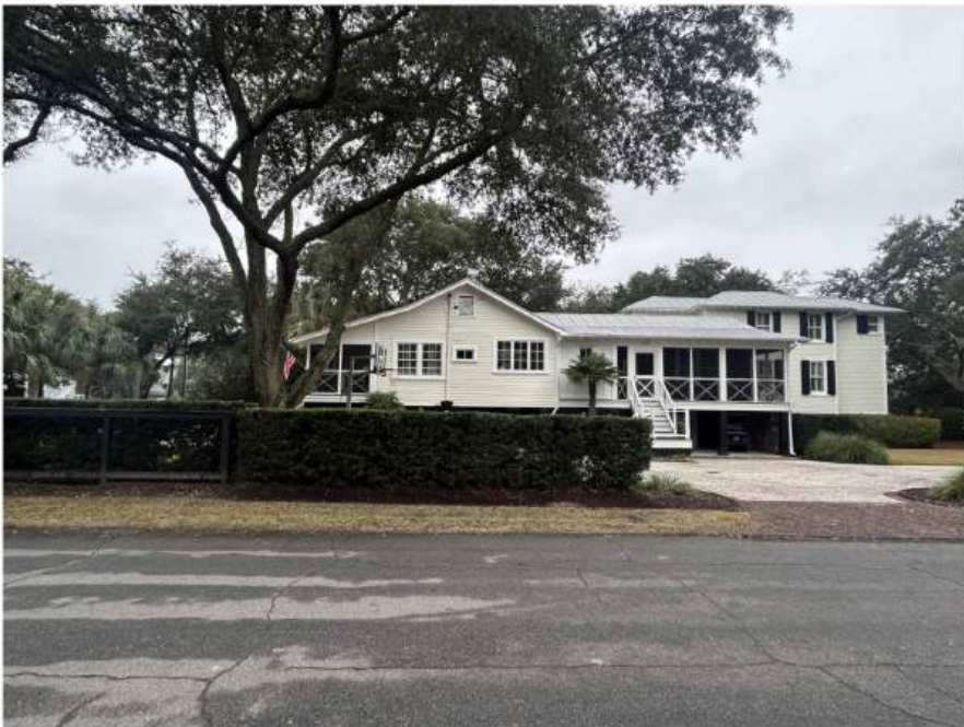
2730 Brooks Street - Existing View from Station 28 Street
