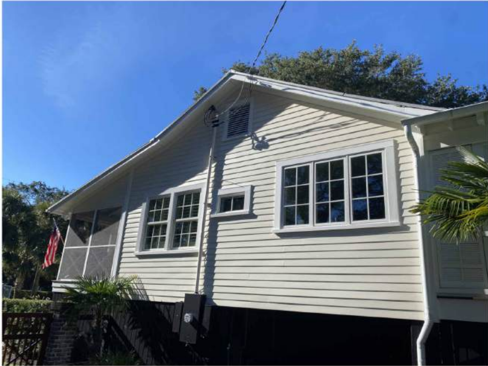
2730 Brooks Street Historic Structure East Facade
