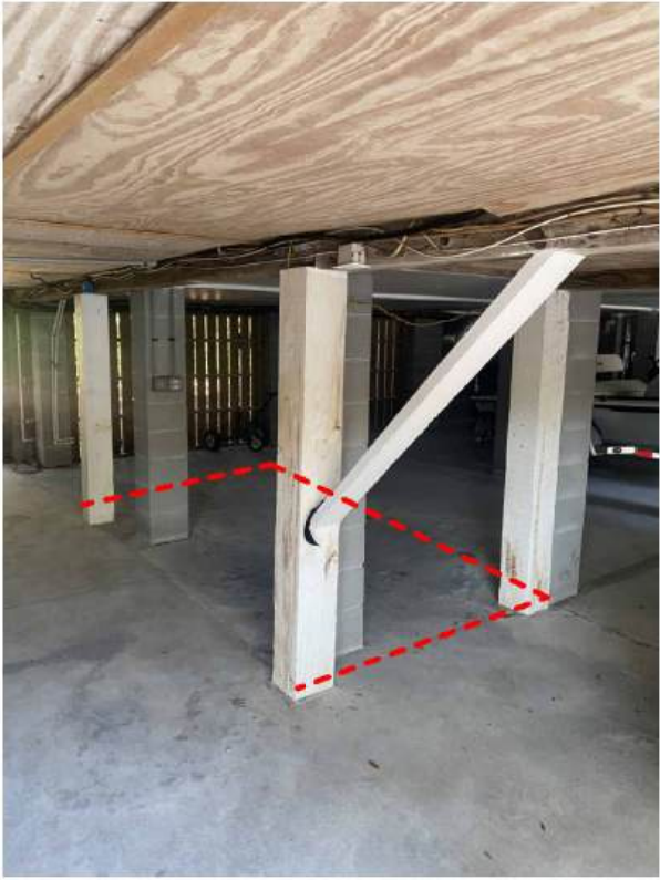
Timber posts below existing structure - indicative of original footprint.
