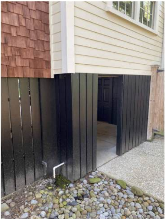
2730 Brooks Street Existing Foundation Screening
