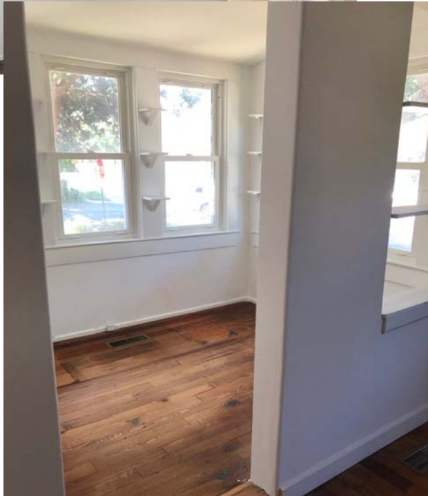
The enclosed front sitting room in part of the enclosed former front porch (bay 8). The threshold marks the original front wall of the house.
