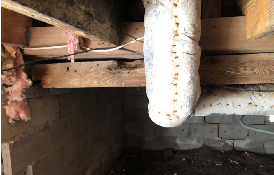
Looking south, there is a CMU block foundation wall that helps support a joist span.
