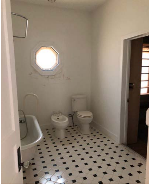
Standing the bathroom facing into the passageway; view of the bathroom from the shelved/back section of the living room, with a historic clawfoot tub.
