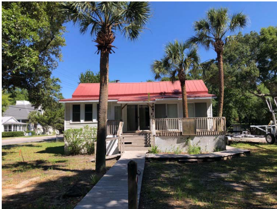
Facade with enclosed porch.
