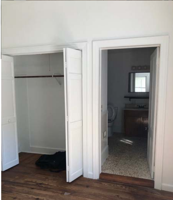
A third bedroom is located off of the living room, to the right. The bedroom is located in bay 1 of the original house. The closet and bathroom are in addition bay 3. Note the historic flooring in the bathroom, and the large threshold to the bathroom where the original back wall of the cottage was located.
