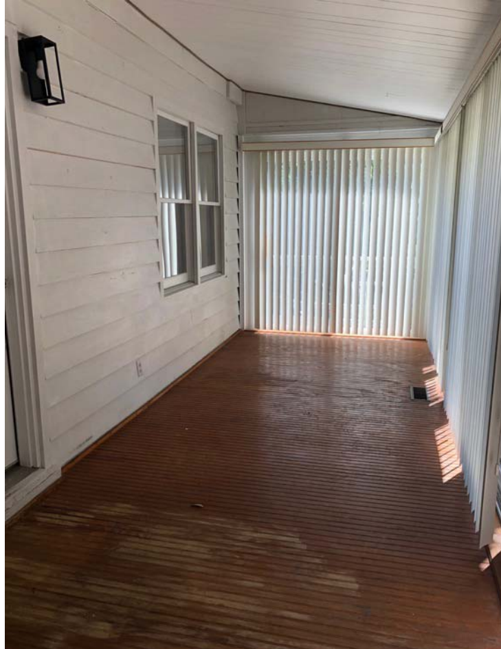
The enclosed front porch, facing west.
