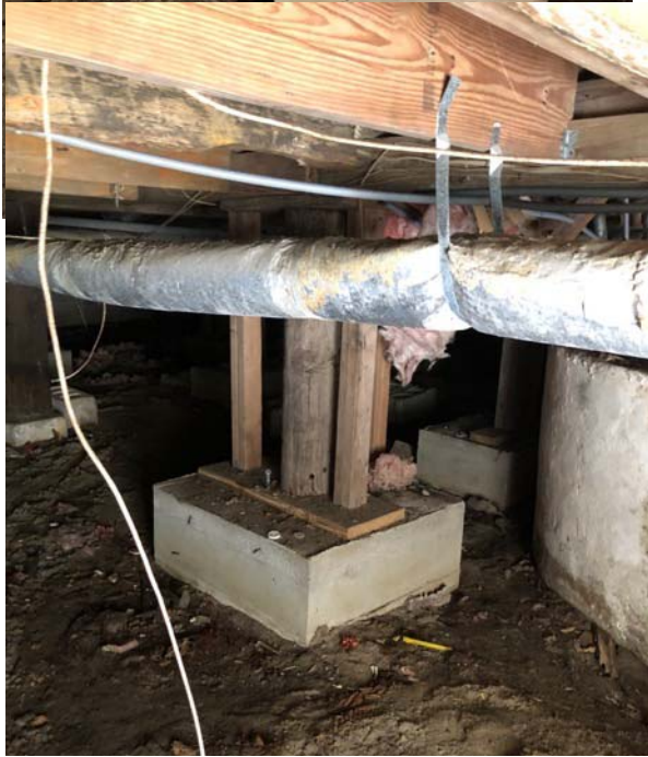
The cistern, foundation, and floor sheathing below bay 3.
