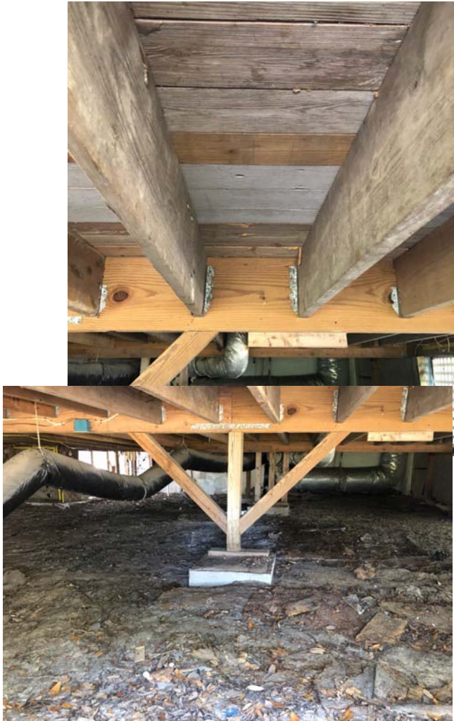
Bay 5: Western rear shed-roofed addition (present by 1971)
