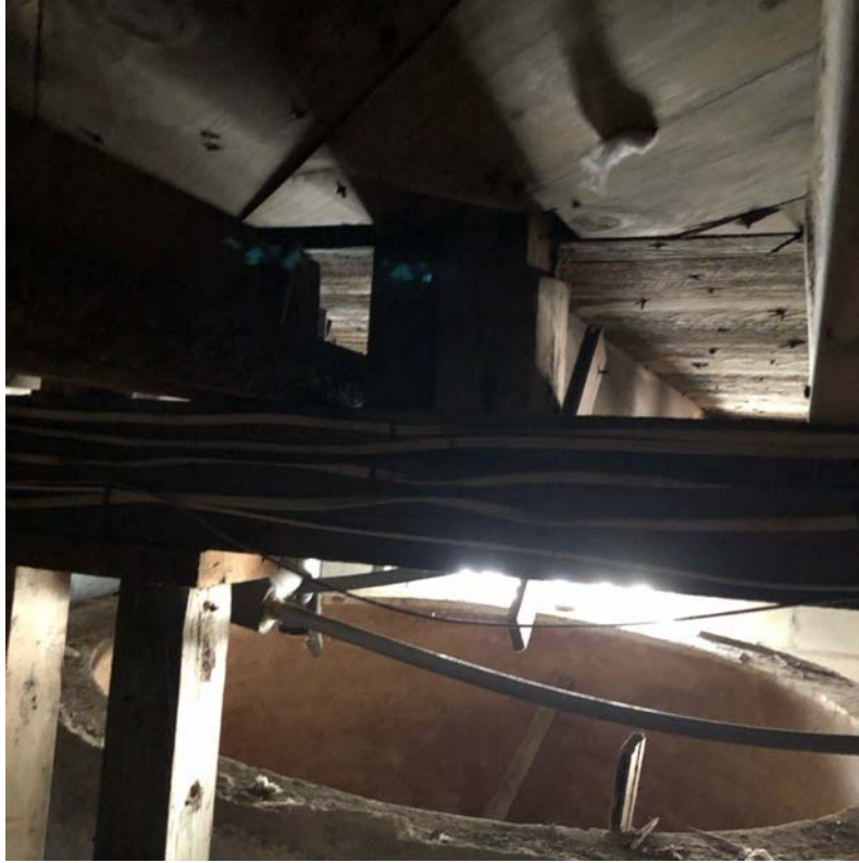
The diagonal sheathing in bay 4, looking west to bay 3's cistern.
