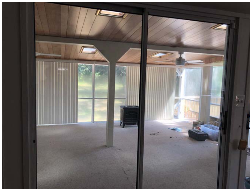
Addition bay 7, the enclosed back porch, present by 1994.
