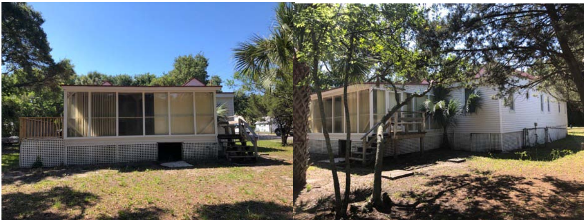
Rear/north elevation of the house with enclosed back porch.
