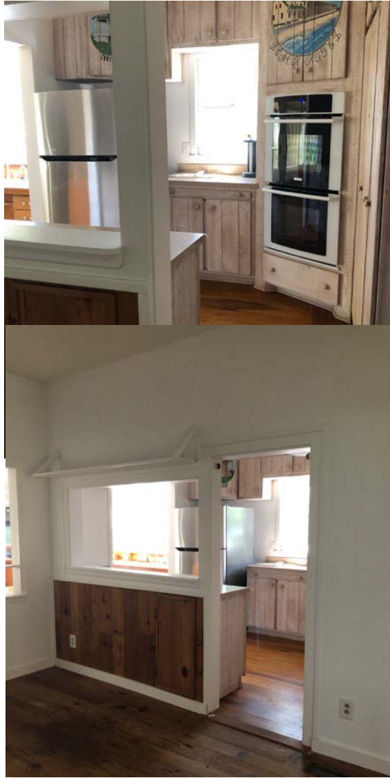
The kitchen (addition bay 3) viewed from the living room. There is no historic material in bay 3, which holds a modern kitchen and bathroom. The former exterior wall was altered with an unglazed opening sometime after the central shed-roofed bay 4 was added.
