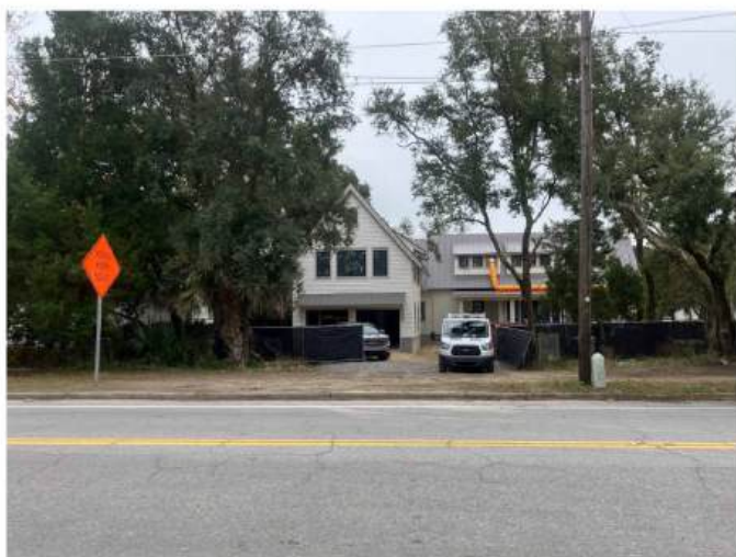
2802 Brooks Street (Under Construction) - Existing View from Jasper Boulevard
