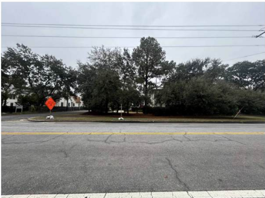
2730 Brooks Street - Existing View from Jasper Boulevard
