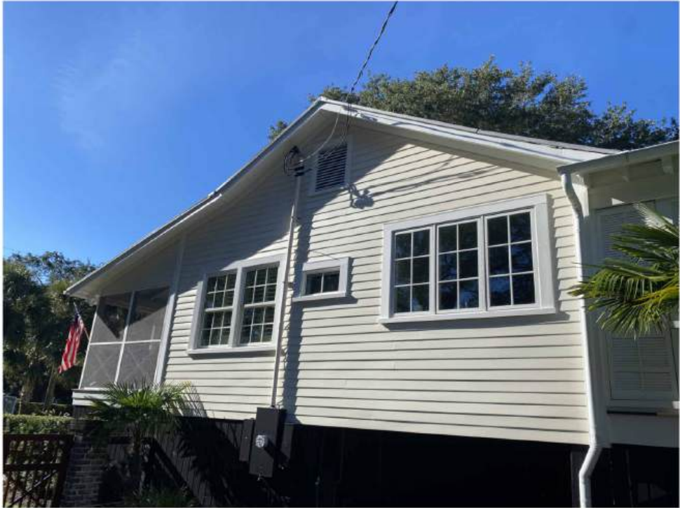
2730 Brooks Street Historic Structure East Facade
