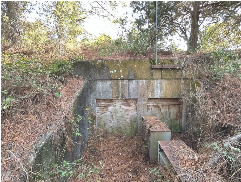
HISTORIC BUNKER HVAC OPENING ON ION AVENUE
