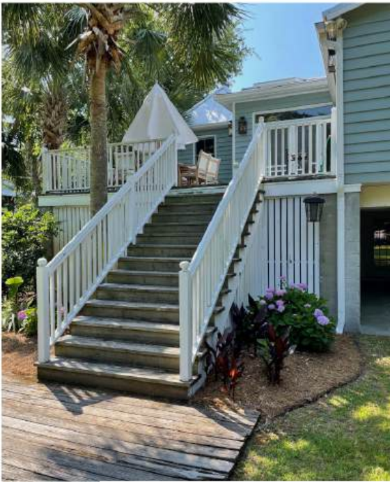
PHOTOS OF EXISTING CONDITIONS
