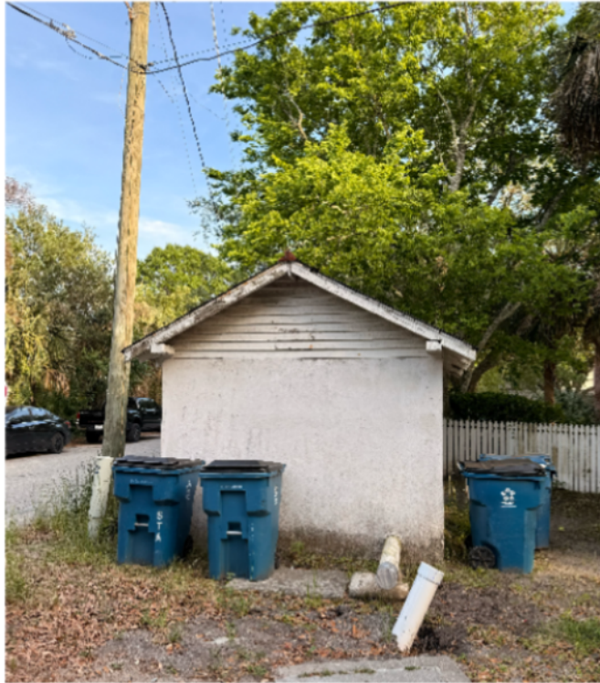
PUMP HOUSE @ CORNER
