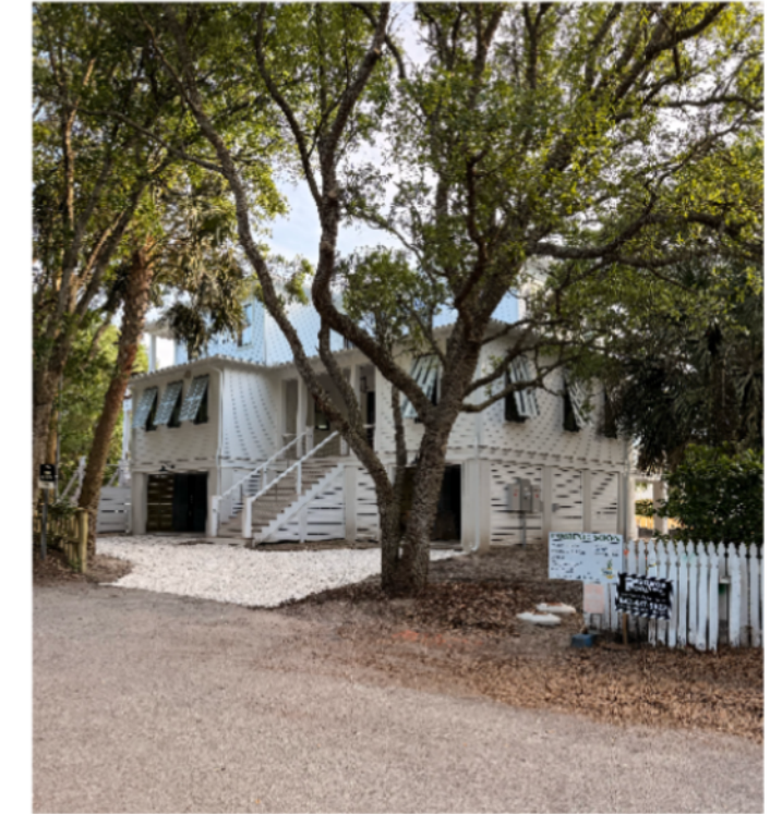
NEW HOUSE @ END OF 18
