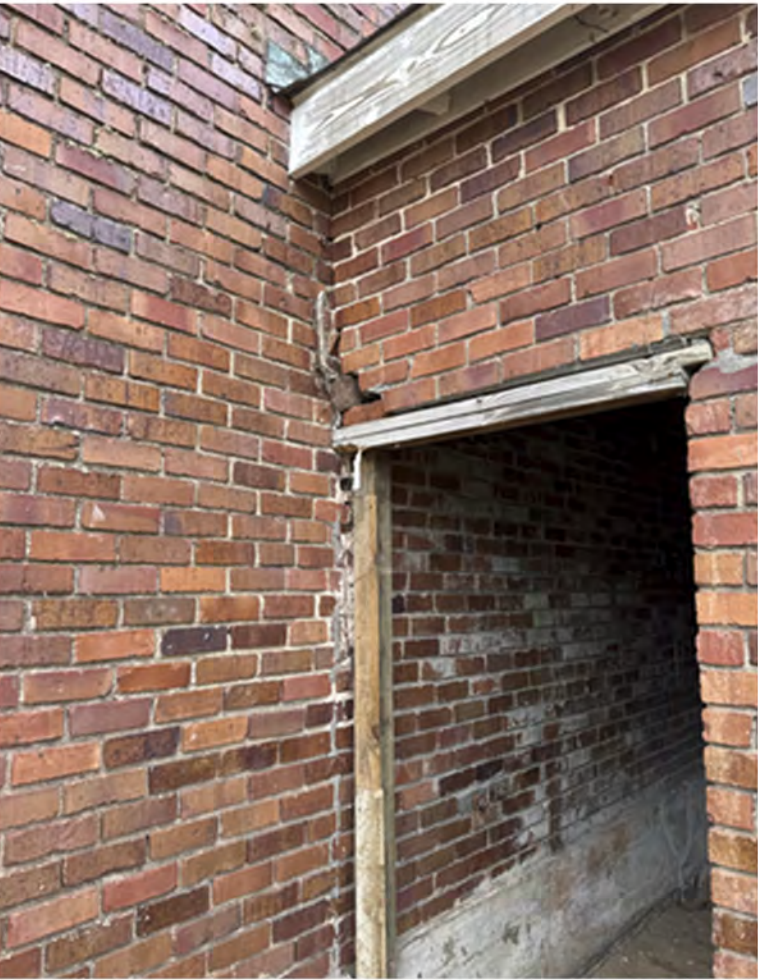
Minimally supported brick at openings and no structural attachment to main structure.
