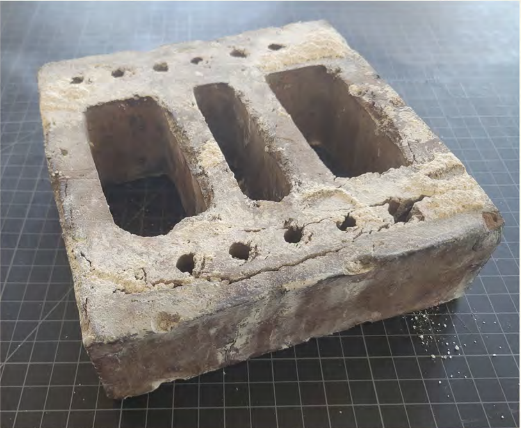
EXISTING BRICK UNIT
