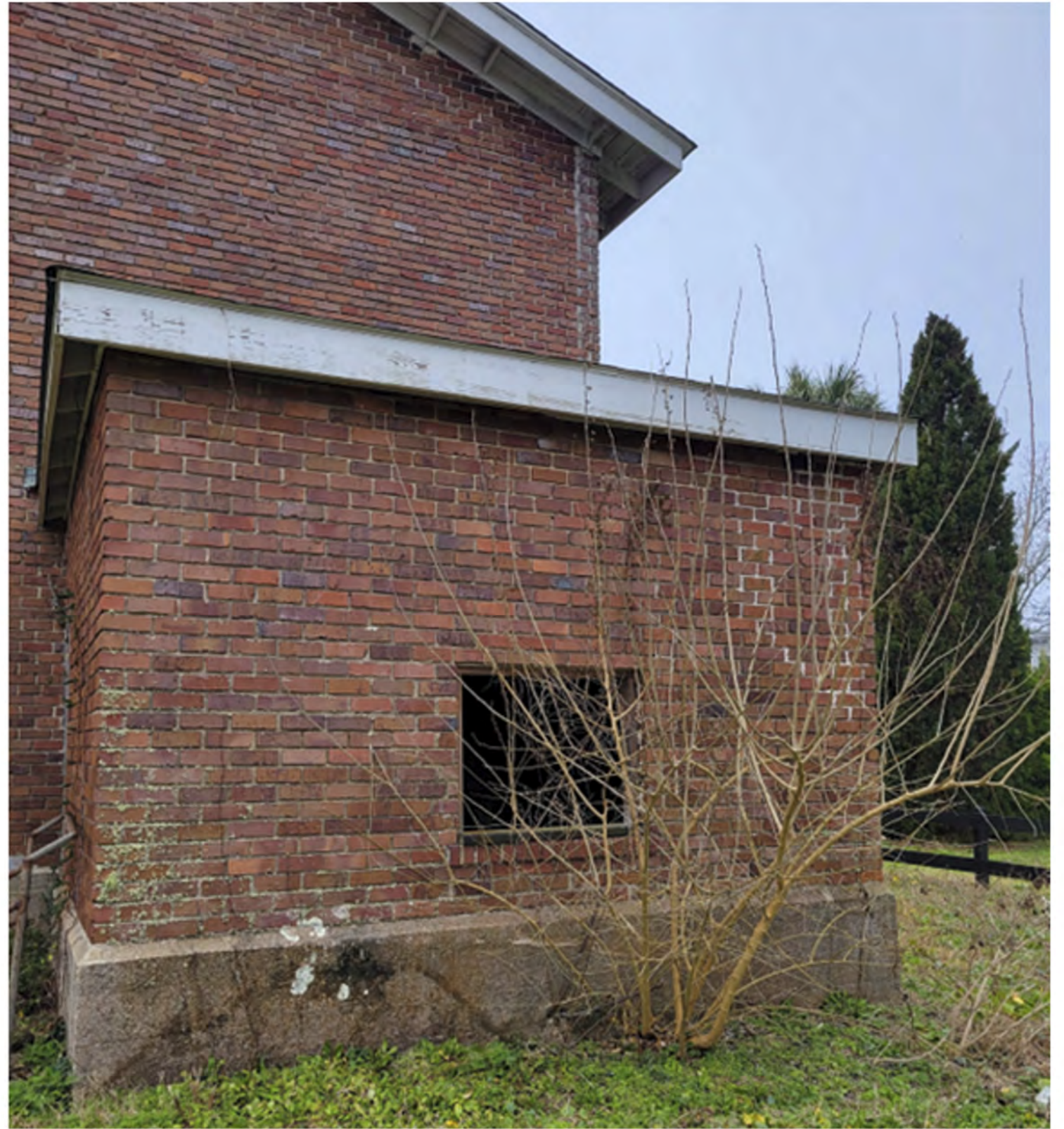
Every facade exhibits multiple stair-step cracks and foundation cracking. Openings were not properly supported, causing additional damage, and there is evidence of multiple attempts to repair the facades over the years.
