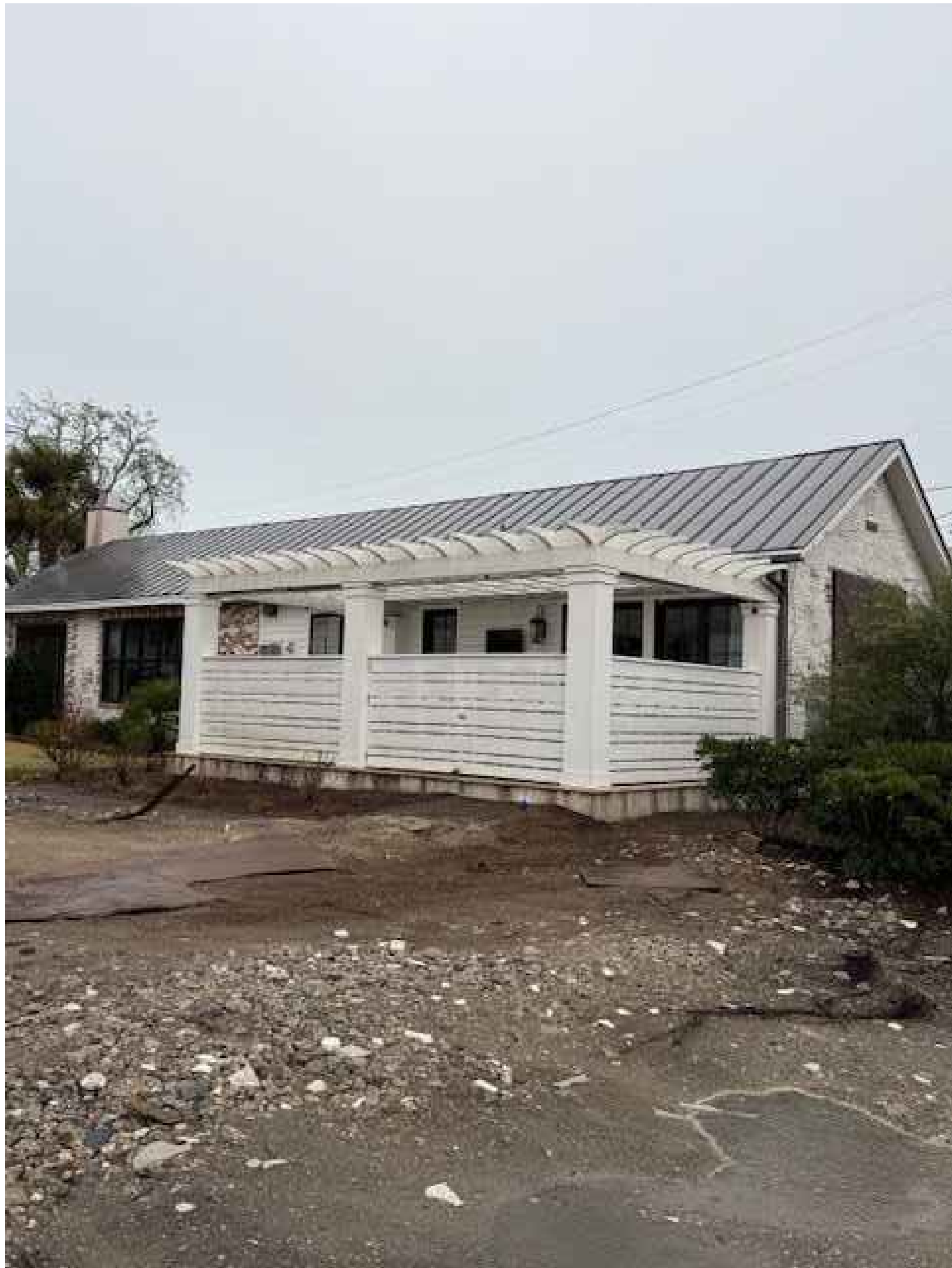
IMAGE OF EXISTING PERGOLA
