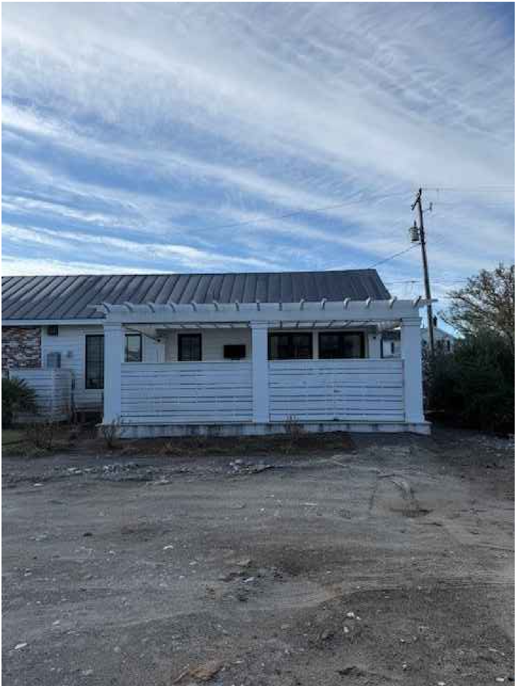
IMAGE OF EXISTING PERGOLA
