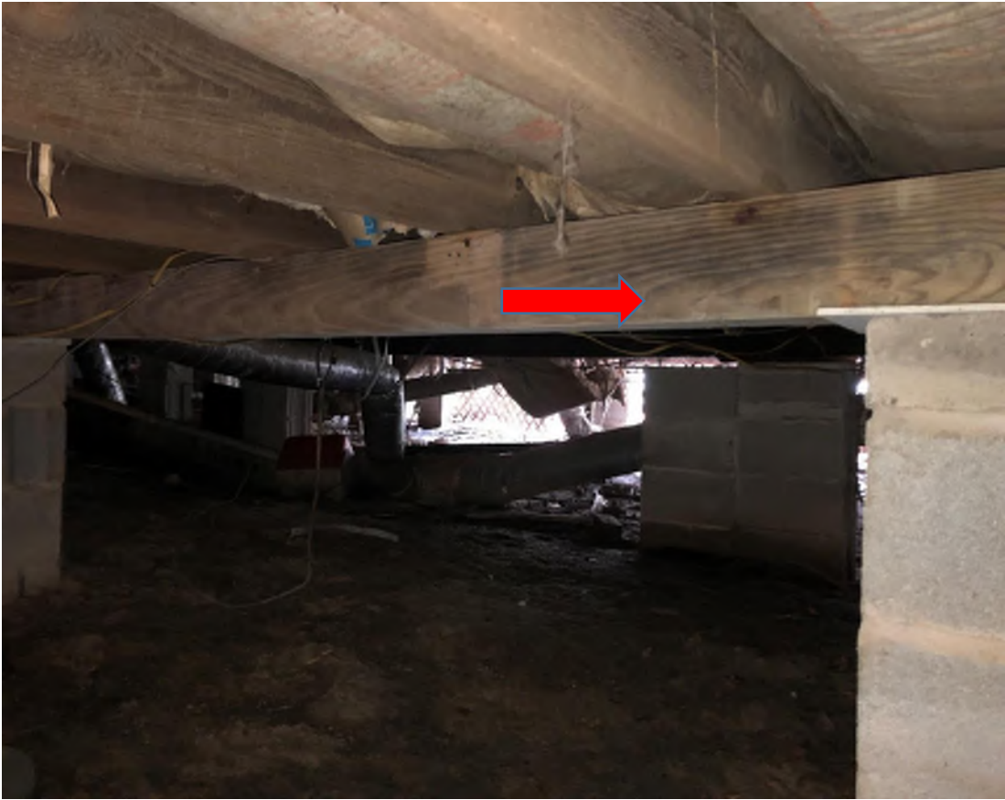
Fig. 1-9. Timber girder appears to be in good condition.
