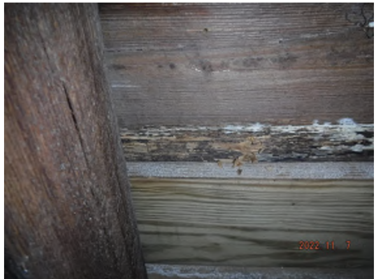
Rot/moisture damage to siding.
