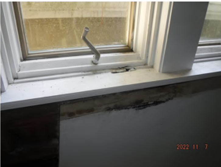
Rot/moisture damage to window.
