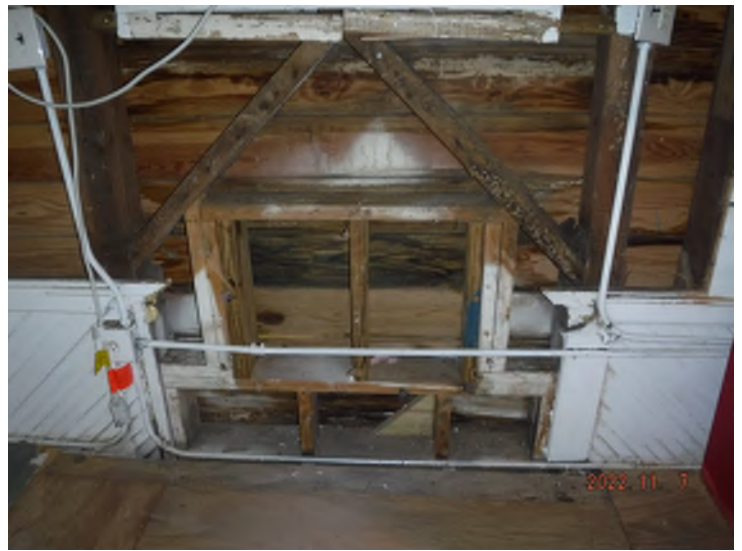
Rot/moisture damage.
