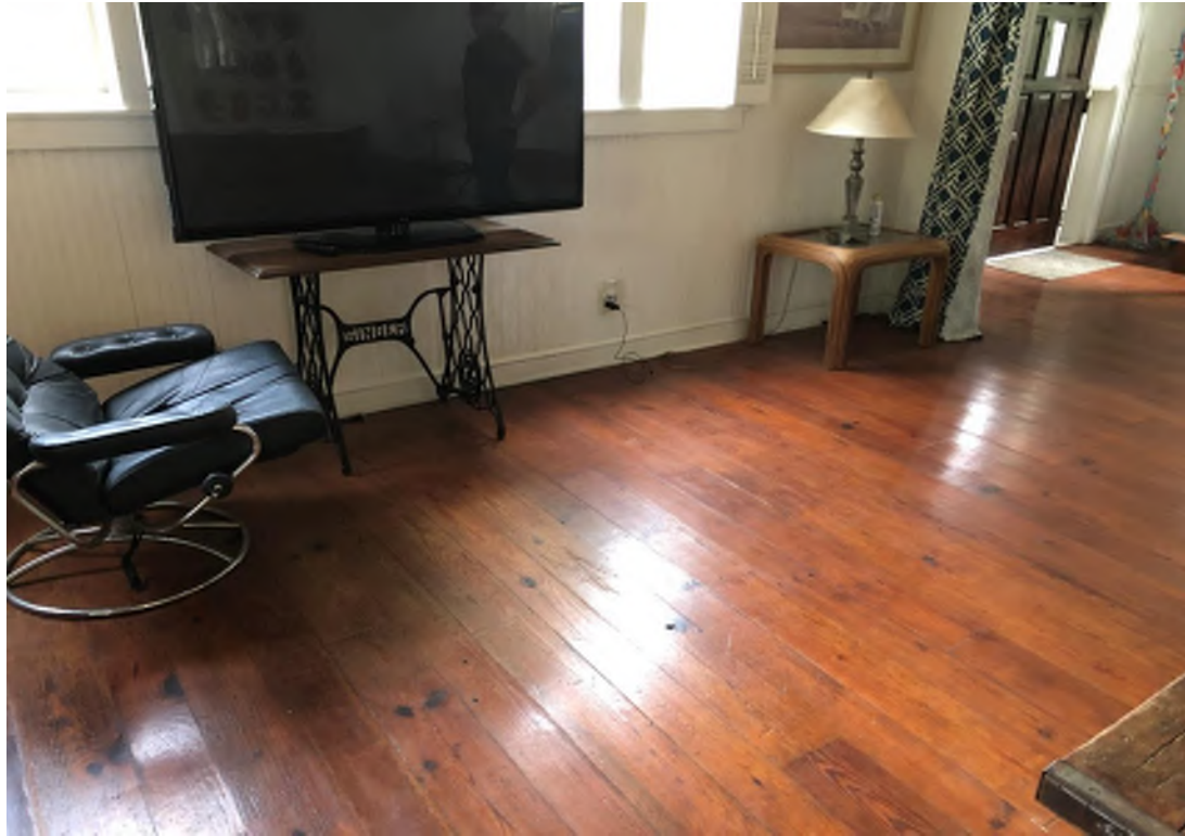
Fig. 1-11. 1 st floor floors are sloping due to unevenness of CMU piers below.
