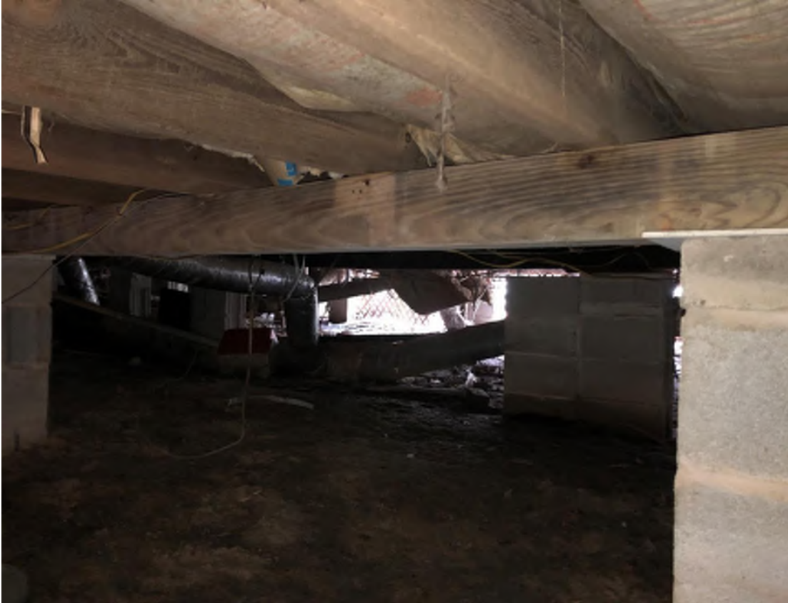
Fig. 1-6. Soil is not level in the crawlspace. Also, there is no vapor barrier present.
