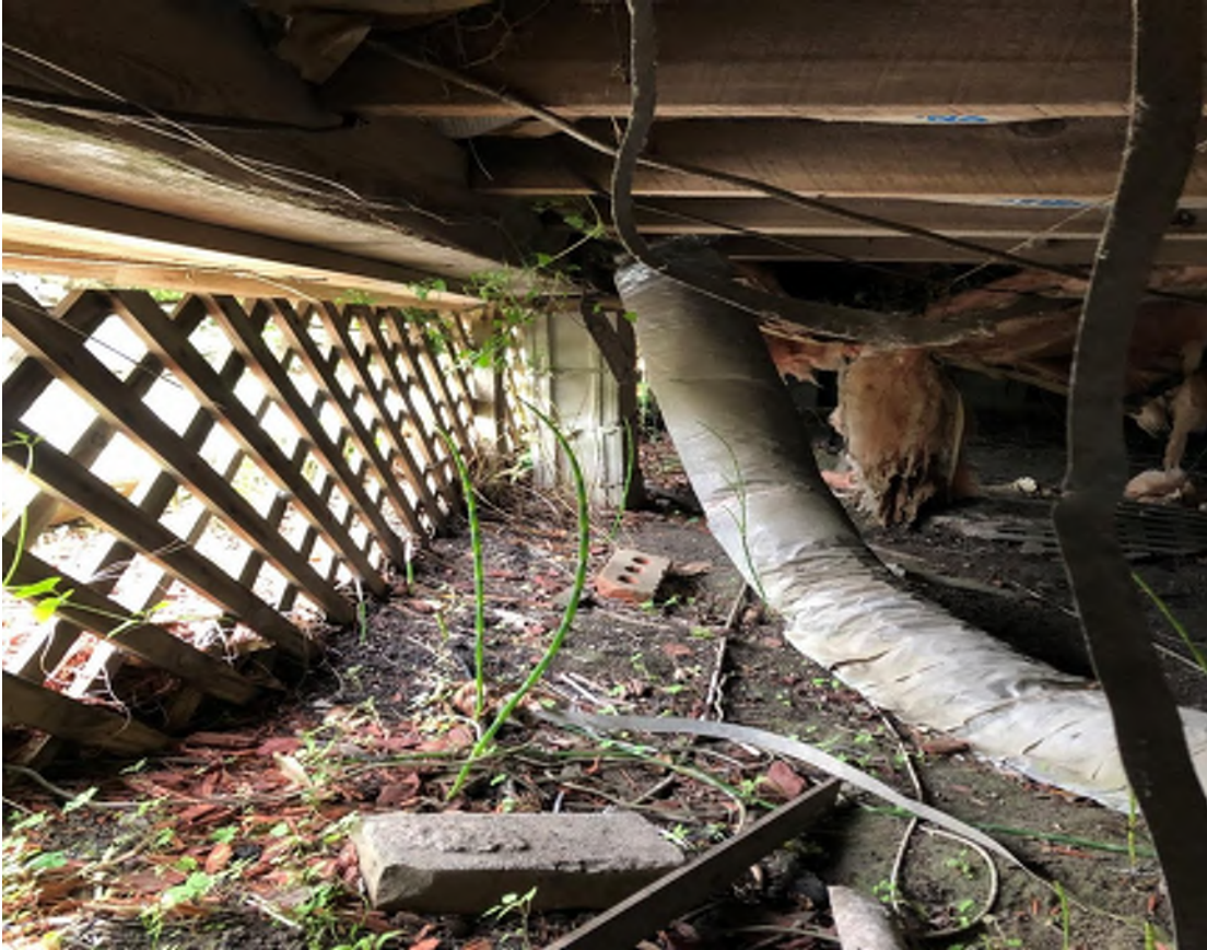
Fig. 1-8. Timber girder appears to be in good condition.
