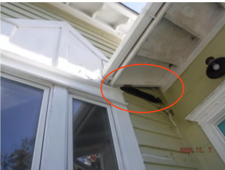
It appears to be rot/moisture damage
