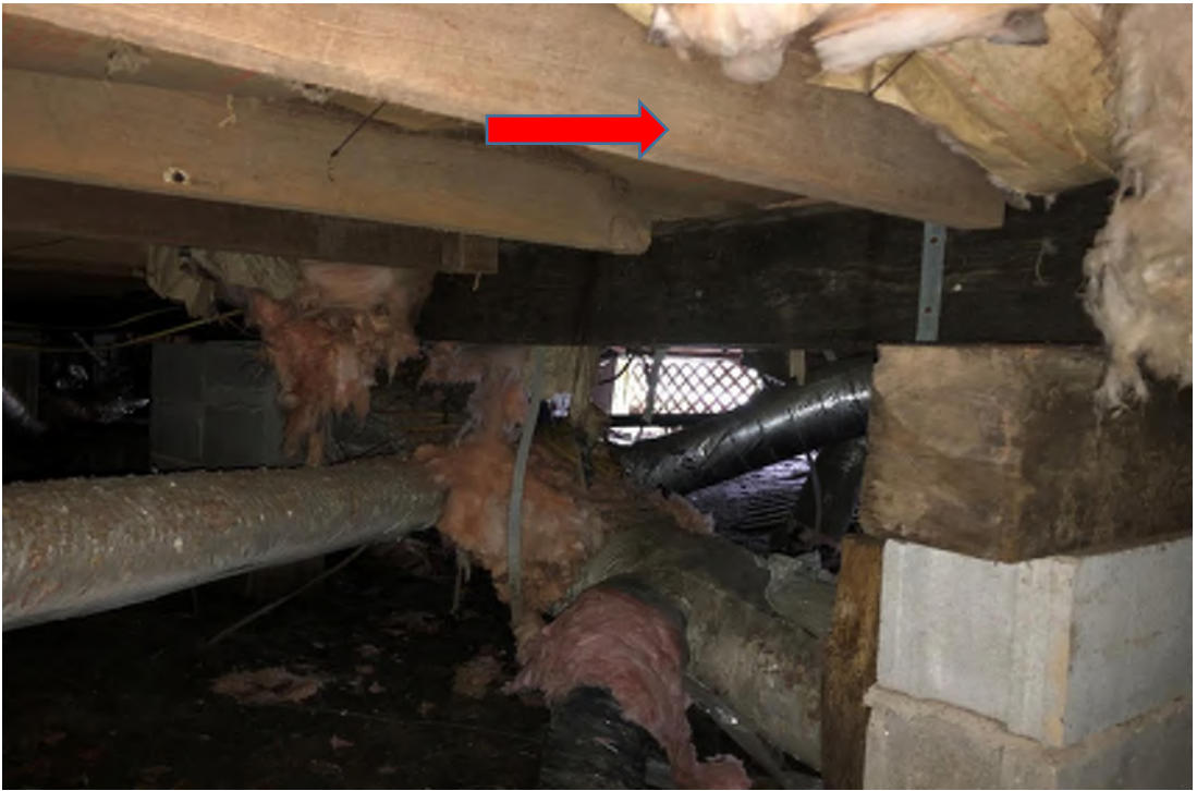
Fig. 1-10. Floor joists appear to be in good condition.
