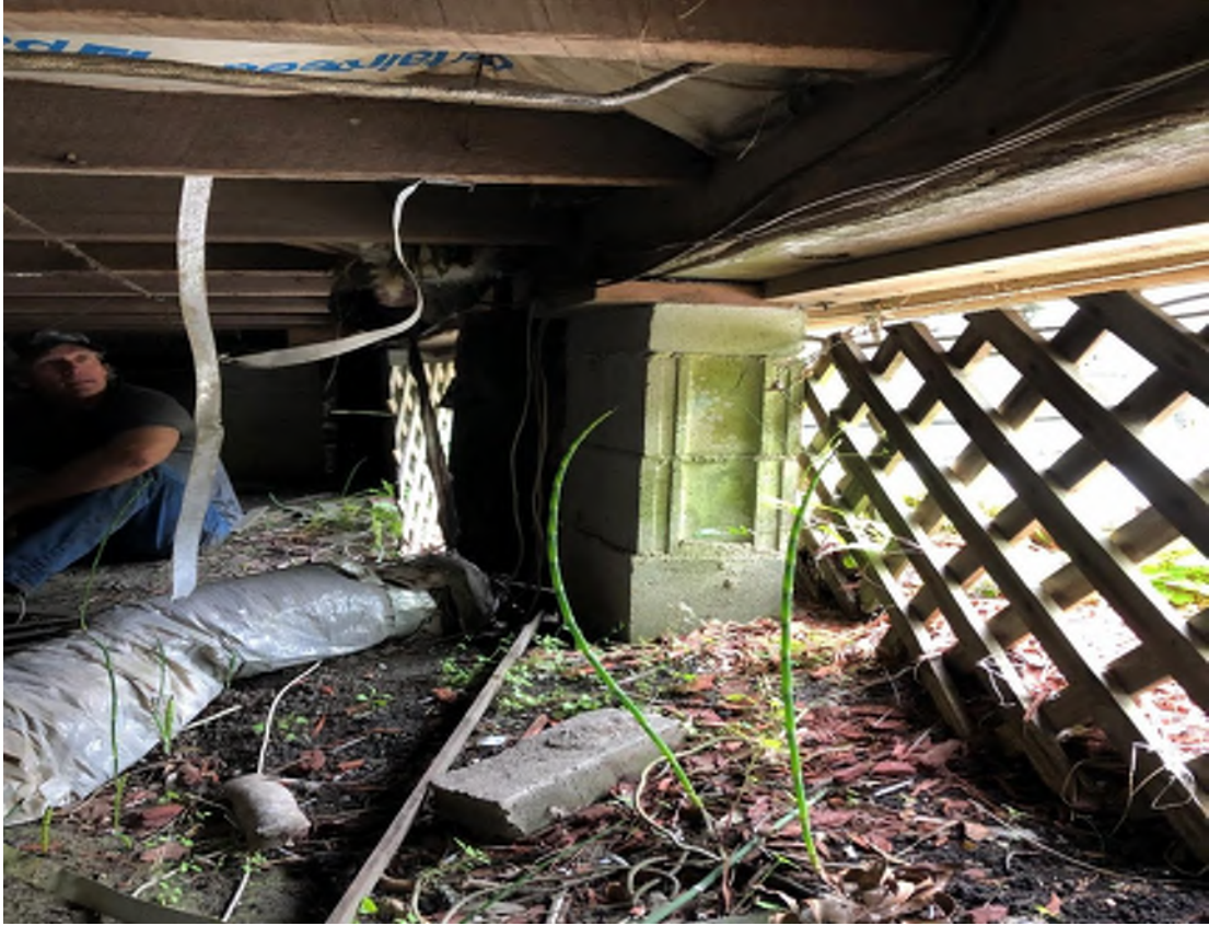
Fig. 1-4. Overturned CMU pier, near front of house, with thin rectangular footing attached to pier.
