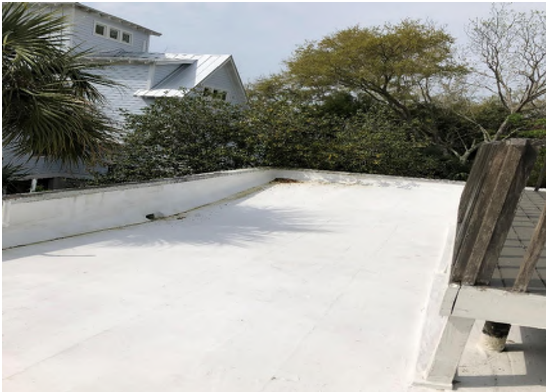
Fig. 1-20. The rear apartment has a commercial style roof, likely a EPDM (Ethylene Propylene Diene Terpolymer) roof.
