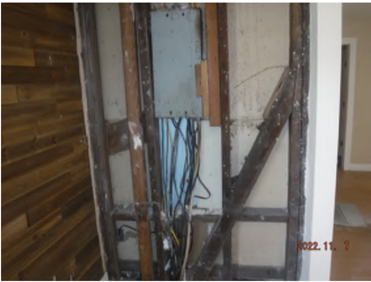
Rot/moisture damage.
