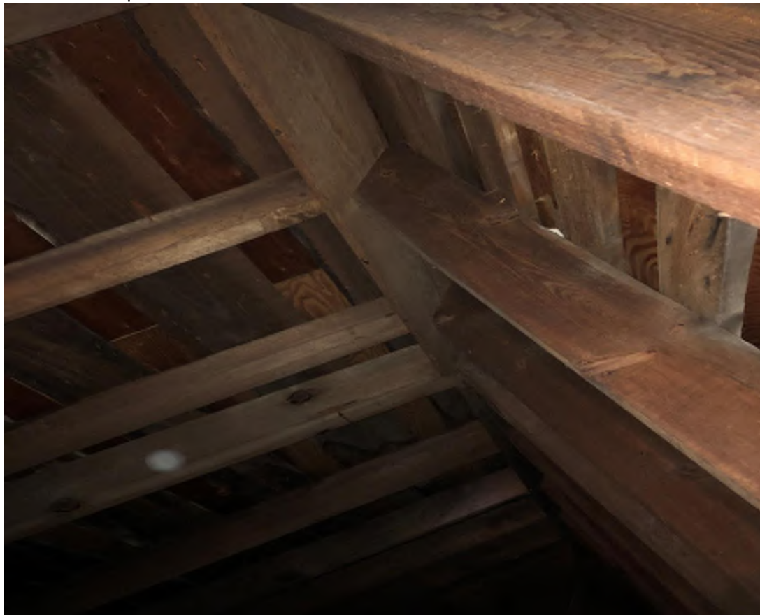
Fig. 1-16. Timber roof rafters and ridge board appear to be in satisfactory condition. However, ridge board is inadequate in size and not continuous.
