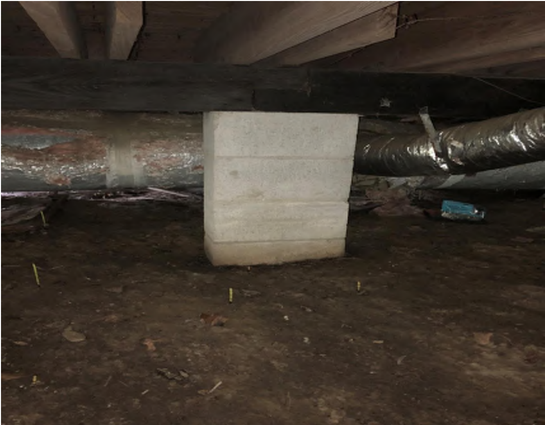
Fig. 1-8. Timber girder appears to be in good condition.
