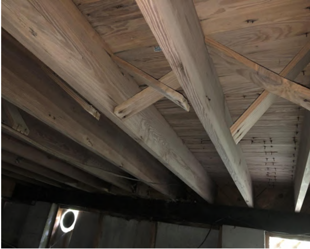
Fig. 1-19. The floor joists blocking are dislodged (under rear apartment).
