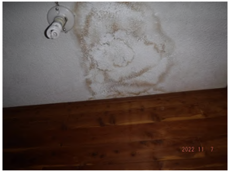
Moisture stains on ceiling
