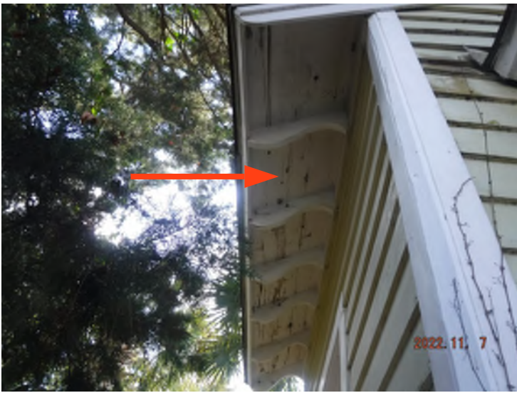
Rot/moisture damage to overhang.
