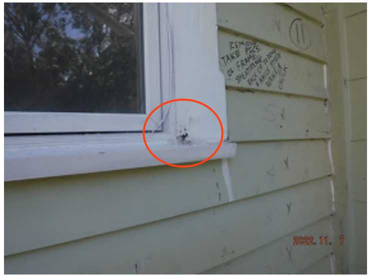
Rot/moisture damage to window trim.
