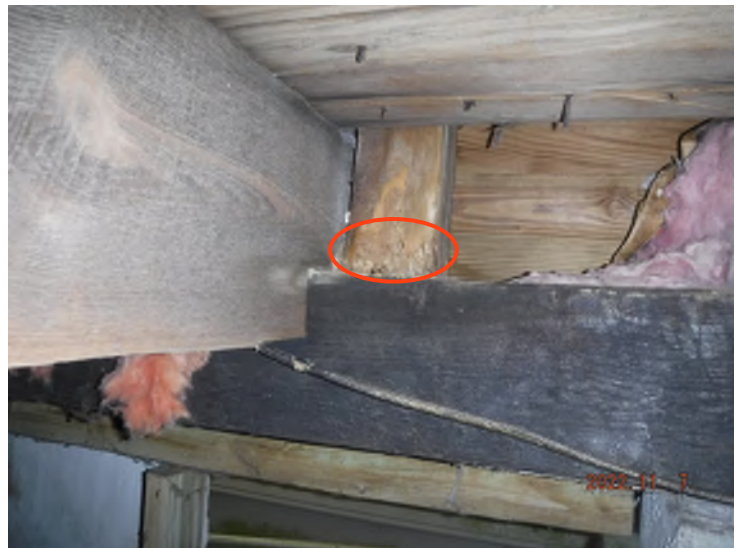
Previous subterranean termite and powder post beetle activity and damage in the crawlspace.
