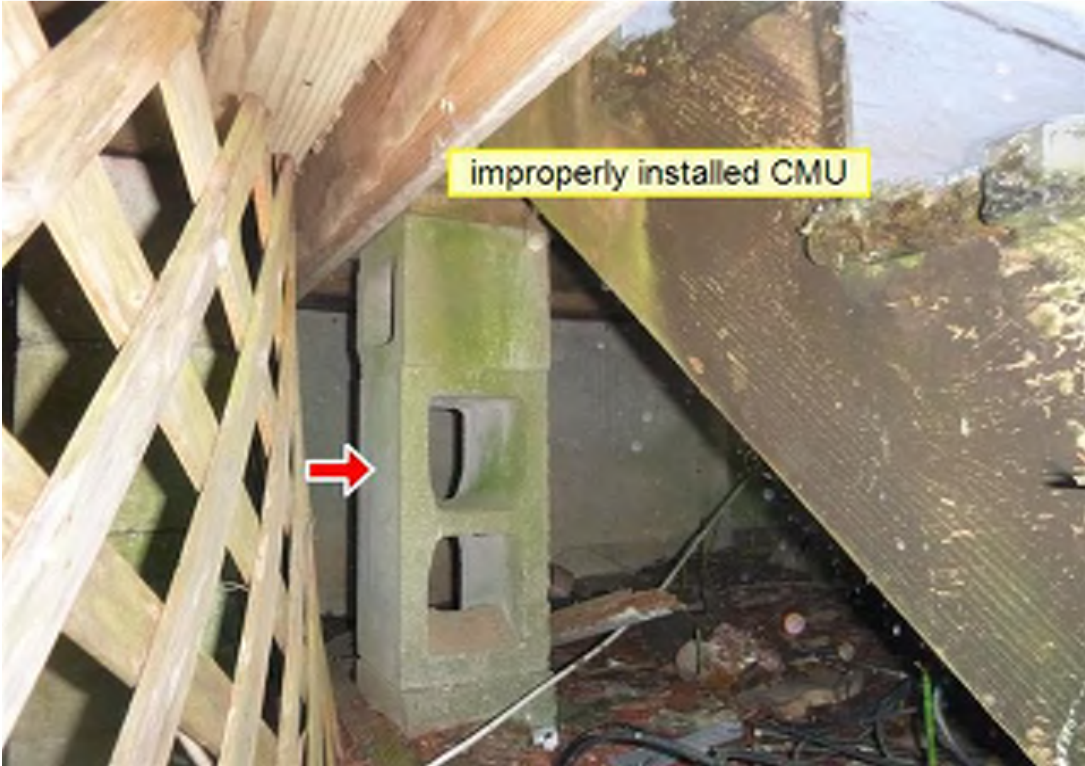
Fig. 1-18. Pier is improperly built and should be replaced.
