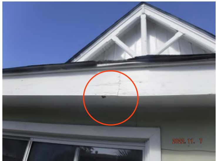
Rot/moisture damage to fascia.
