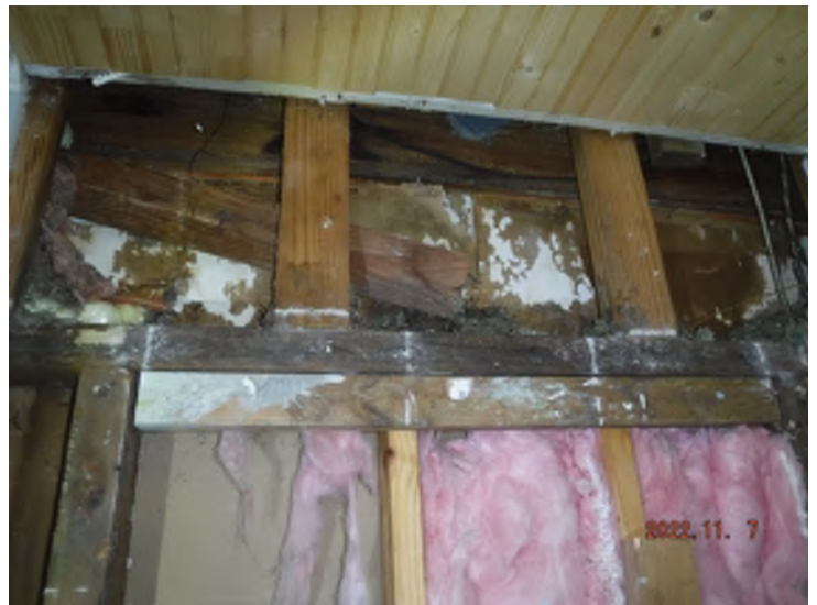
Rot/moisture damage.
