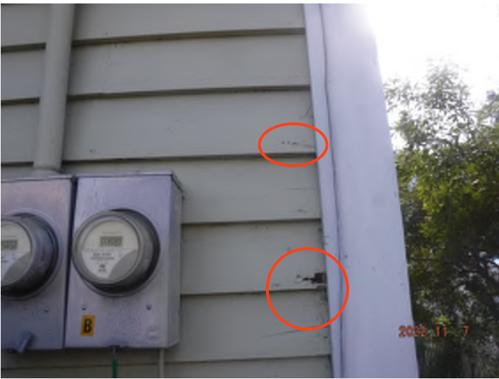
Rot/moisture damage and previous subterranean termite activity damage to siding.
