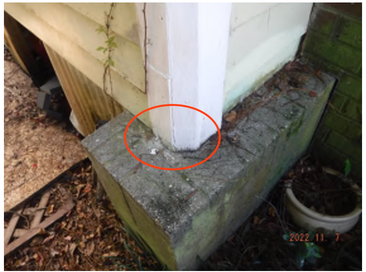
Rot/moisture damage to trim.
