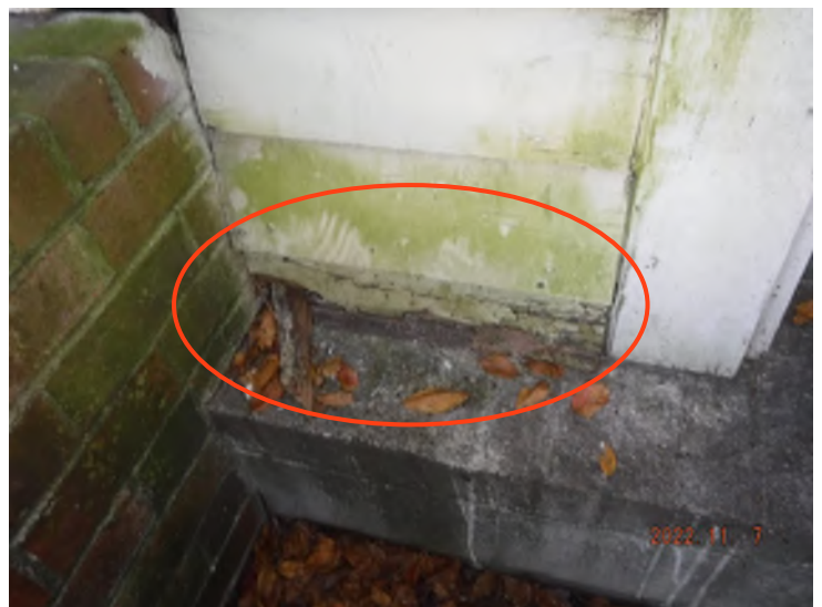
Rot/moisture damage to siding.
