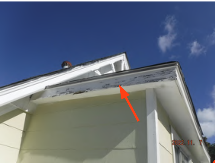
Rot/moisture damage to fascia.
