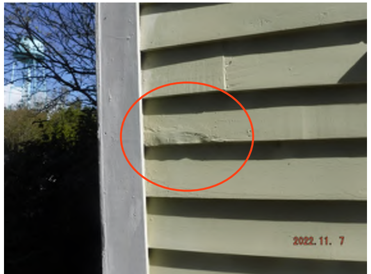
Rot/moisture damage to siding.
