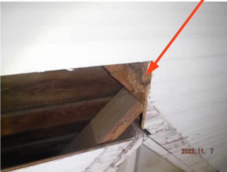
Rot/moisture damage to fascia.
