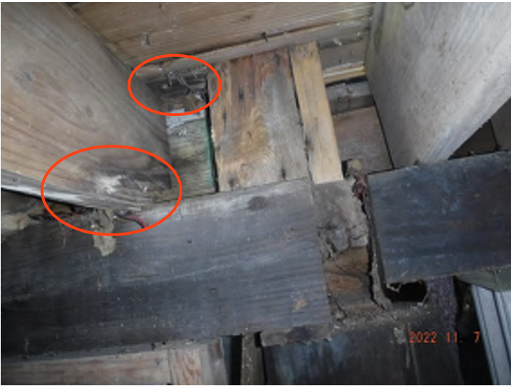
Rot/moisture damage
