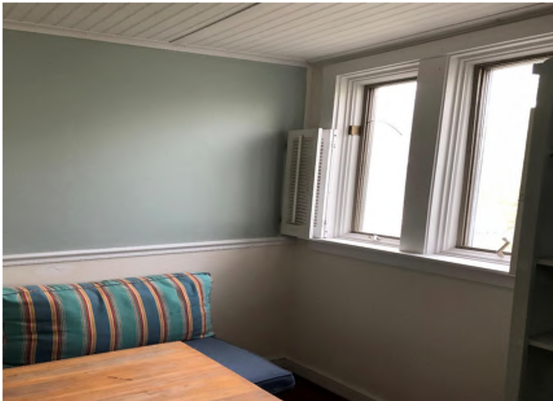
Fig. 1-12. Wall in kitchen is leaning outwardly, due CMU piers rotation underneath in crawlspace.
