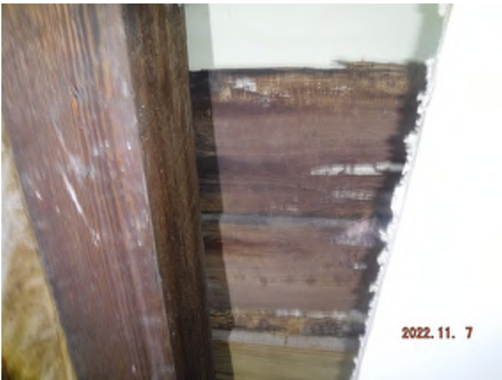
Rot/moisture damage to siding.
