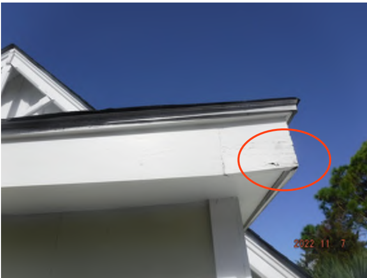
Rot/moisture damage to fascia.
