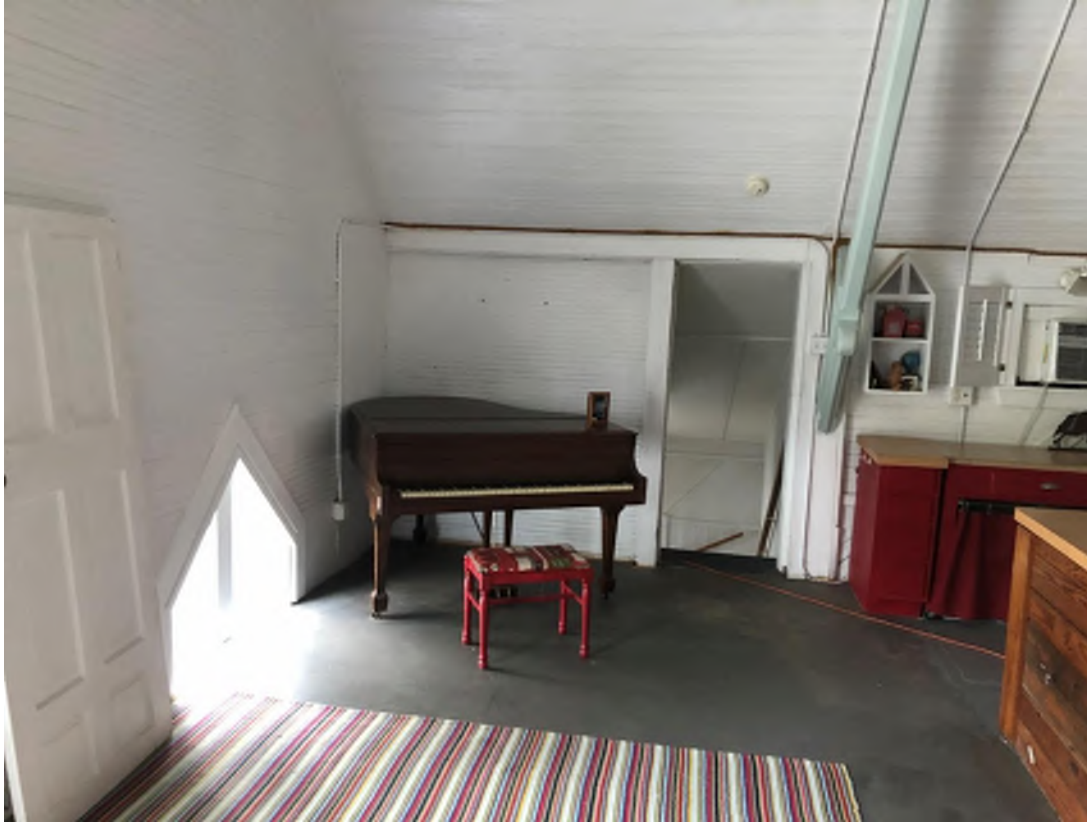
Fig. 1-15. 2 nd floor sloping from bottom left (area w/ carpet) down towards the piano.
