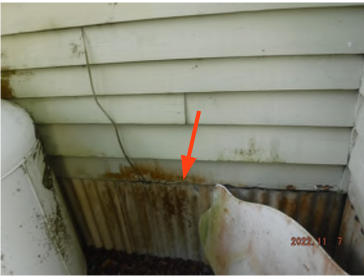
Rot/moisture damage to siding.
