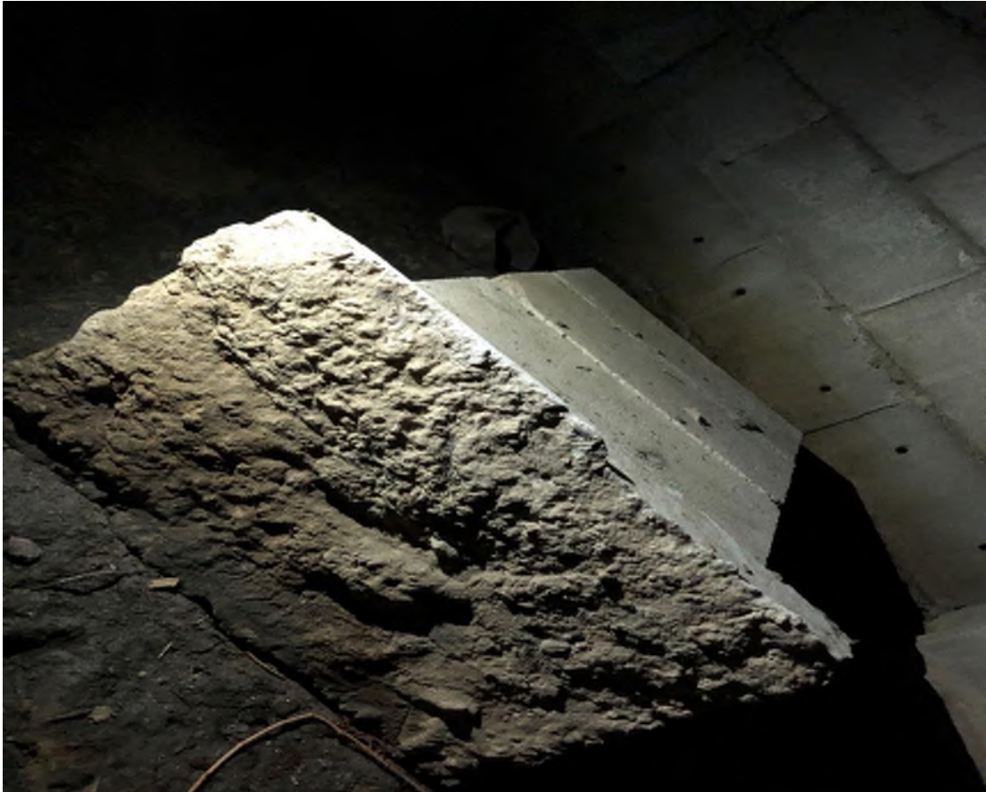
Fig. 1-4. Overturned CMU pier, near front of house, with thin rectangular footing attached to pier.
