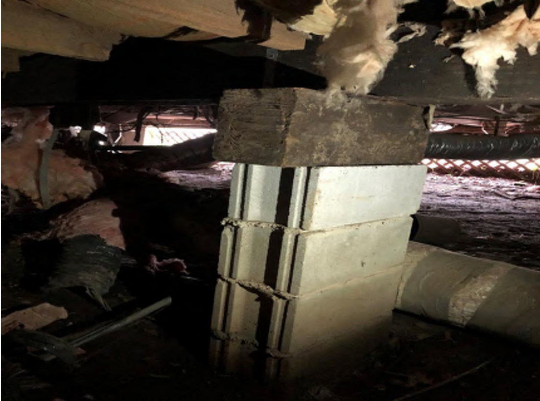
Fig. 1-6. Soil is not level in the crawlspace. Also, there is no vapor barrier present.
