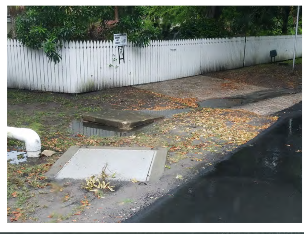
APRIL 2017, ATLANTIC AVENUE & STATION 18 ST INTERSECTION DURING AN APPROXIMATE 4.0-INCH RAIN EVENT (2-YEAR STORM EVENT IN CHARLESTON COUNTY ESTIMATED 4.6-INCH IN 24 HOUR)
