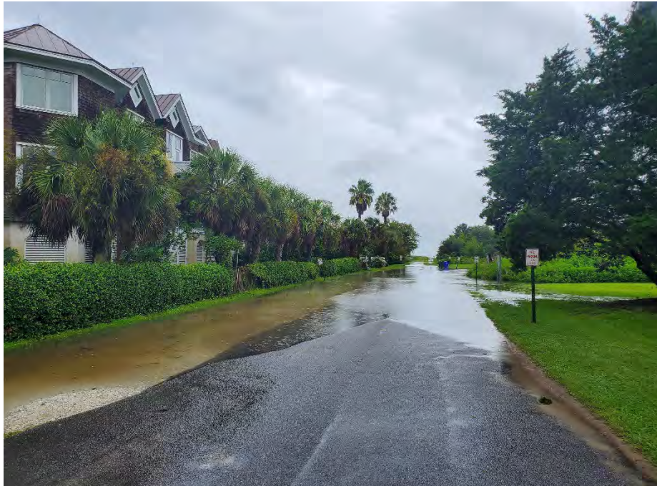
Lite rainfall – standing water due to no outlet.
