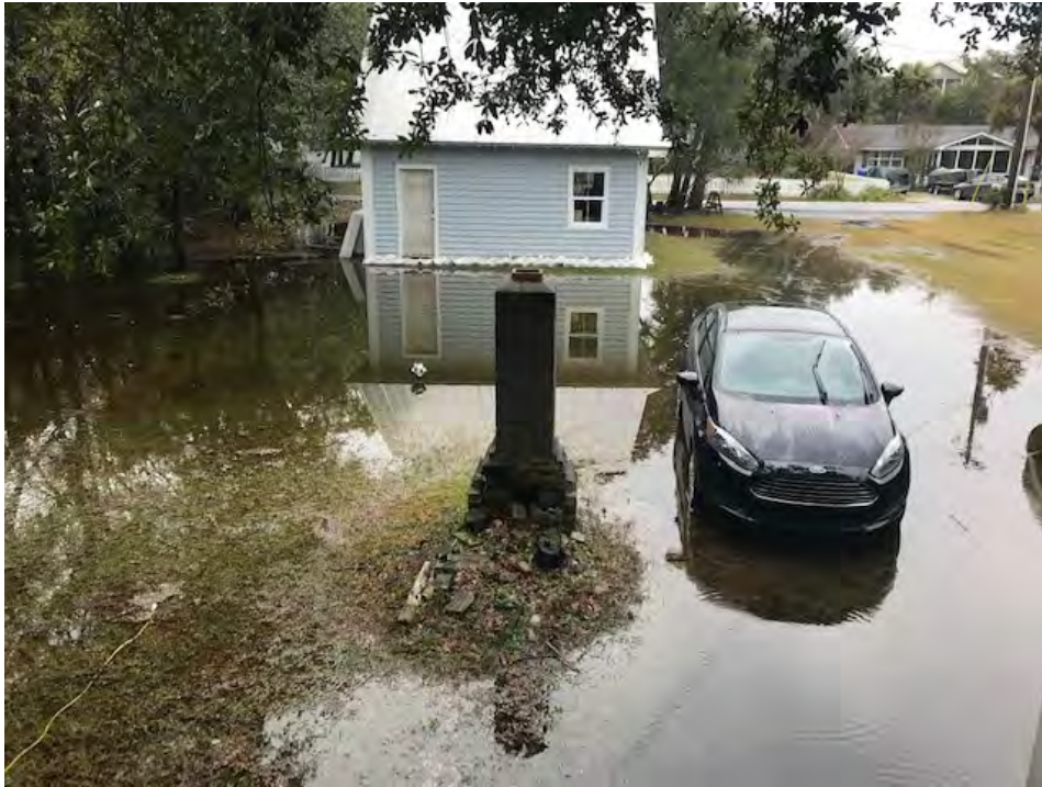
Flooding from short rainfall uphill from proposed pump station site at Sta 18.
