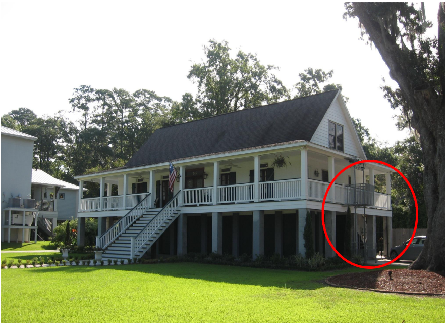
For high increase elevation buildings, chair lifts should be placed on rear or side elevations where they are less visible. This design has minimal structural framework and the porch can be viewed behind it.
