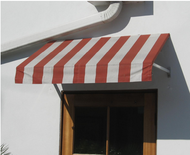
This entrance at the commercial building at 2019 Middle Street displays an appropriate canvas awning.
