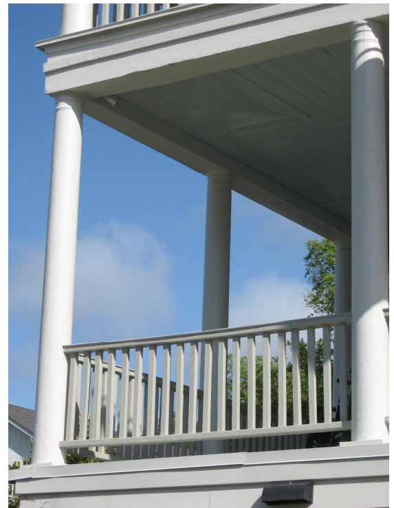
By the early twentieth century, porch columns were often designed in classical styles including Tuscan, as at 1808 Middle Street.
