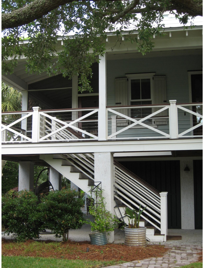
The porch on the elevated dwelling at 1856 Central Street has appropriate porch column and foundation pier alignments and railing.
