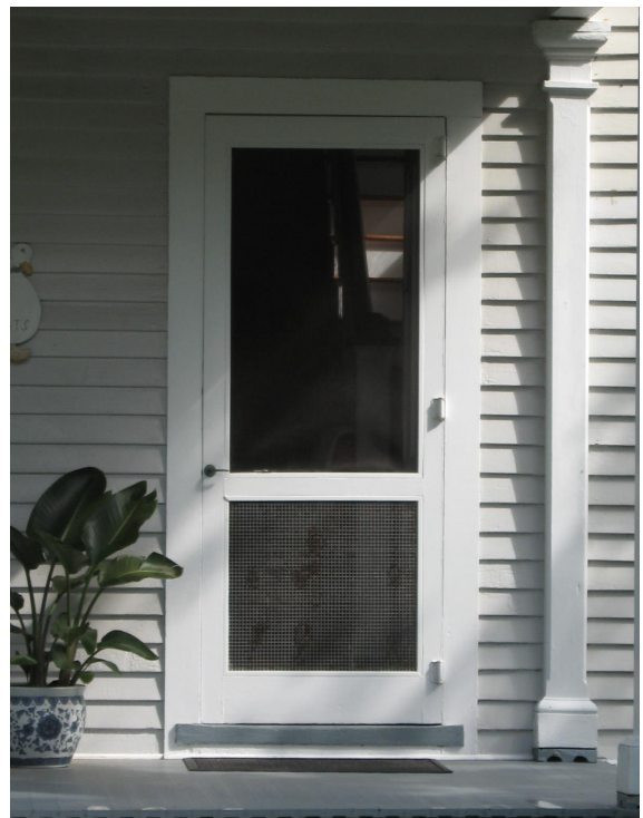
Preserve original or appropriate design screen doors (1748 Central Street).
