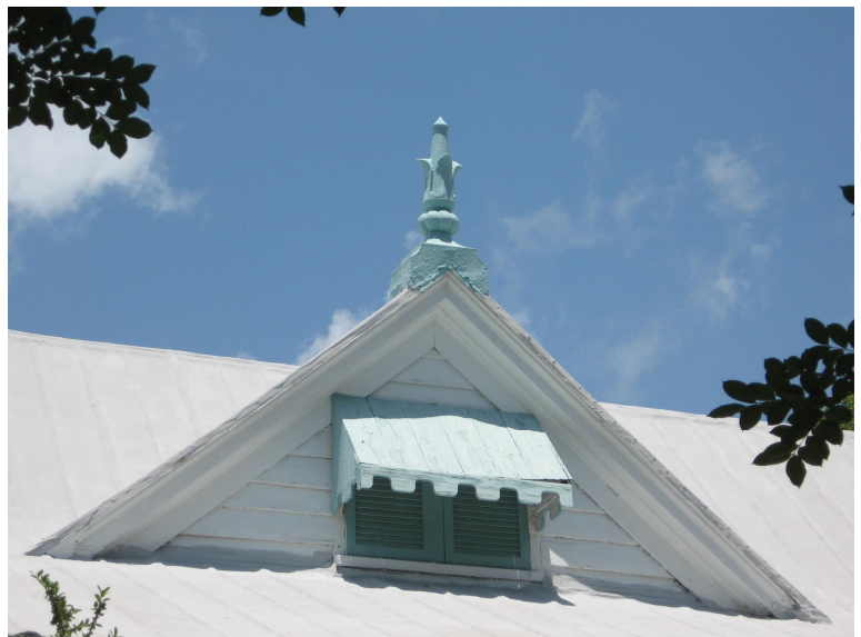
A distinctive wood finial is a distinguishing detail at the roofline of 2662 Middle Street.
