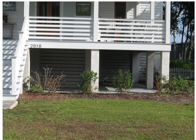
These stuccoed concrete piers are appropriate for the dwelling and are aligned with the porch columns above (2018 Middle Street).
