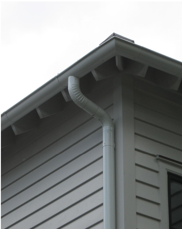
Gutters are recommended to be half-round design with round downspouts, (924 Middle Street, left and 2612 Jasper Street, right).
