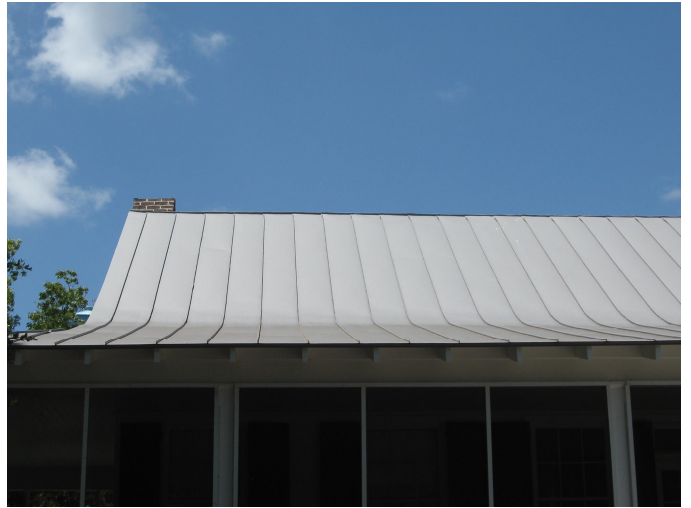
YES - Examples of appropriate metal roofs include the crimped design at 1908 I'on Avenue (left) and the metal standing seam roof at 2430 I'on Avenue (right).
