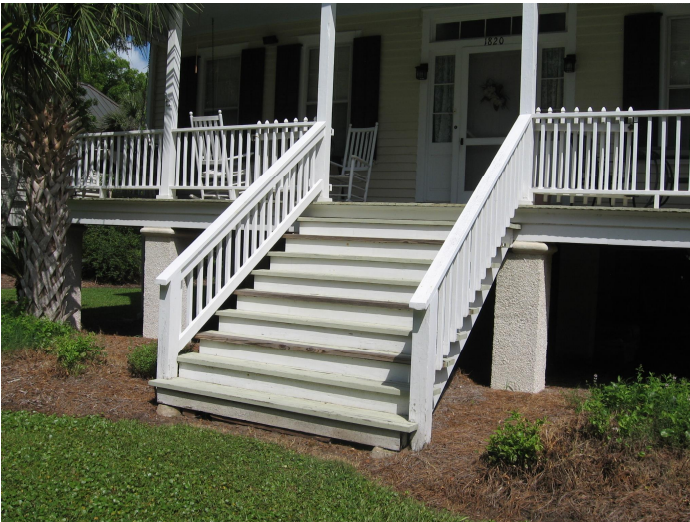
Illustration of a straight-run staircase for a low increase building elevation project (1820 Central Street).
