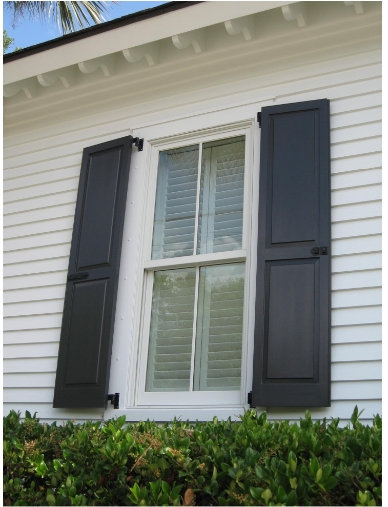
The two-over-two sash window at 1514 Middle Street is an example of an appropriate aluminum clad wood sash window.
