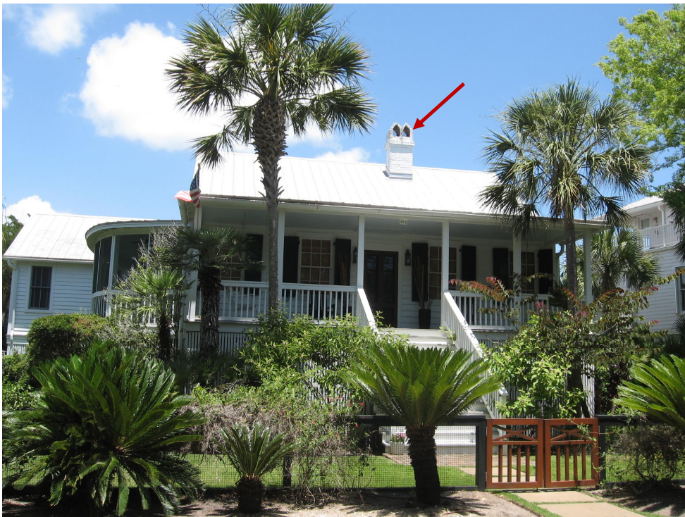
Elevation projects should have the chimneys preserved and elevated with the dwelling as at 950 Middle Street.
