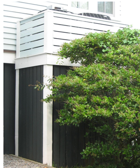
These elevated mechanical units are screened with lattice panels (left, 1744 I'on Avenue) and horizontal slats, (right, 1856 Central Street).
