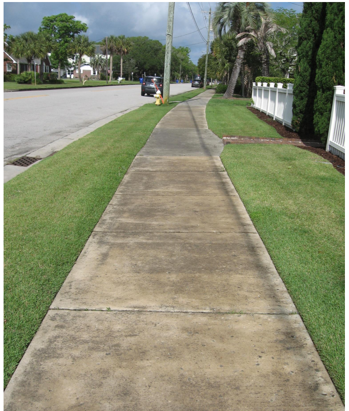
Concrete sidewalks added in the early- to -mid-20th century should be preserved and maintained as in the 1700 block of Middle Street.
