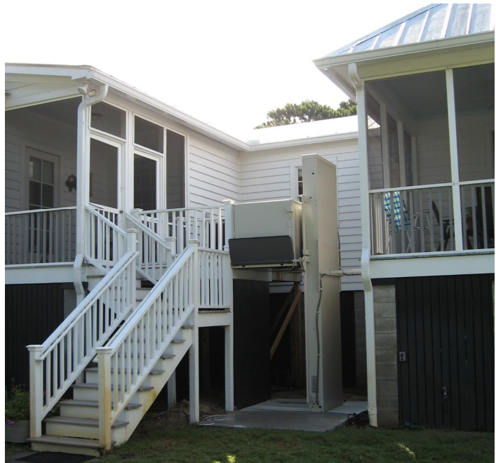
This chair lift at 2602 Jasper Street is appropriately sited at the rear elevation and recessed within the two wings to reduce visibility.
