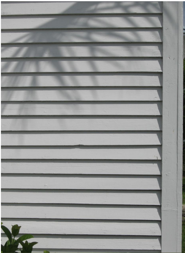
At left is the weatherboard siding at 1754 Central Street which contrasts with the novelty (or drop) siding which has tongue-in-groove boards with concave curves as at 1902 I'on Avenue at right.
