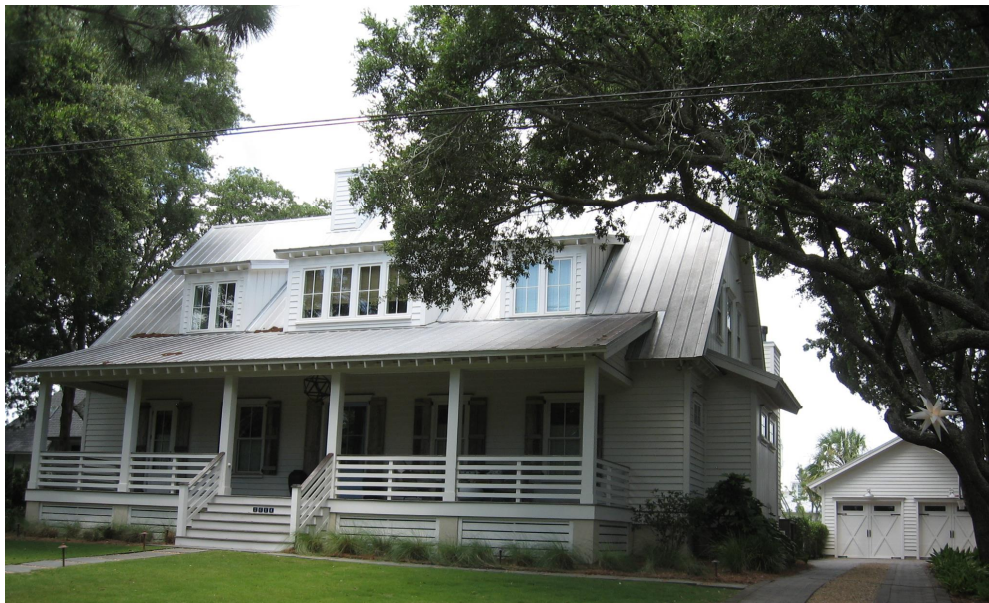
Built in 2015, the dwelling at 2614 Gold Bug Avenue was designed in a traditional gabled ell plan with appropriate scale, materials and orientation to the street.
