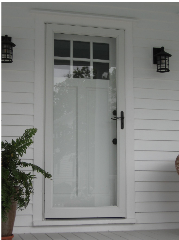
YES- Storm doors should be unobtrusive and blend with the historic door as in this example.
