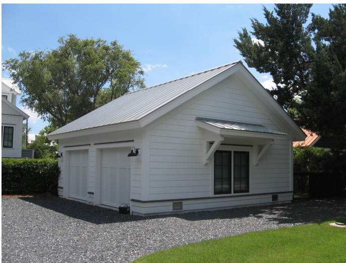
YES: This new garage is appropriately scaled, and its garage door is based on traditional designs. Flood vents were also added to this building ( 2408 Myrtle Street).
