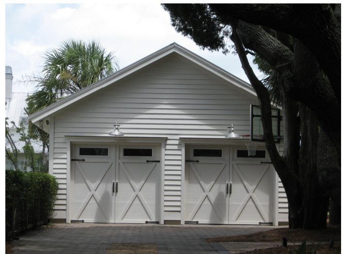
YES: This new garage features a gable front design and has appropriate glass and wood garage doors (2614 Gold Bug Avenue).
