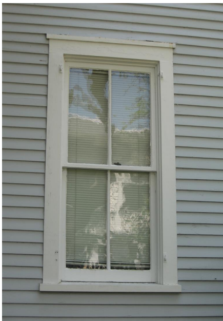
By the late nineteenth century, two-over-two wood sash windows were widely used in Sullivan's Island (1744 I'on Avenue).
