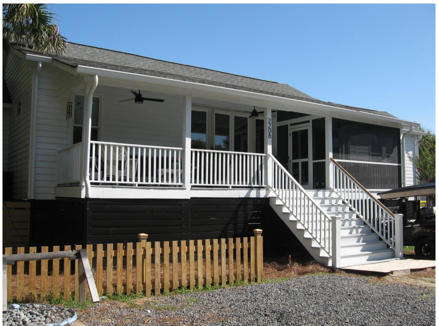
Screening of front porches is discouraged but may be appropriate if minimal structural framing is used, and only one bay of the porch is enclosed as at 2602 Jasper Street (above) and 2208 I'on Avenue (right).
