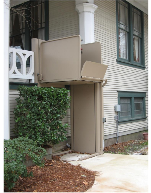
ADA compliance can be achieved for low elevation buildings through adding chair lifts. This example shows an ADA-compliant parking space and a lift screened with landscaping. Only a small section of this porch railing was removed and can be reinstated when the lift is no longer in use.
