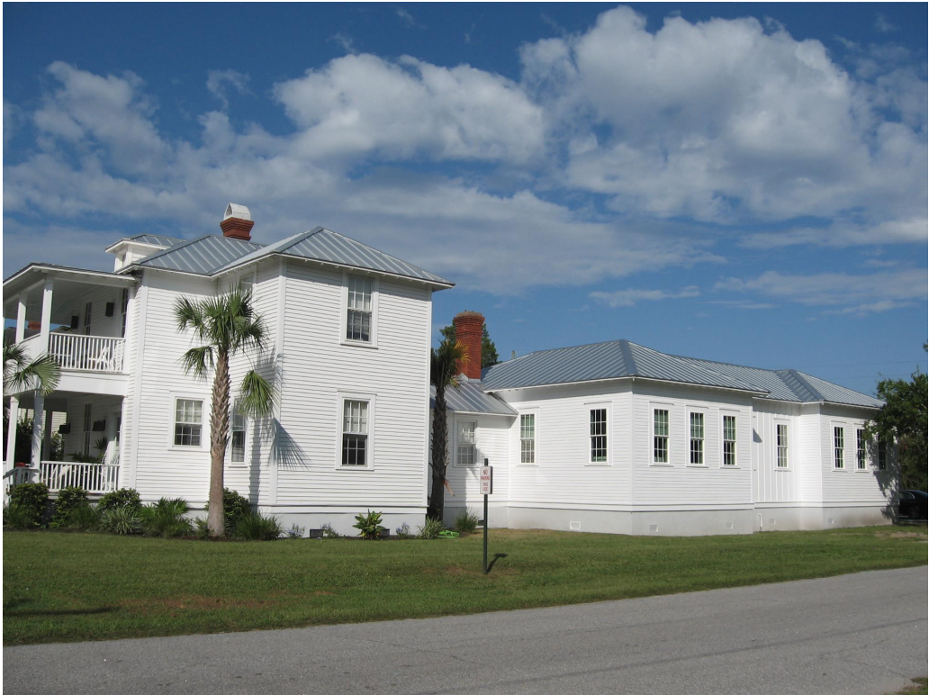
The dwelling at 1754 Central Street was designed with a large rear addition connected by a recessed hyphen.
