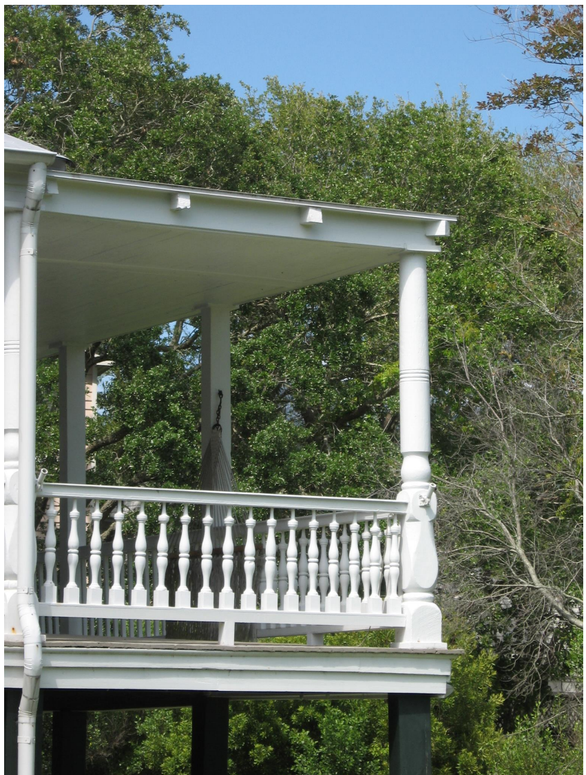
Milled wood porch columns and turned balusters on the porch railings are one of the most important defining features of a dwelling's style (1112 Osceola Avenue).
