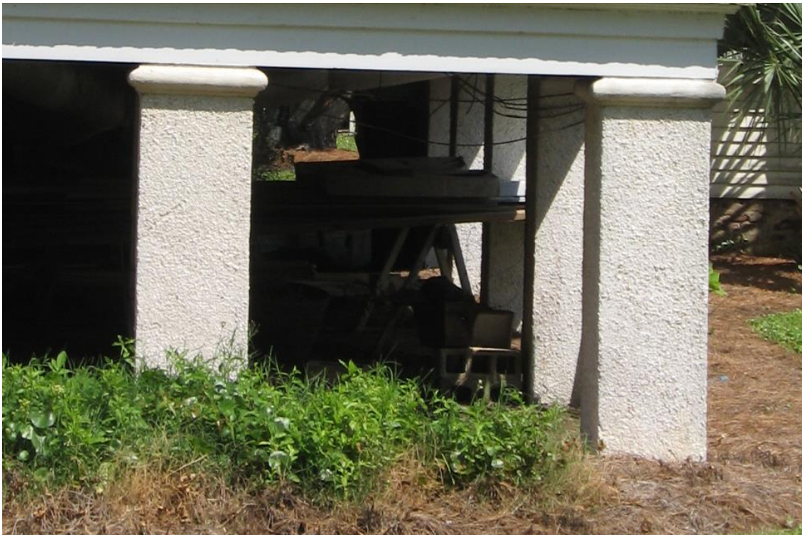
Foundation piers for dwellings are often of concrete and stucco materials such as at 1820 Middle Street.
