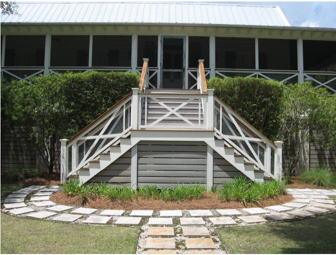
Example of a center/linear split staircase for a high increase building elevation project (2408 I'on Avenue).
