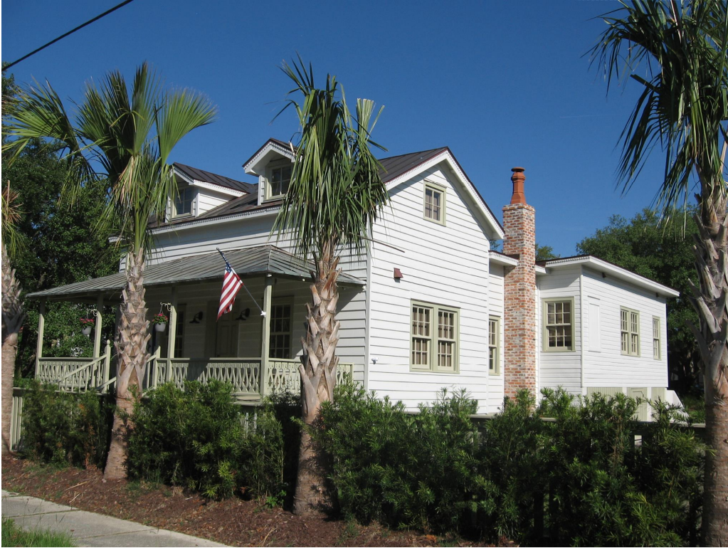
The dwelling at 2630 Middle Street has a rear addition which is inset from the footprint of the original dwelling (above) and has appropriate materials and details (below).
