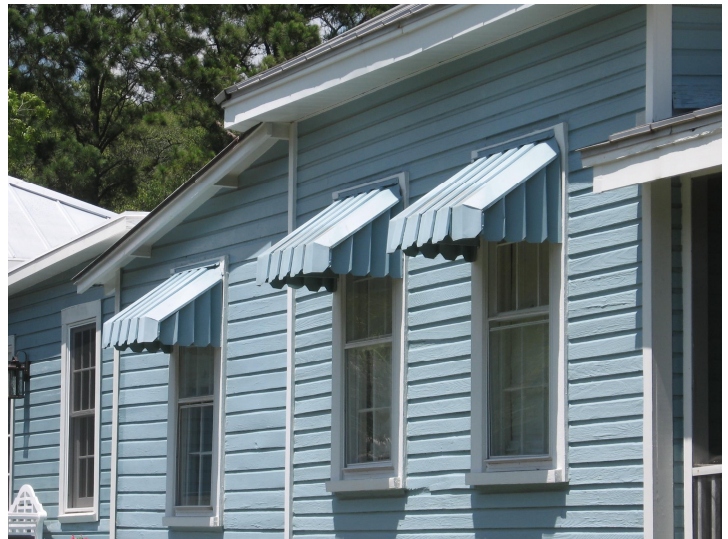
Appropriate metal awnings at 2614 Myrtle Street.
