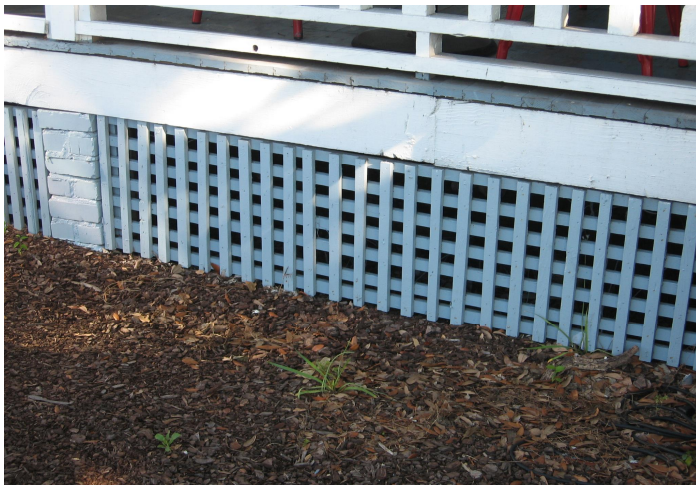
Lattice panels are appropriate treatments for screening between brick piers (2120 Middle Street).
