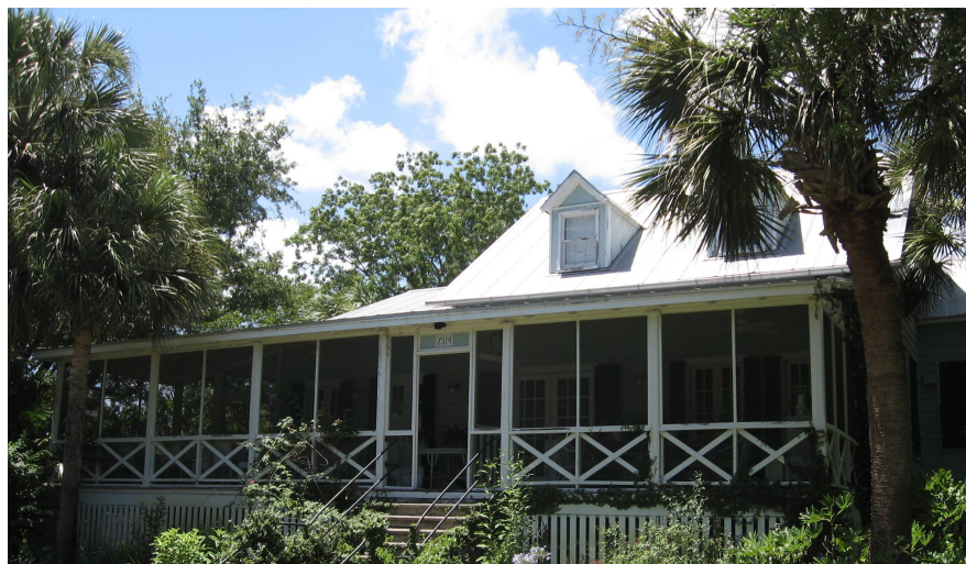
Another common typology is a one and one-half story cottage with an "L" shaped porch, (2504 Iron Avenue).
