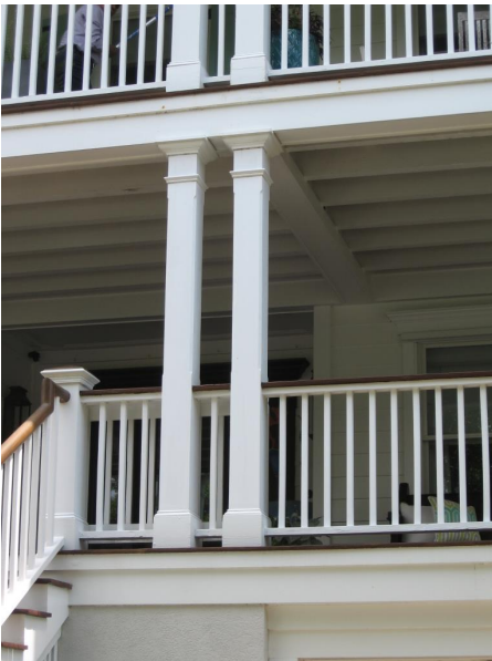
The porch at 1002 Middle Street displays Doric-motif porch columns.
