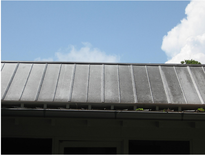
YES - Examples of appropriate metal roofs include the crimped design at 1908 I'on Avenue (left) and the metal standing seam roof at 2430 I'on Avenue (right).
