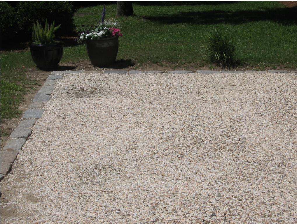
Driveways should be of permeable paving materials to allow for water absorption. At left is a driveway composed largely of gravel at 2061 Pettigrew Street. At right is a driveway at 2614 Myrtle Street of interlocking concrete pavers which helps to decrease water runoff.
