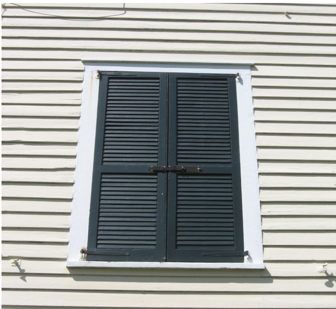
When closed, shutters should cover the window opening to which they are attached (1820 Central Street).
