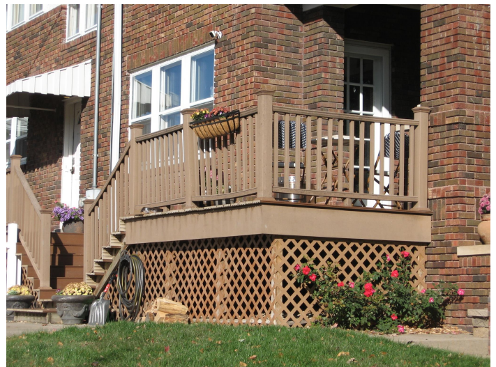
YES: This deck is appropriately sited at the rear entrance, has square balusters and lattice panels to enclose the foundation.
